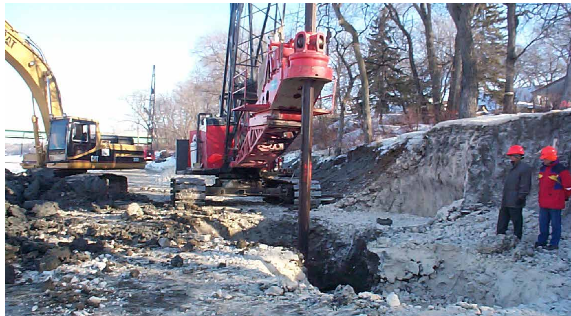
1 DRILLING ROCKFILL COLUMNS Large diameter holes are drilled into the bank through the weak clay and into deeper, stronger soil known as "till".
