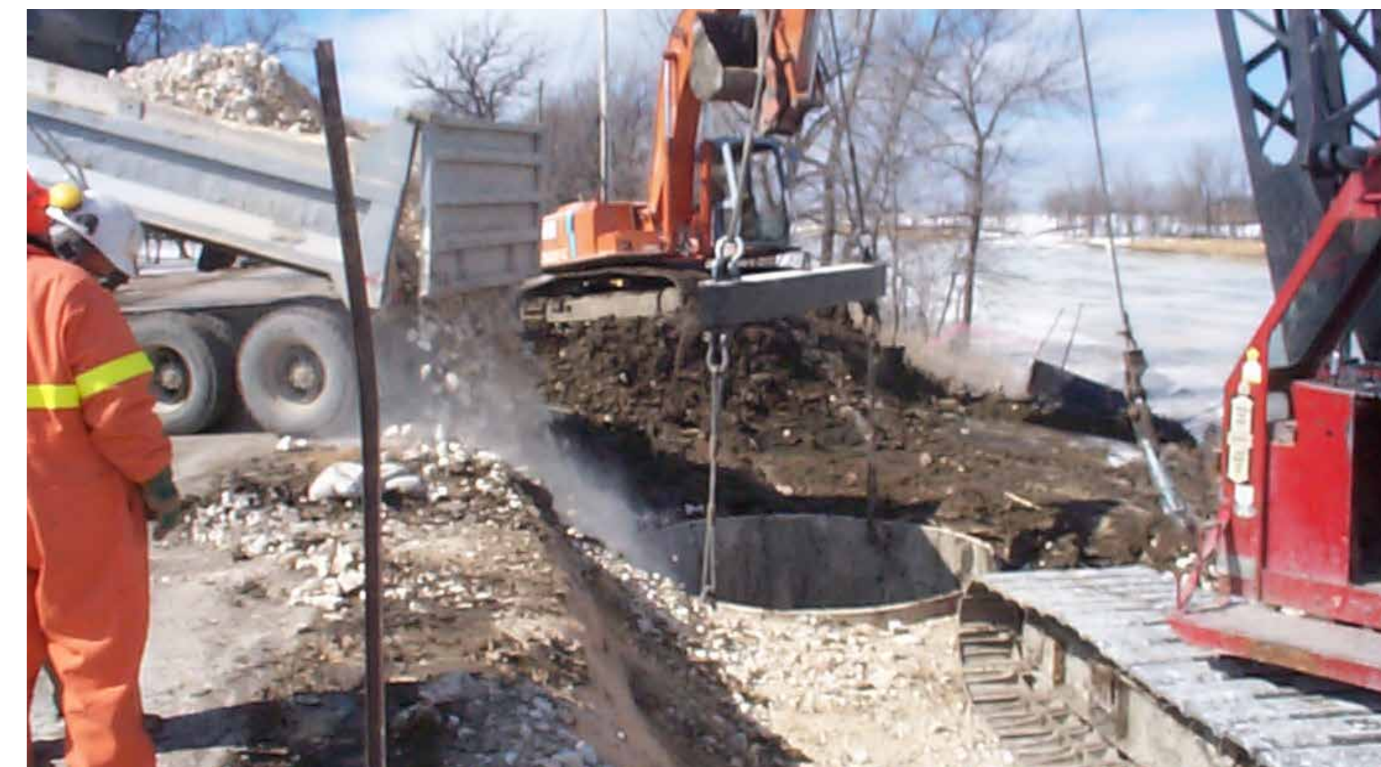
2 FILLING ROCKFILL COLUMNS The holes are backfilled with stronger materials (crushed rockfill).
