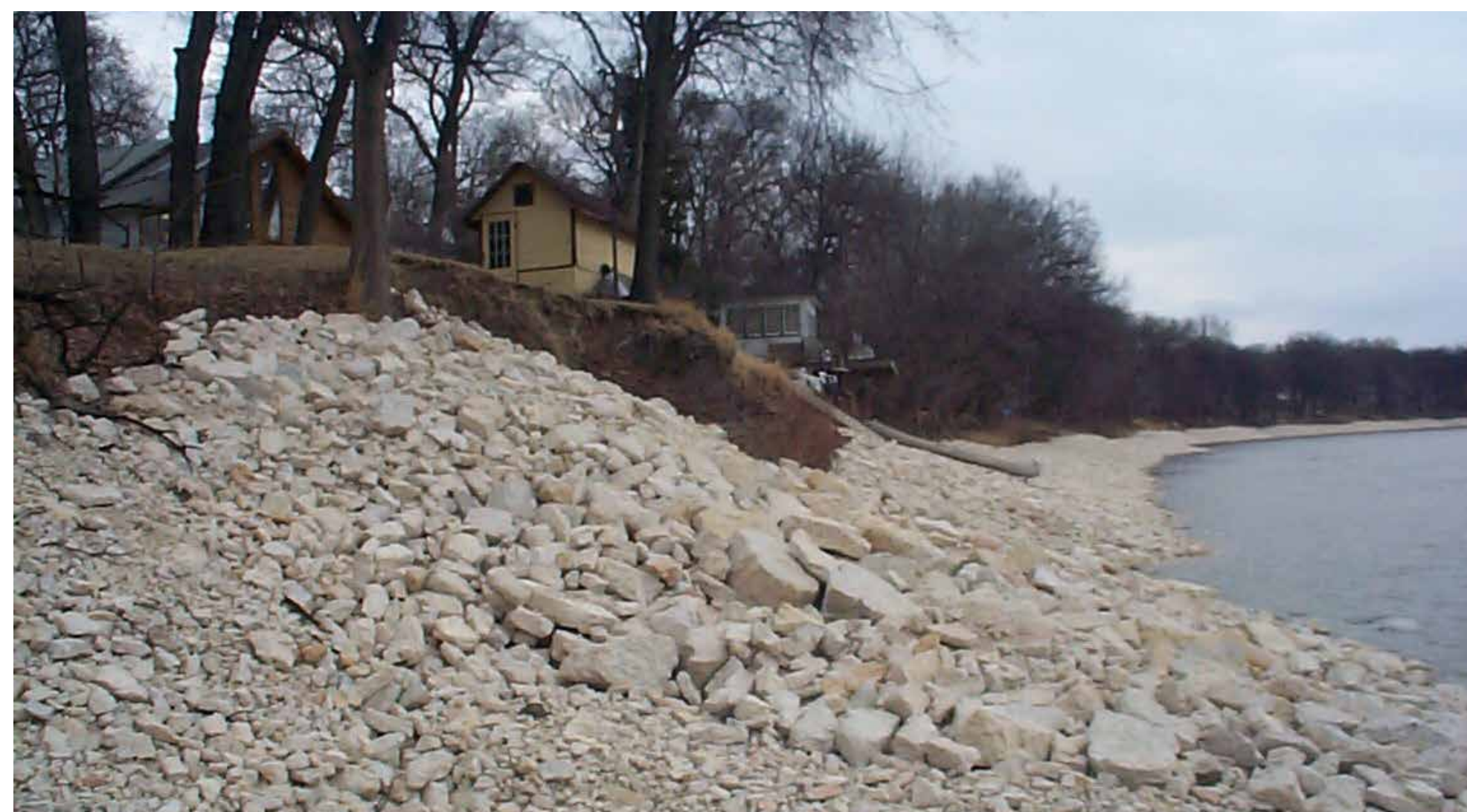
3 PLACING RIPRAP The rockfill columns are covered with clay and soil. A rockfill riprap blanket is placed along the shoreline to protect soils from erosion.
