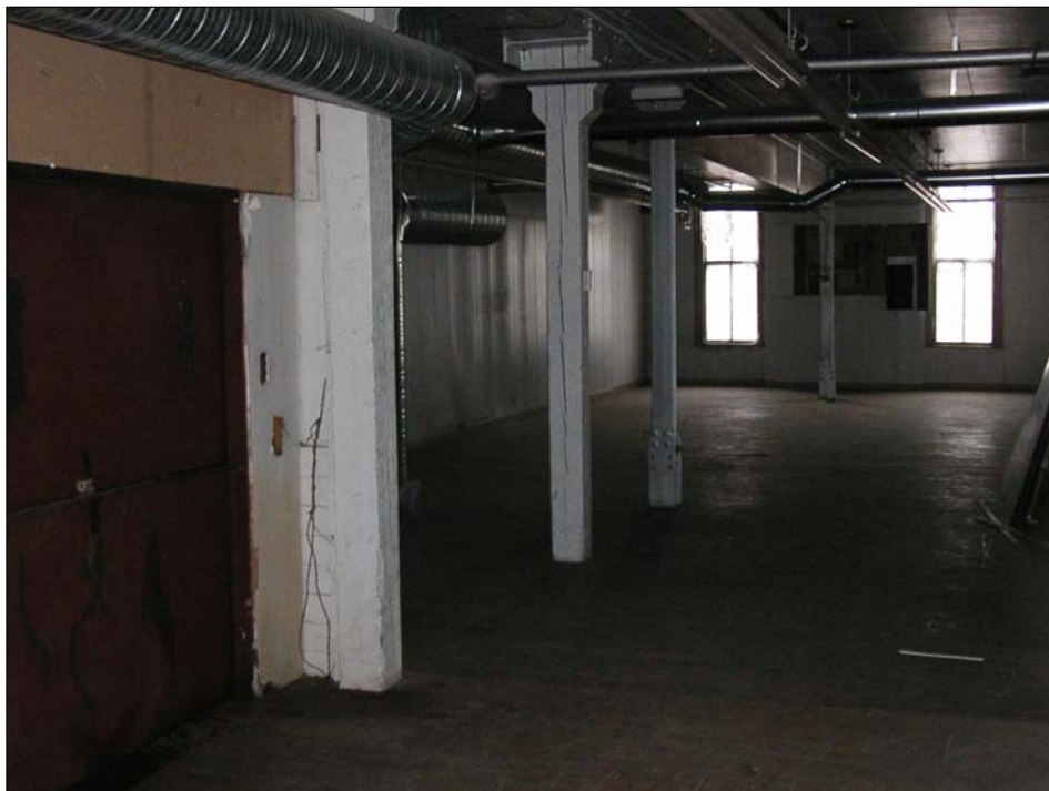
Plate 12 – Second floor posts, original wooden elements in foreground, steel replacement posts to rear (east end), 2004. ( M. Peterson, 2004. )
