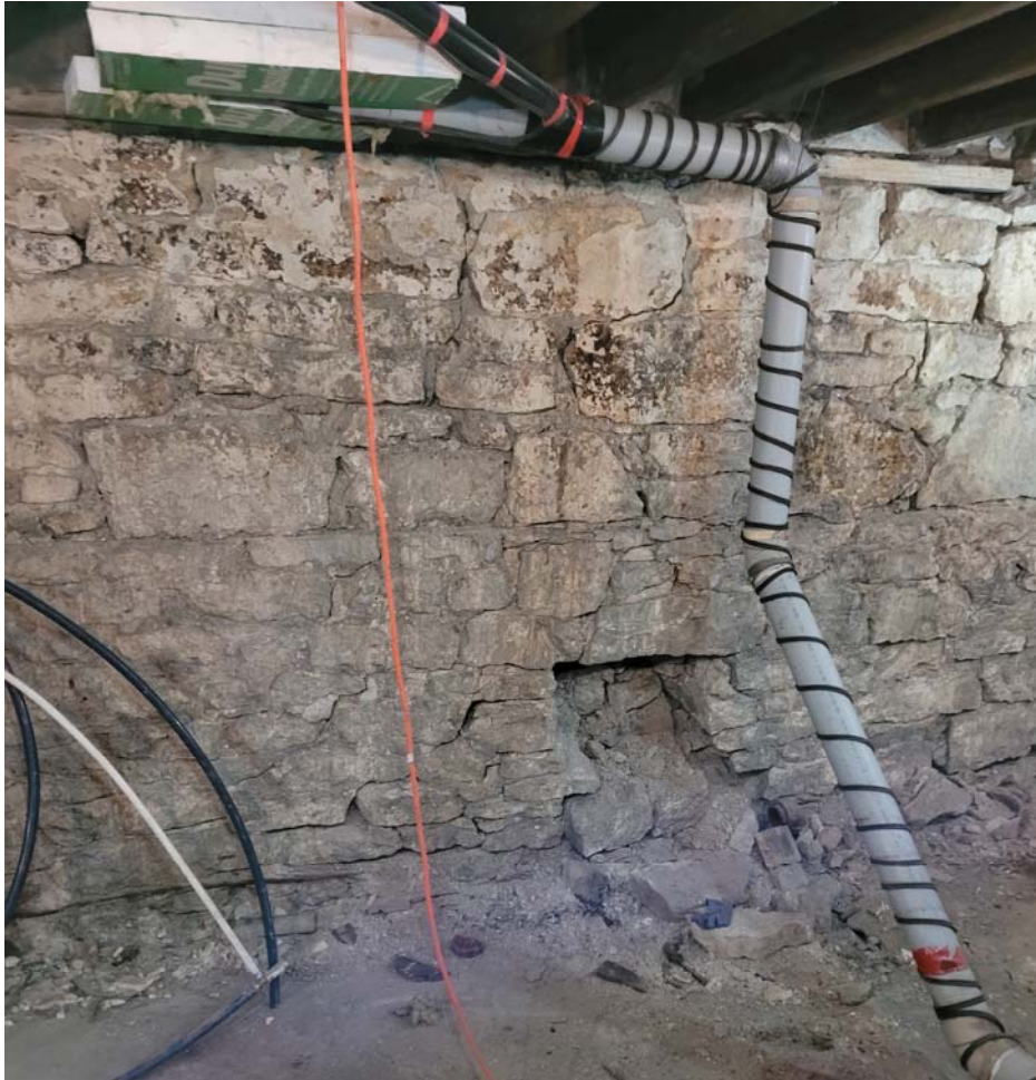
Photo 2: 242 Princess – Rubble wall bulge/damage at south-west corner.
