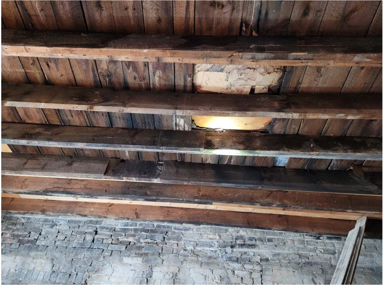
Photo 8: 242 Princess – Water damage and roof joists reinforcing spliced mid-span.
