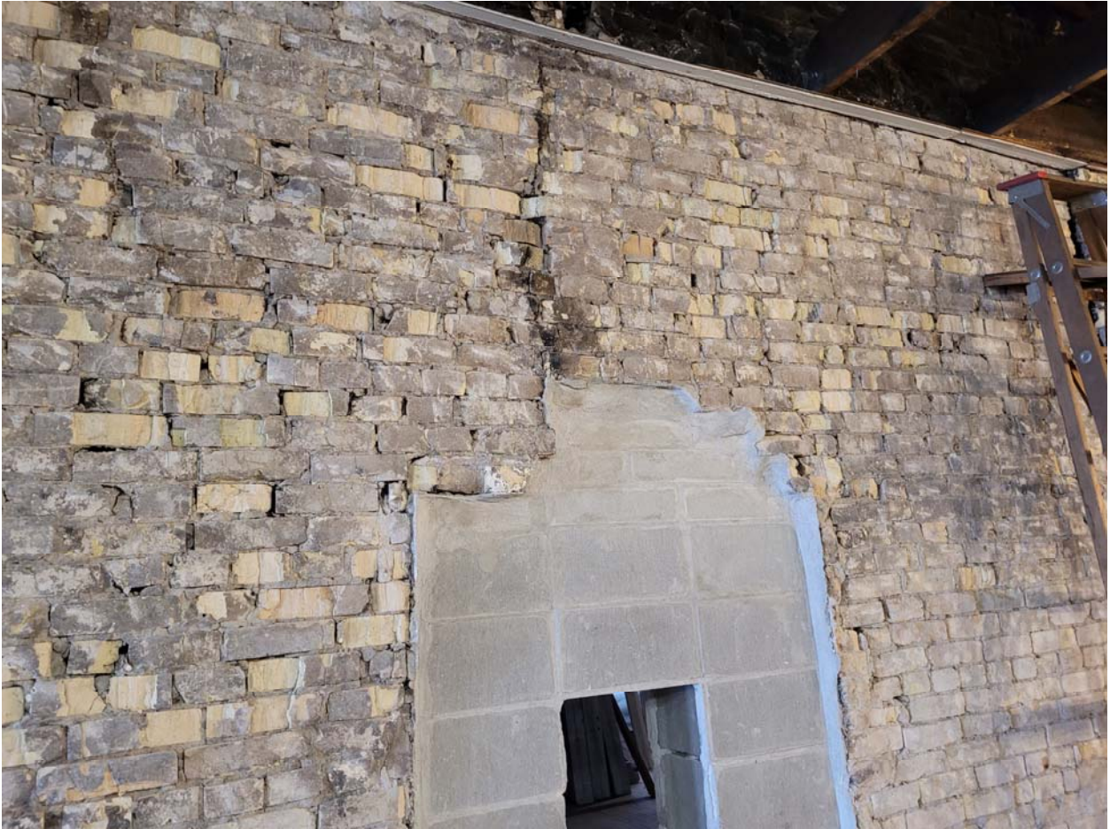
Photo 24: 244 Princess – Interior demising wall requiring repointing.
