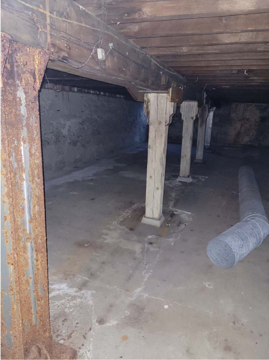
Photo 31: 244 Princess – Corrosion of columns in basement.
