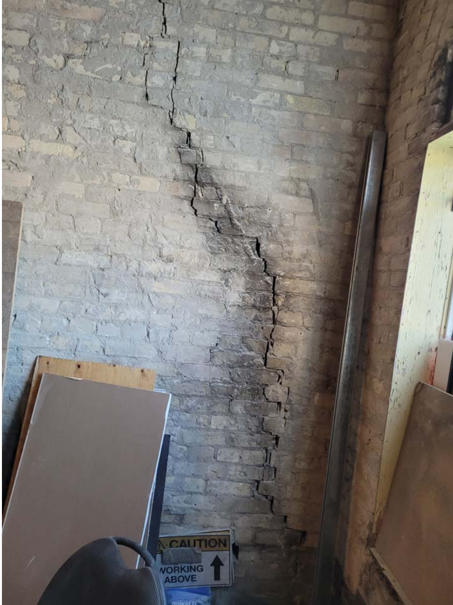
Photo 28: 244 Princess – Significant crack at demising wall at connection to east façade.
