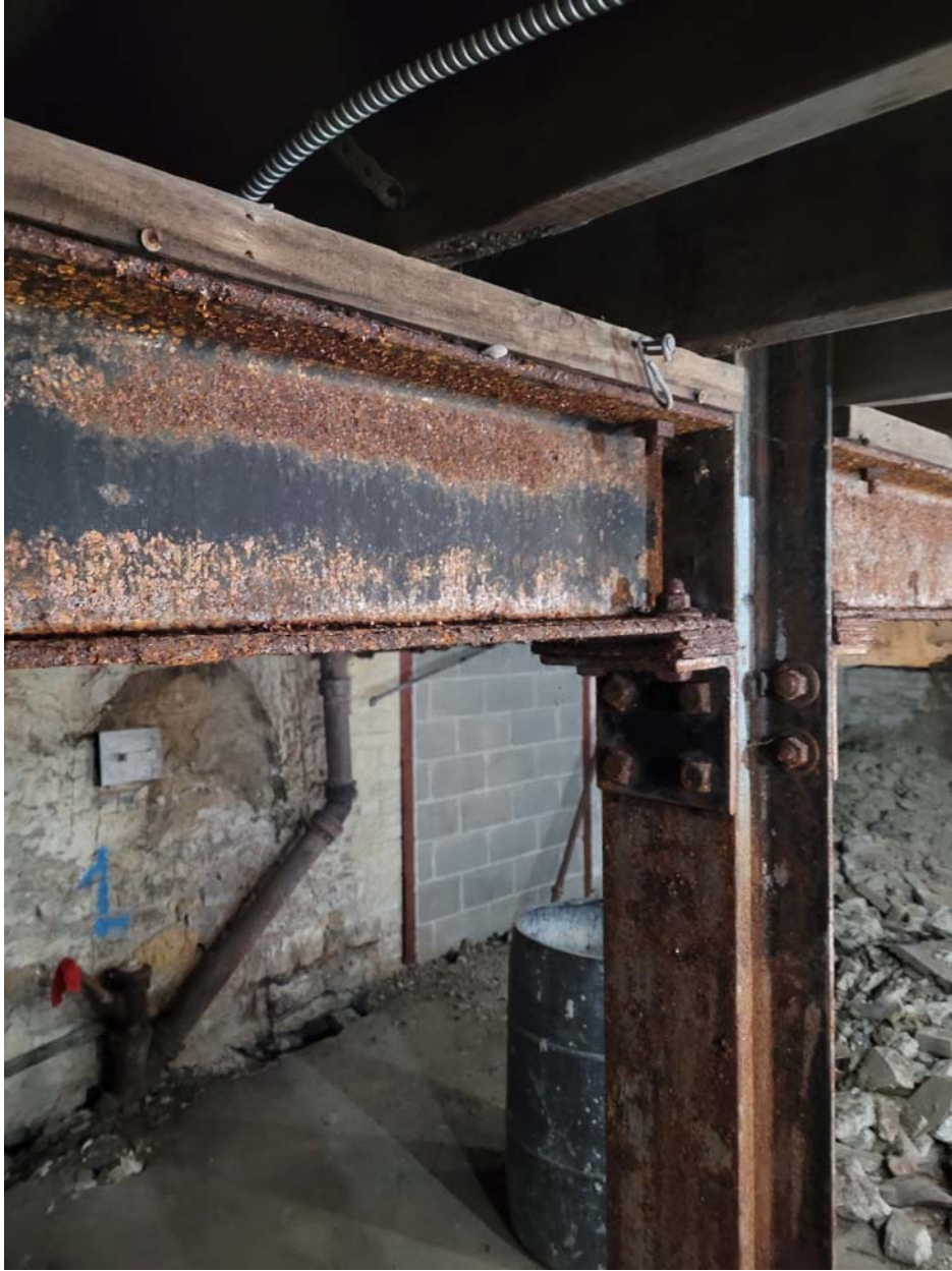
Photo 5: 242 Princess – Steel beam/column corrosion.
