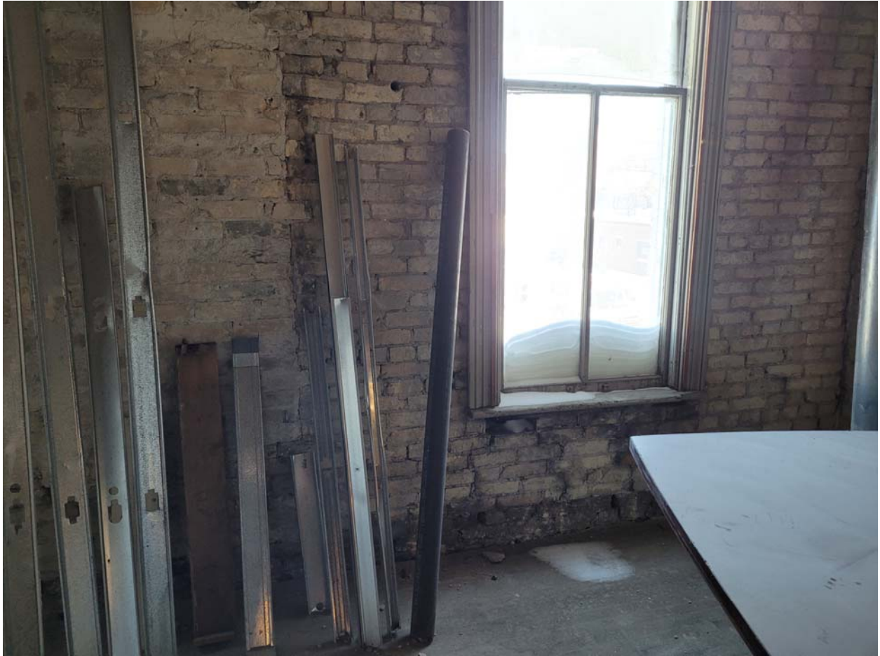
Photo 26: 244 Princess – Perimeter wall requiring repointing.
