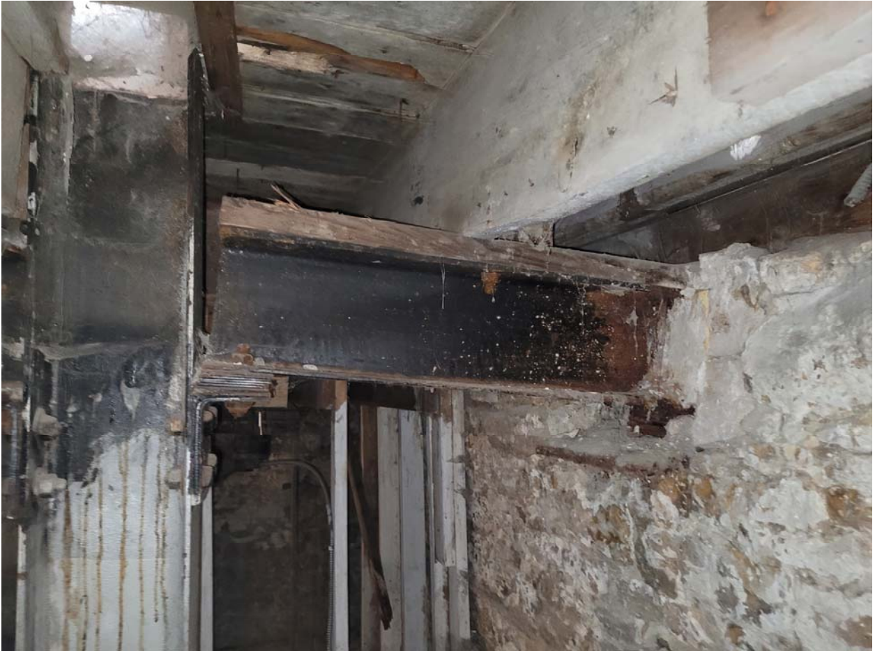
Photo 6: 242 Princess - Steel beam connection to east wall with signs of settlement.
