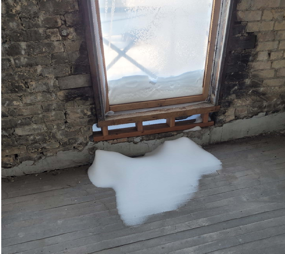
Photo 32: 246 Princess – Brick repair required at window on east façade
