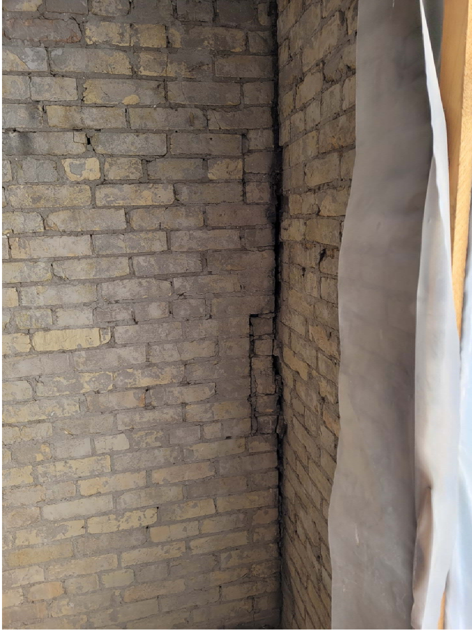
Photo 12: 242 Princess – Brick separation where east façade meet demising wall.
