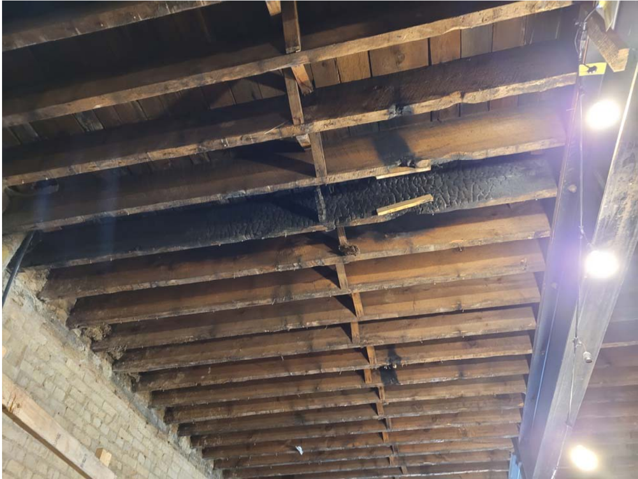
Photo 19: 242 Princess – Typical example of fire damaged joist.
