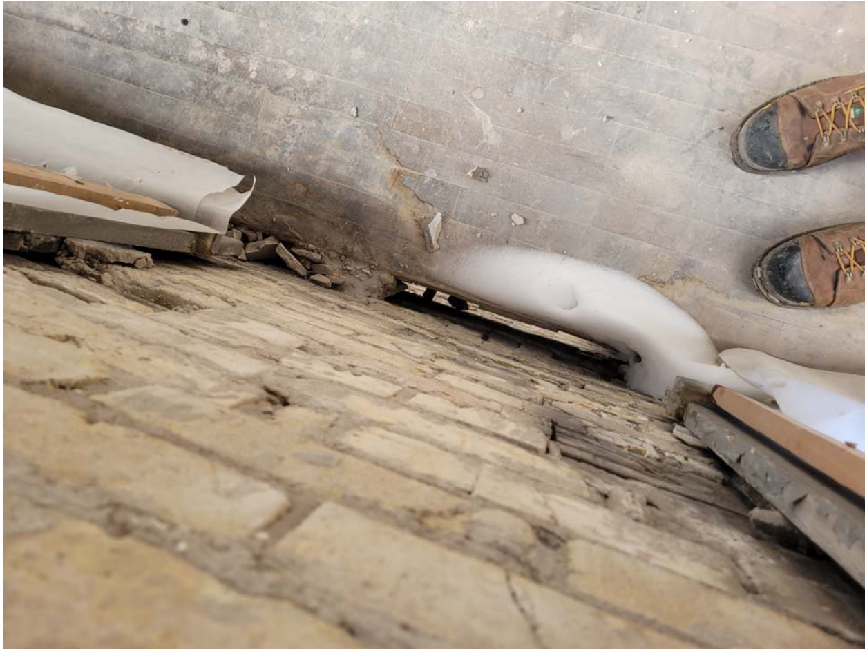
Photo 13: 242 Princess – Gap between east façade and third floor framing.
