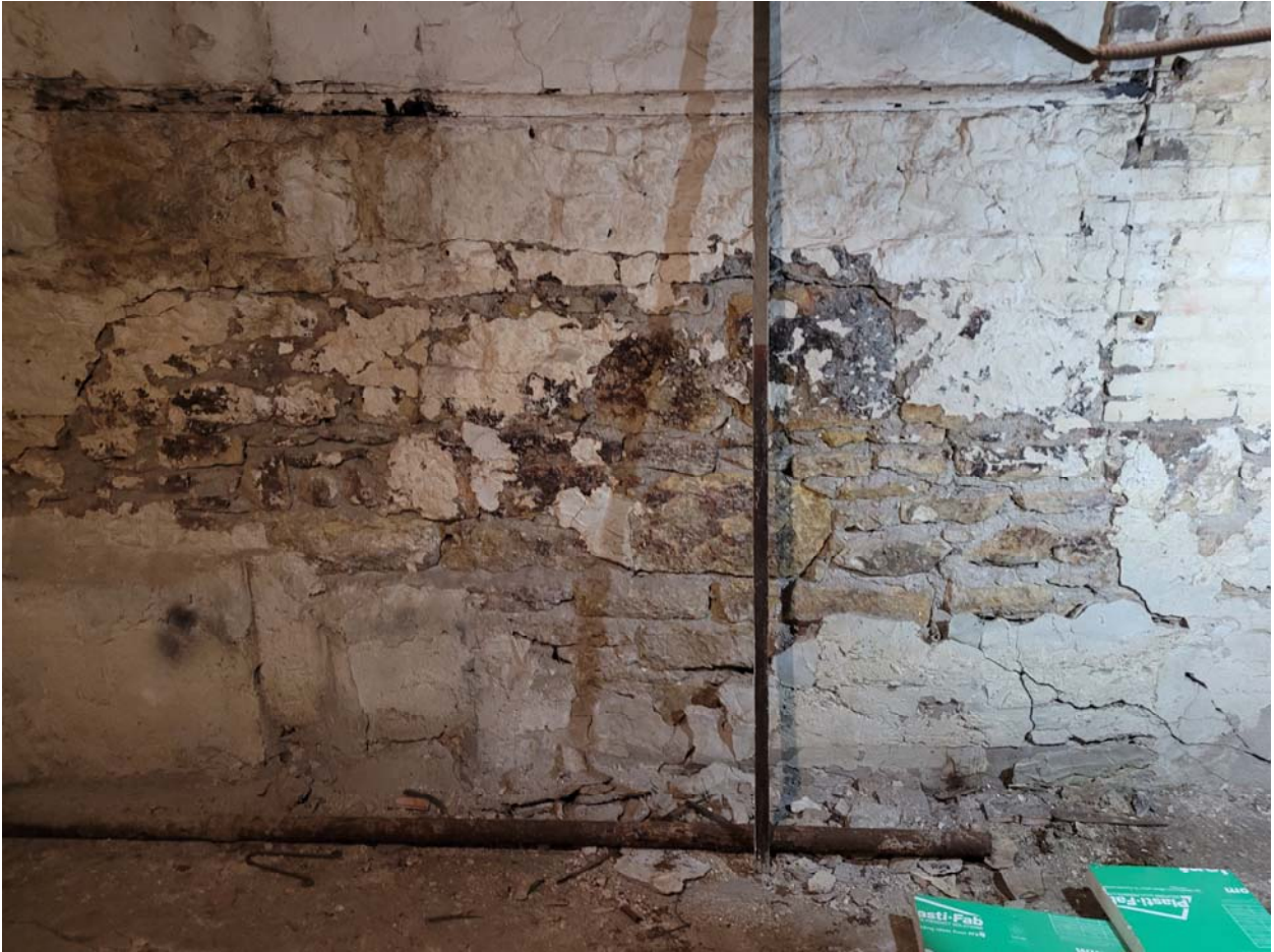
Photo 36: 246 Princess – Demising rubble wall requiring repointing.
