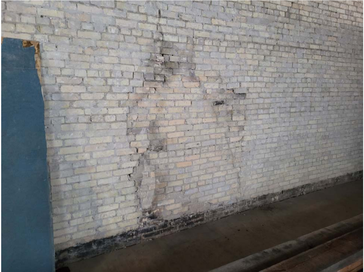
Photo 10: 242 Princess – Cracking and brick deterioration at center of dividing walls.
