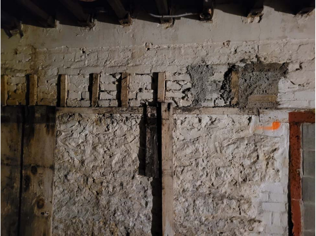
Photo 30: 244 Princess – Rubble demising wall requiring repointing.
