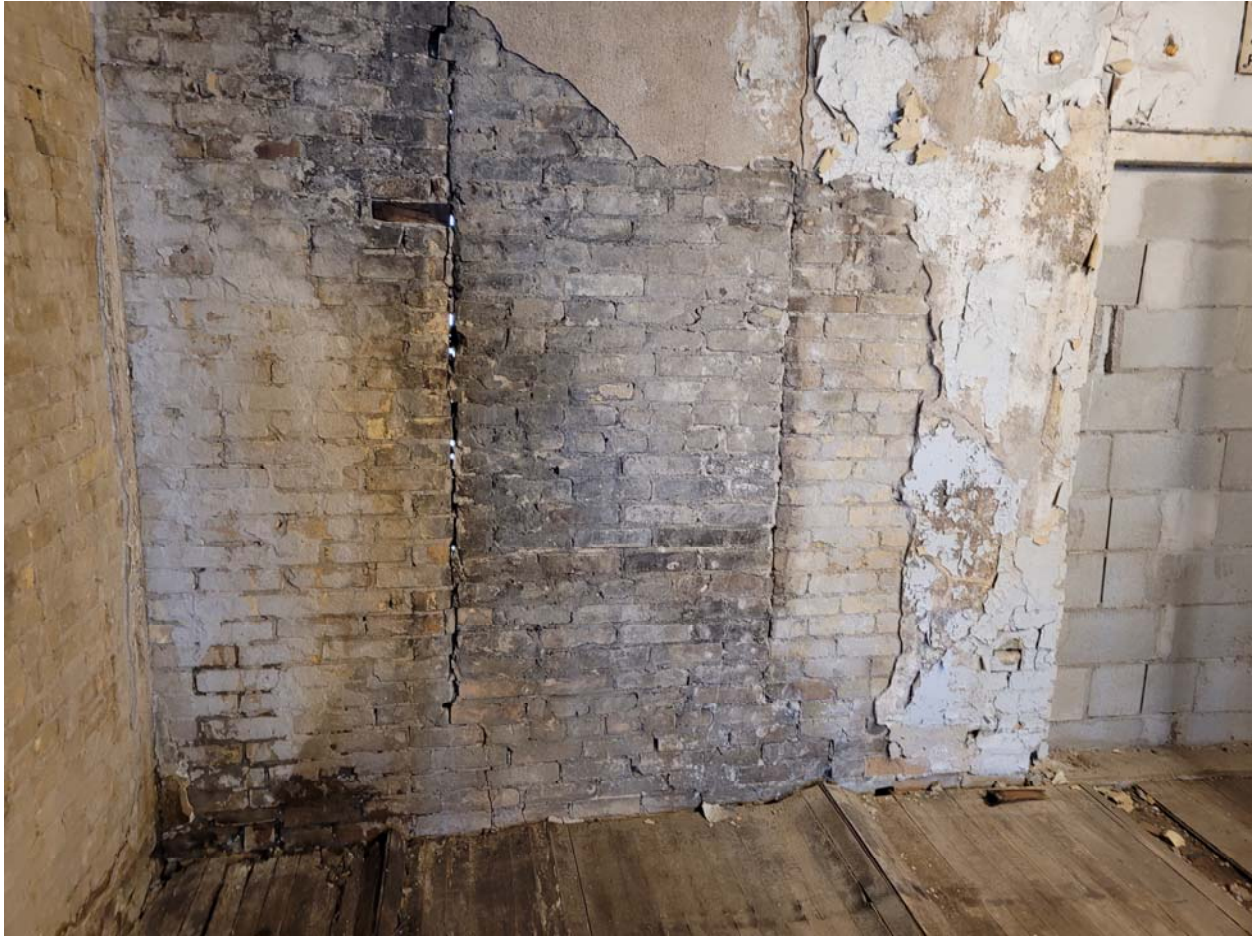
Photo 22: 244 Princess –Signicant crack in west façade.
