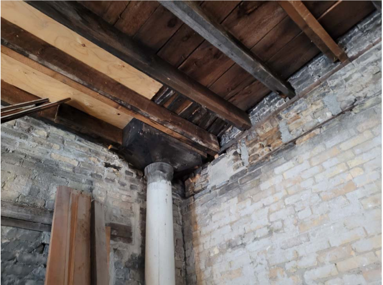
Photo 7: 242 Princess – Roof drain with damaged roof framing.
