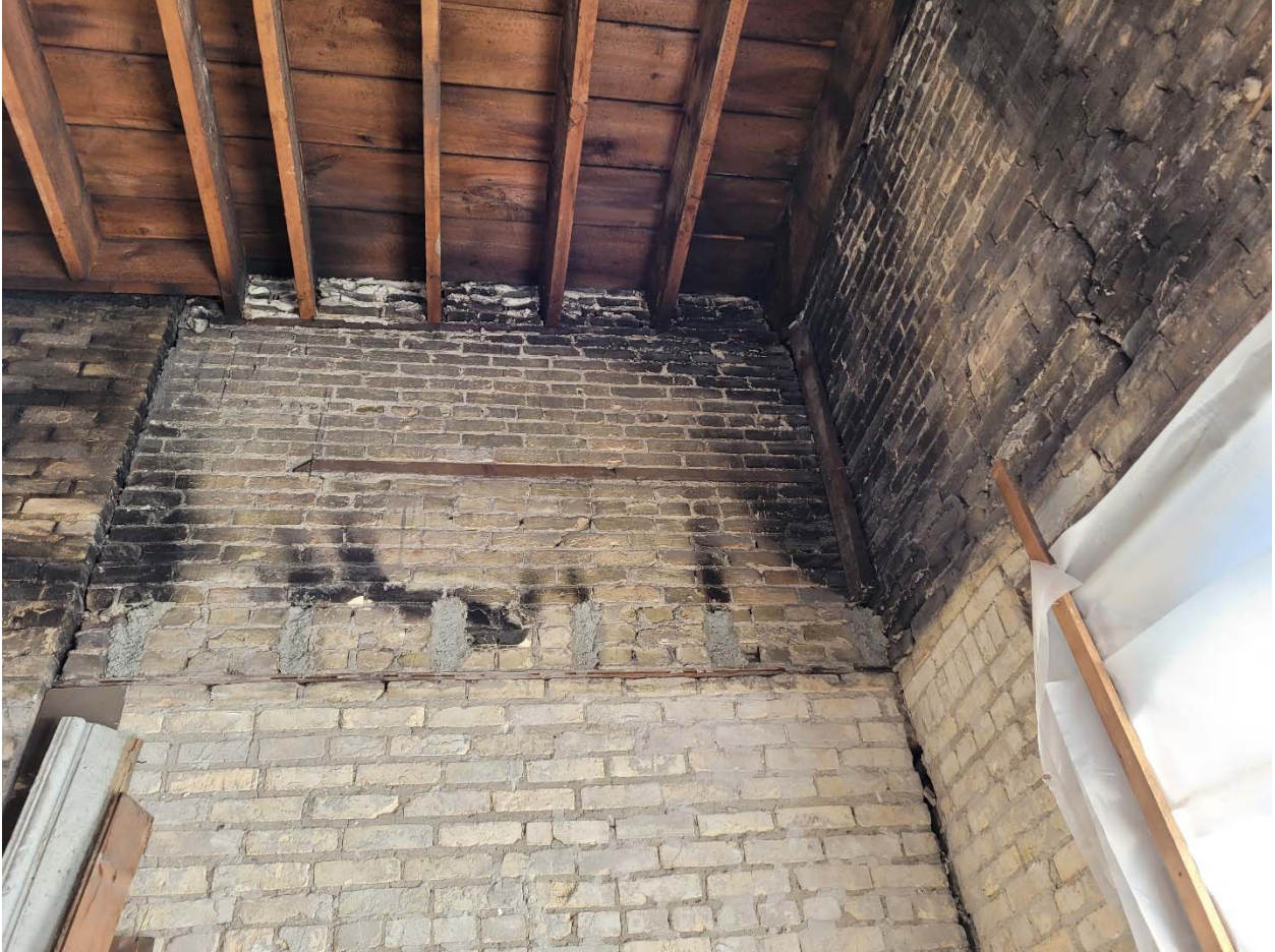
Photo 11: 242 Princess – Possible fire damage in north-east corner of roof framing.
