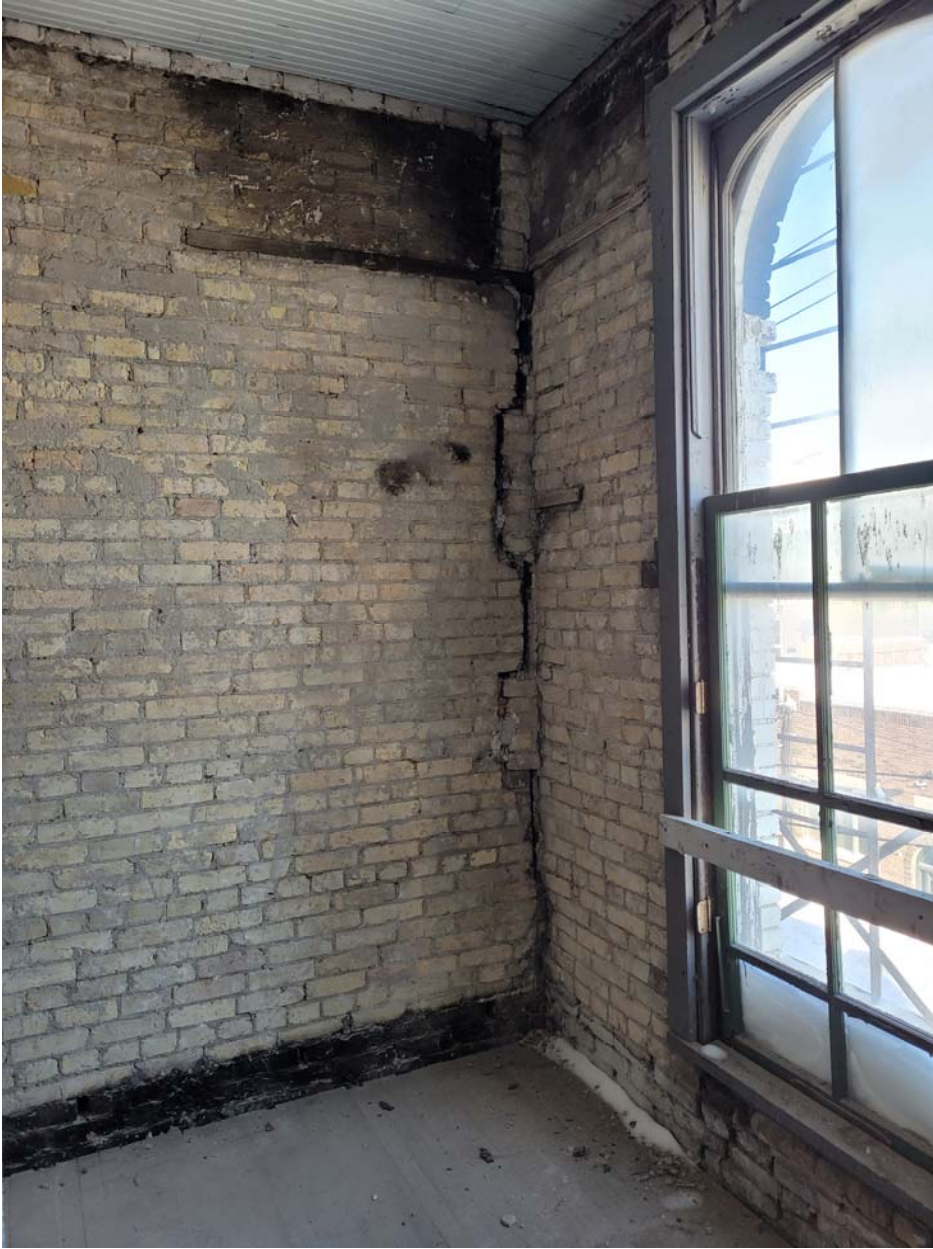
Photo 23: 244 Princess – Brick separation where east façade meet demising wall.
