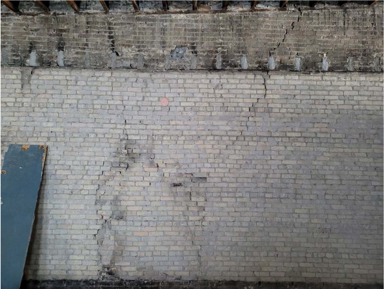
Photo 14: 242 Princess – Cracking and brick deterioration at center of dividing walls.
