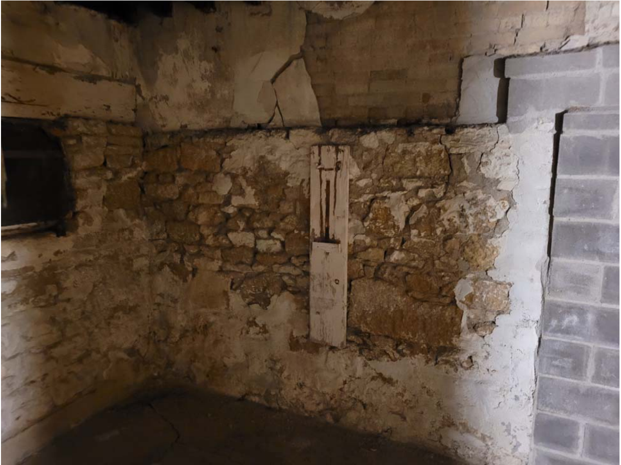
Photo 29: 244 Princess – Rubble demising wall requiring repointing.
