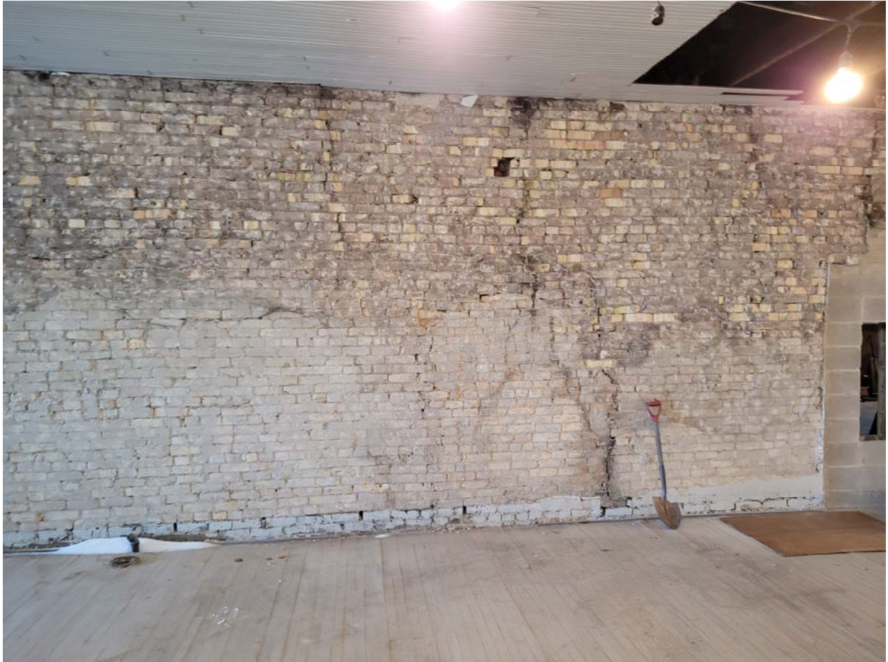
Photo 25: 244 Princess – Interior demising wall requiring repointing.
