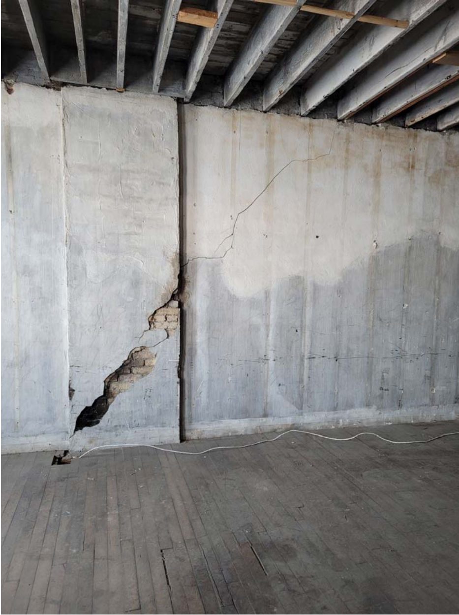
Photo 33: 246 Princess – Crack at demising wall near east façade with large crack.
