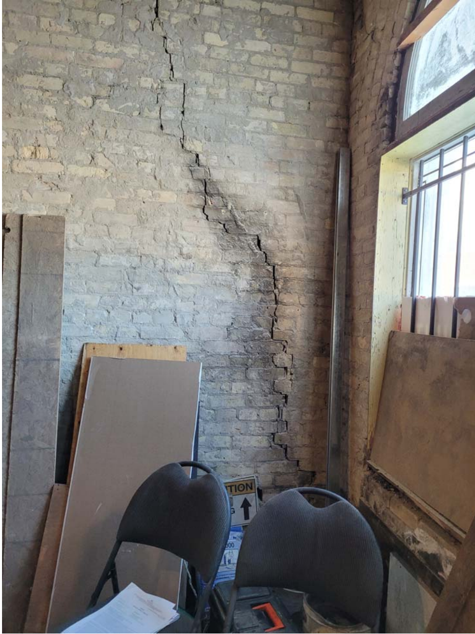
Photo 20: 244 Princess – Significant crack at demising wall at connection to east façade.
