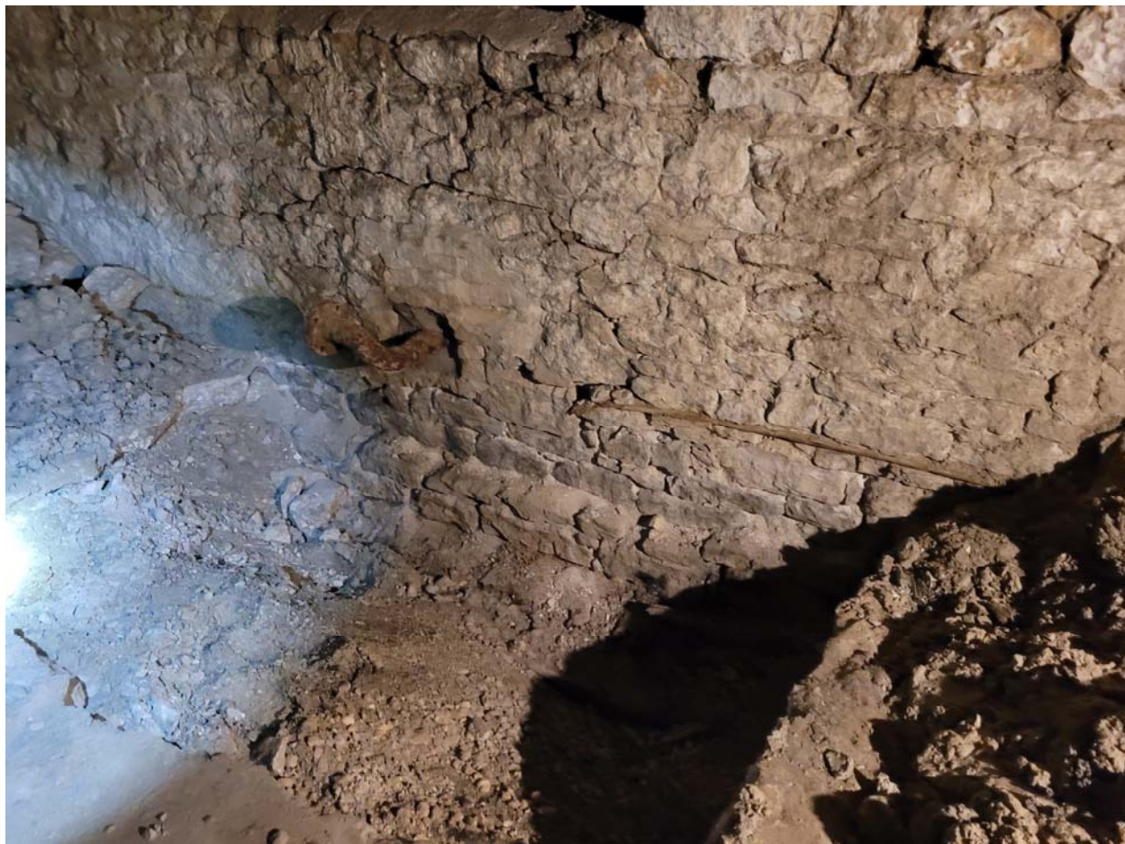
Photo 4: 242 Princess – Exposed foundation to be infilled and typical rubble wall requiring repointing.
