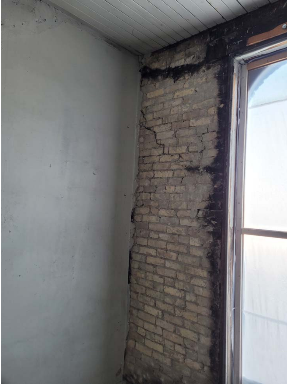
Photo 34: 246 Princess – Repointing required at east façade.
