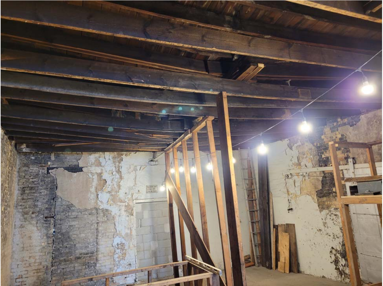
Photo 21: 244 Princess – Broken roof joists with shoring wall below.
