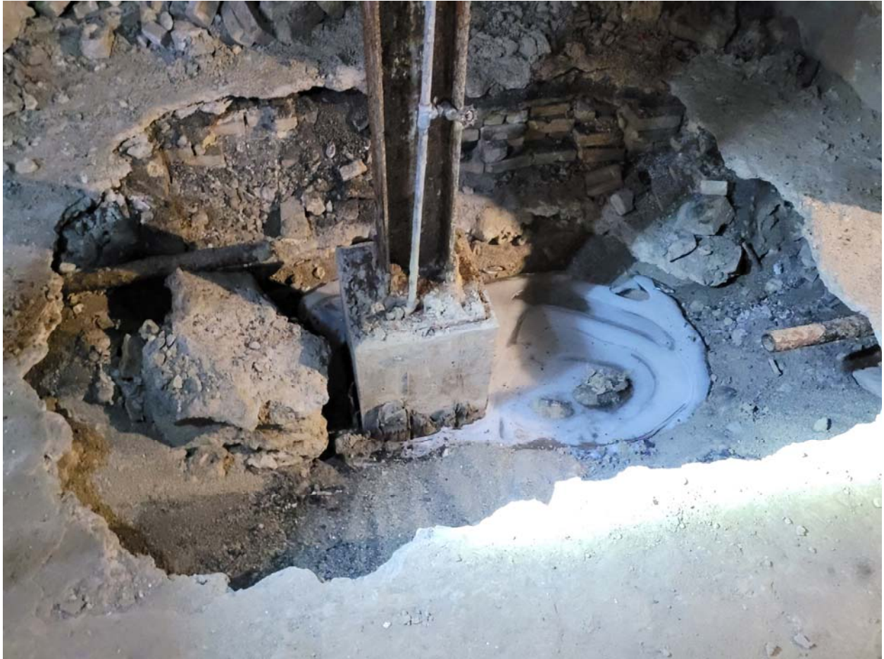
Photo 3: 242 Princess – Exposed foundation to be infilled.
