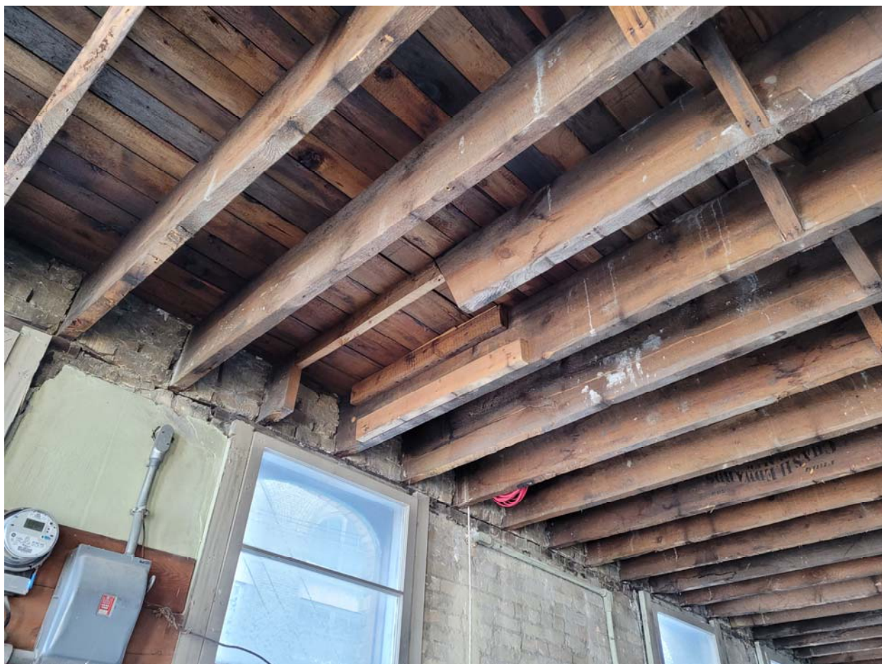
Photo 17: 242 Princess – Typical example of cut floor joists to be repaired
