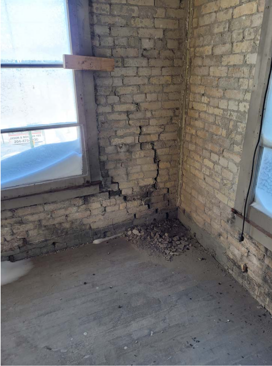
Photo 16: 242 Princess – Masonry cracking at south-east corner.
