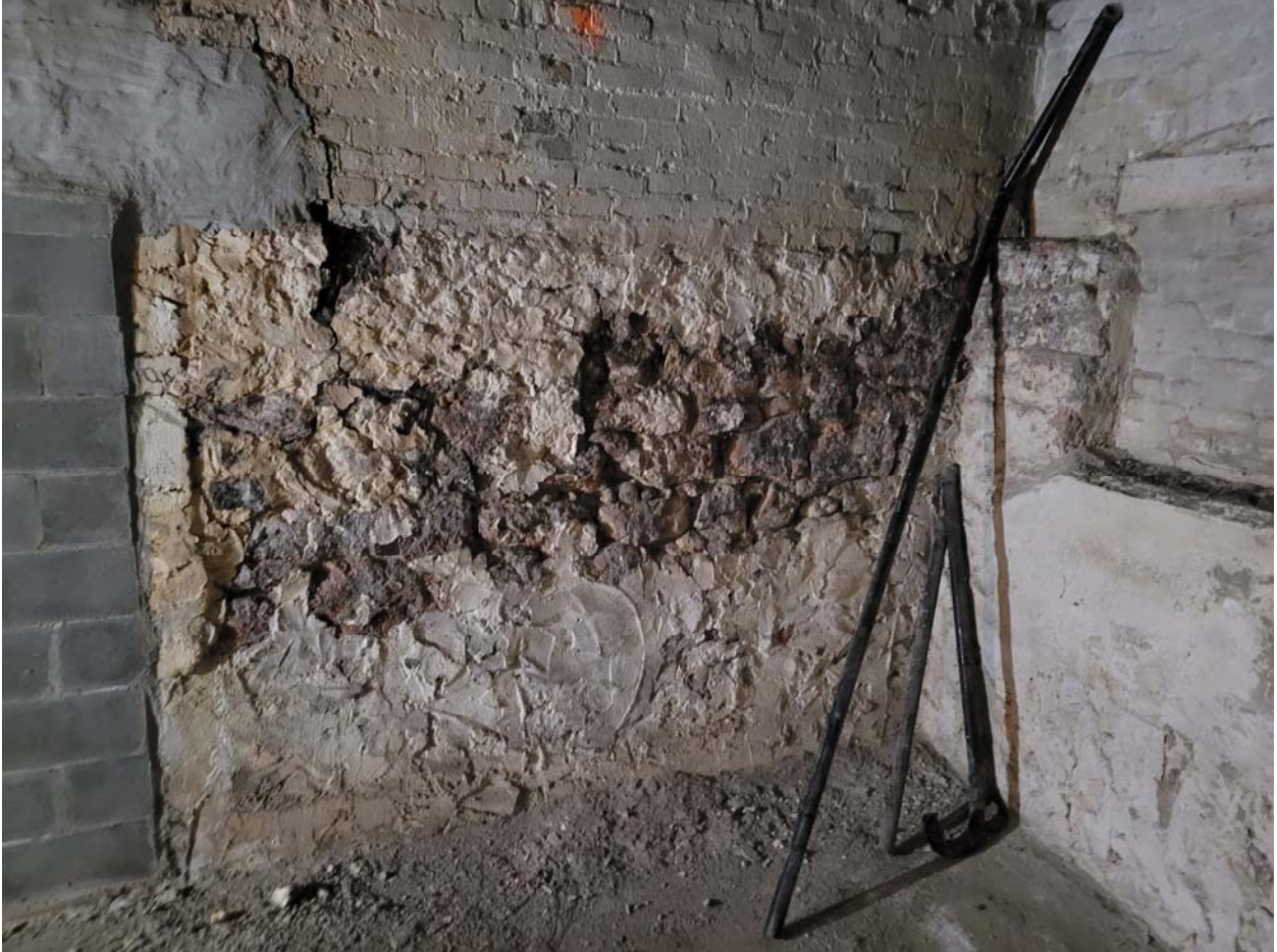
Photo 35: 246 Princess – Demising rubble wall requiring repointing.
