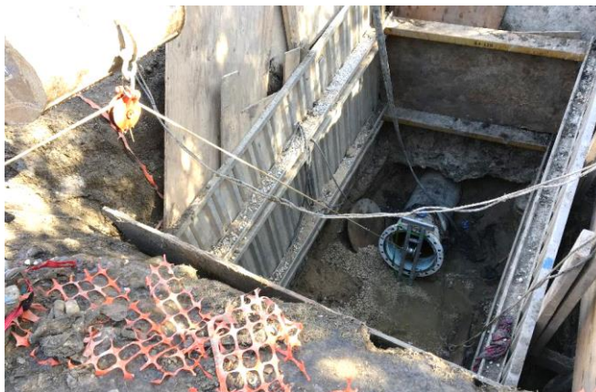
Figure 9. South Excavation winchline set-up.
