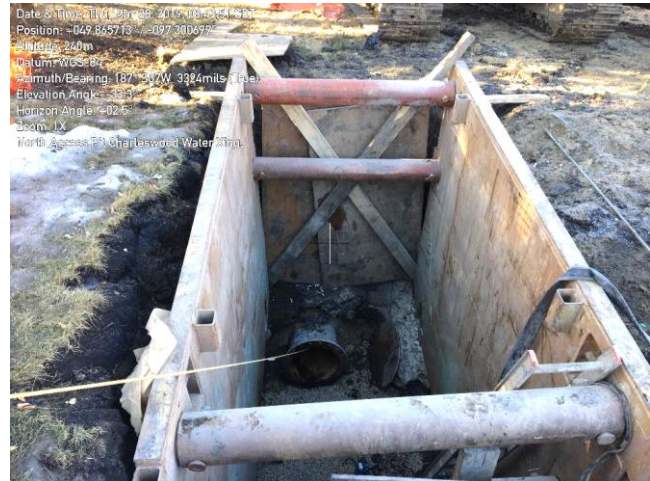
Figure 7. Tagline being pulled up at north excavation to pull south side winchline through the Feeder Main.
