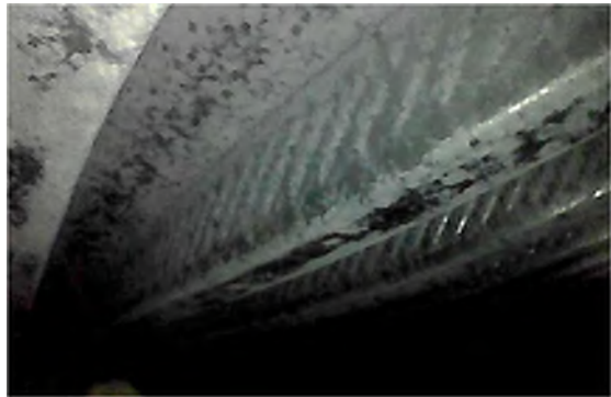
Figure 22: Stay-in-place Deck Forms at P1G2
