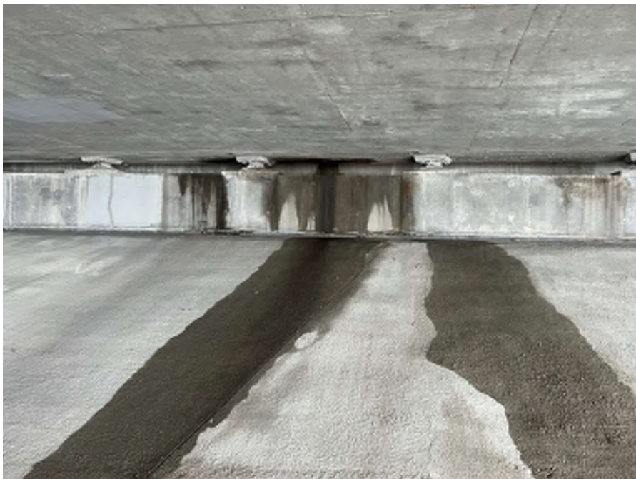
Photo 70 - Leakage on abutment seat and slope paving
