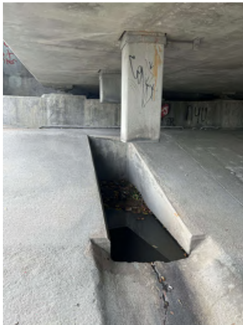
Photo 22 - Typical drains
