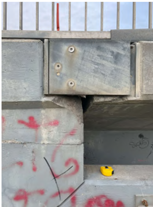
Photo 75 - Spall on corner of SE wingwall
