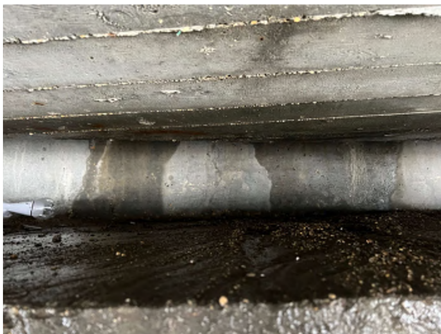
Photo 68 - Typical leakage on abutment backwall
