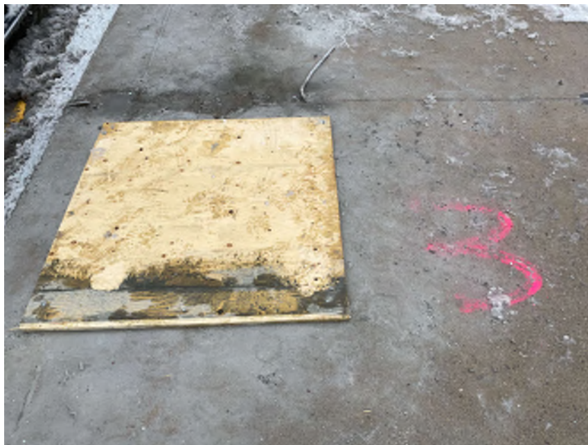
Photo 17 - Typical Test Pit temporary plywood covers
