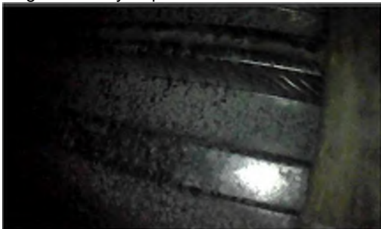
Figure 9: Stay-in-place Deck Forms at SAG7
