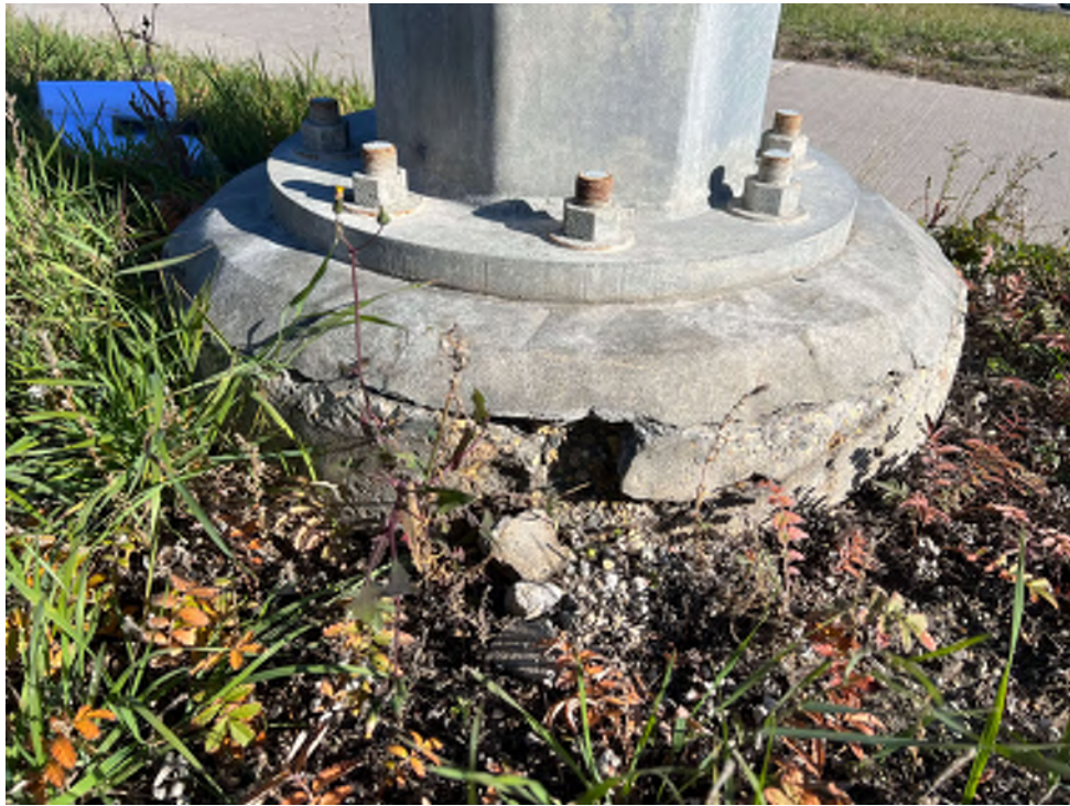
Photo 5 - Spalling on foundation top
