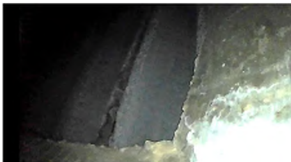
Figure 34: Stay-in-place Deck Forms at P3G9
