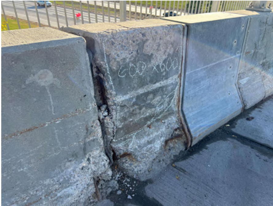
Photo 59 - NE approach barrier, delaminations near expansion joint
