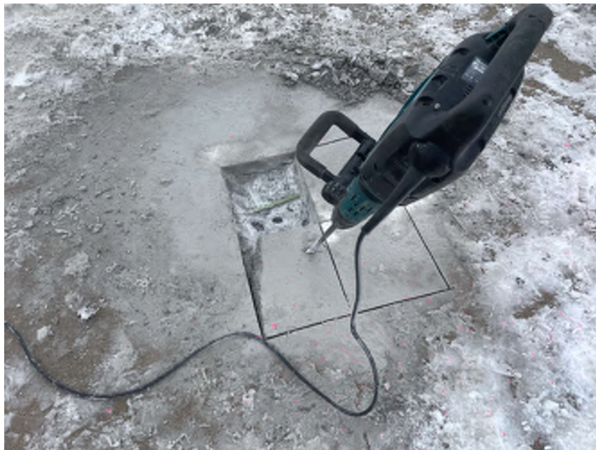
Photo 2 - Median Test Pit 1 - at start of removals, closer view
