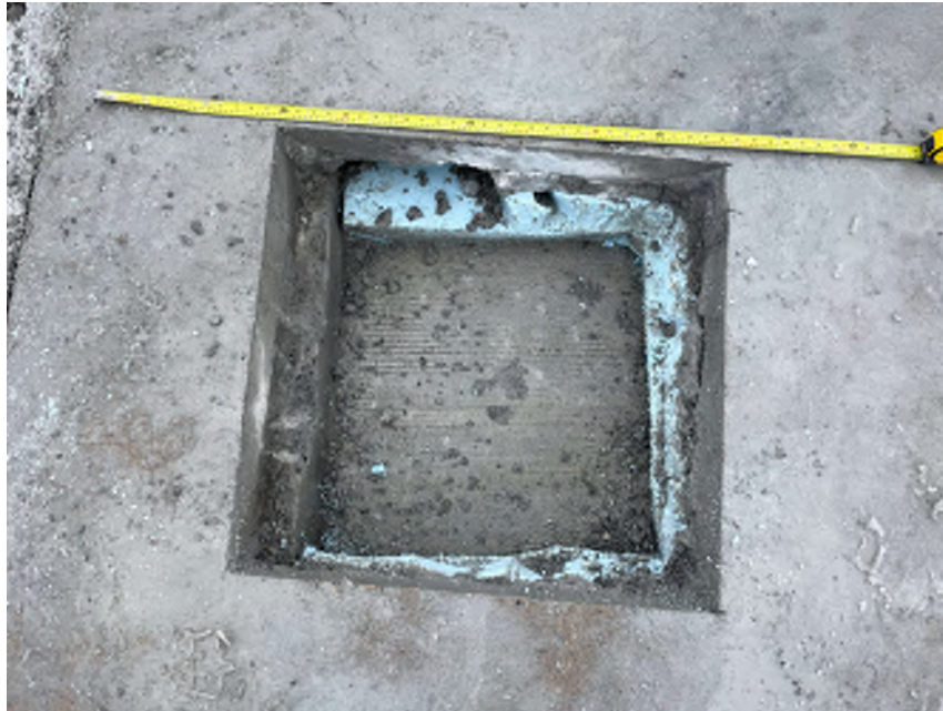
Photo 15 - Median Test Pit 3 - median slab concrete and styrofoam removed, concrete noted to be dry and in good condition, light flaking surface chipping occurred during s
