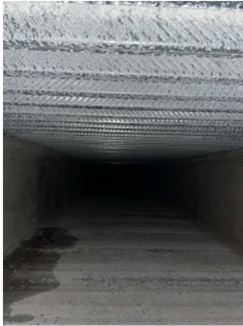
Photo 11 - Deck core hole D12, view inside box girders, note white corrosion oxidation product on SIP formwork
