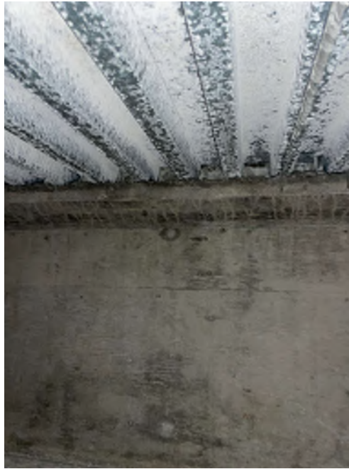
Photo 13 - Deck core hole D12, view inside box girders, girder web and top flange, note dampness and staining
