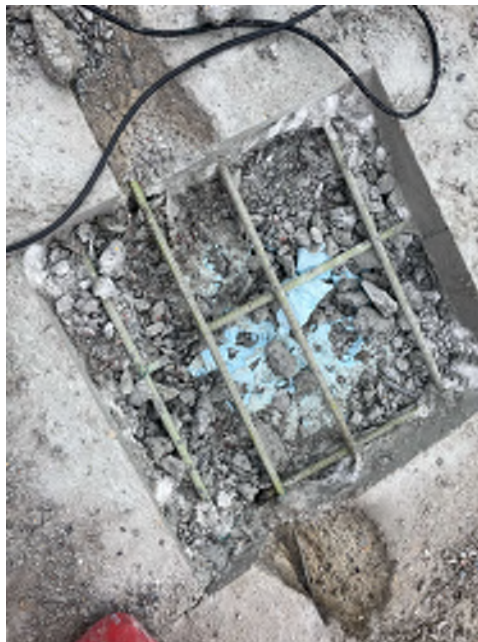
Photo 8 - Median Test Pit 2 - median slab concrete removed, styrofoam partially exposed, longitudinal bar under transverse joint corroded through
