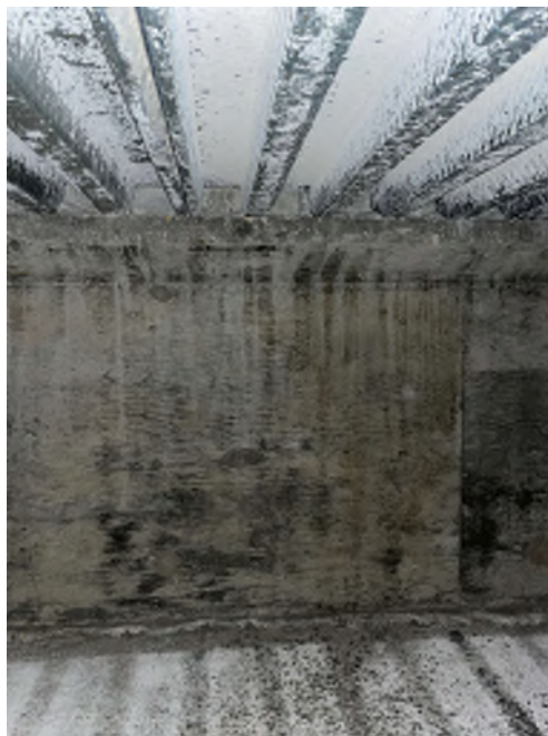
Photo16 - Deck core hole D29, view inside box girders, girder web and top flange, note dampness and staining, additional view
