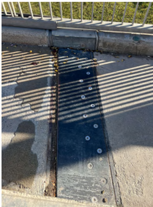
Photo 19 - SU1 expansion joint over sidewalk
