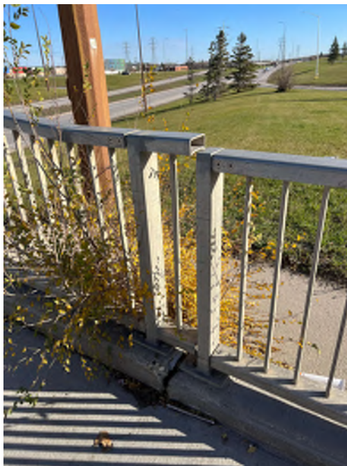
Photo 67 - Pedestrian handrail at SE corner showing differential settlement (~50mm)
