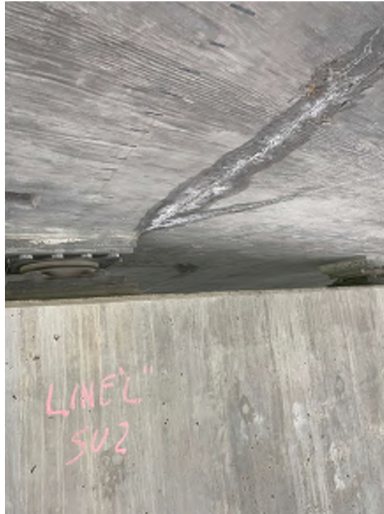
Photo 15 - Span 2, narrow crack with efflorescence and wetness near Line "L"
