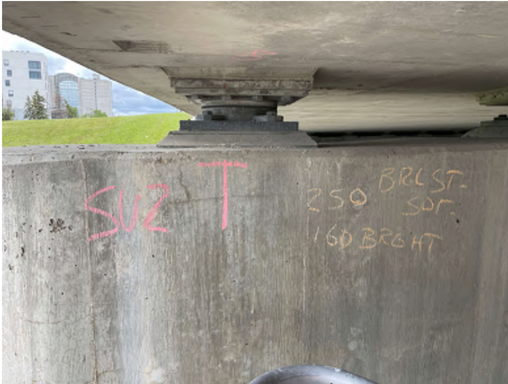
Photo 11 - SU2 Pier, Line "T" East exterior bearing
