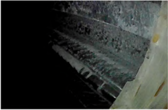
Figure 25: Stay-in-place Deck Forms at P1G5
