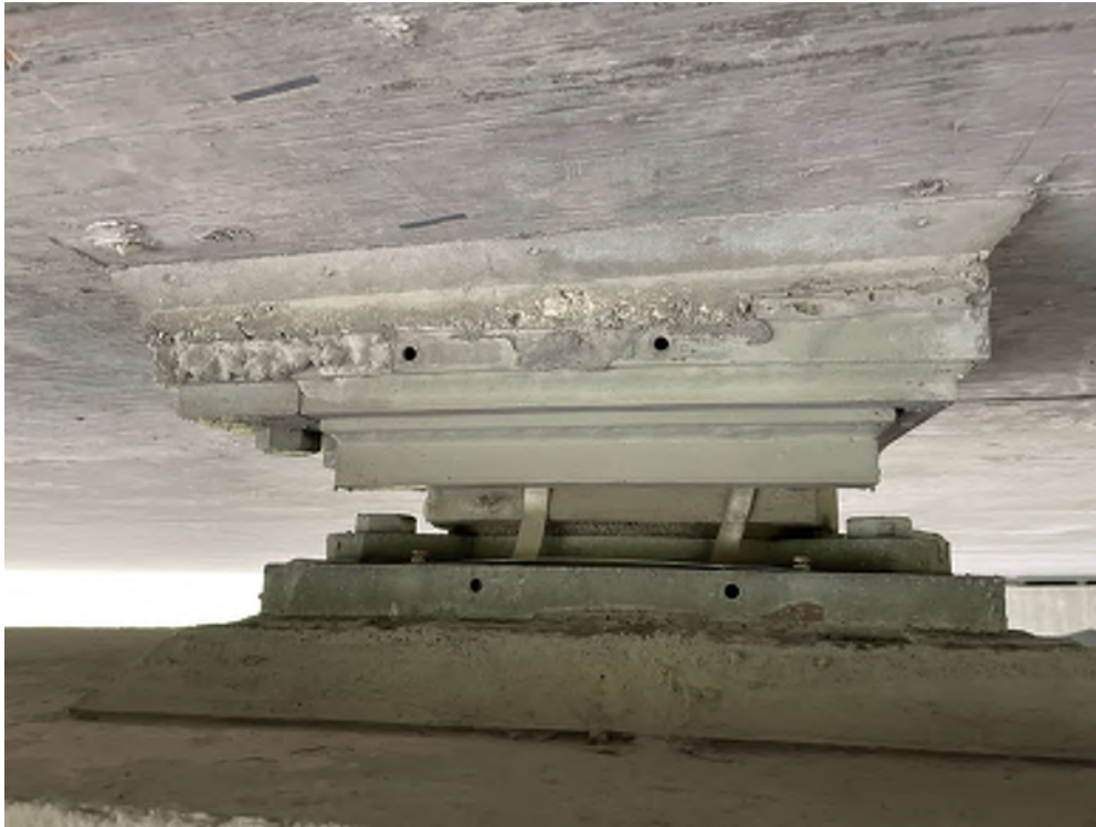
Photo 09 - SU3 Pier, Line "H" bearing, loose Teflon strips on south side, close up view
