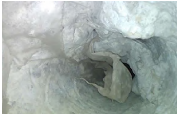
Figure 12: Blocked Drainage Hole at SAG12
