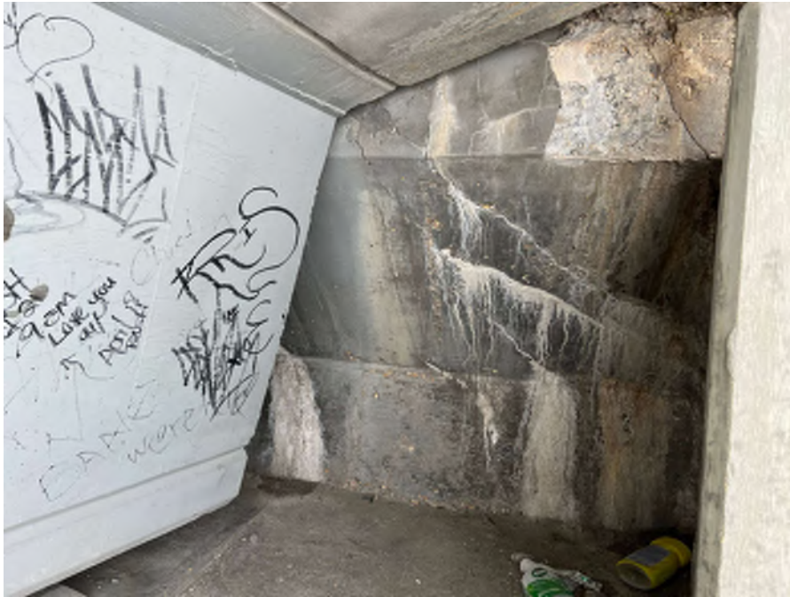
Photo 69 - SU5 abutment backwall cracking at East end
