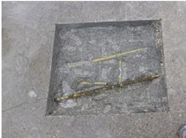
Photo 2.4 – Test Patch at Wide Crack with Failed Epoxy Coating and Corroded Reinforcing Directly Below Crack
