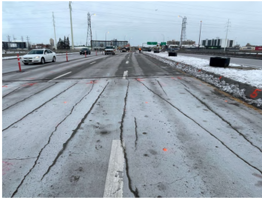
Photo 1 - Typical approach slab medium to wide longitudinal cracking
