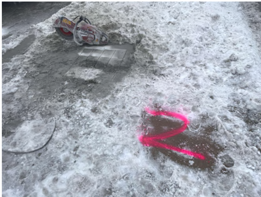
Photo 6 - Median Test Pit 2 - at start of removals, note deterioration at joint location
