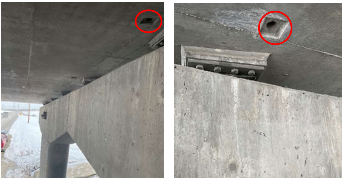
Figure 4: Typical View of Drainage Holes Used for Borescope Inspection
