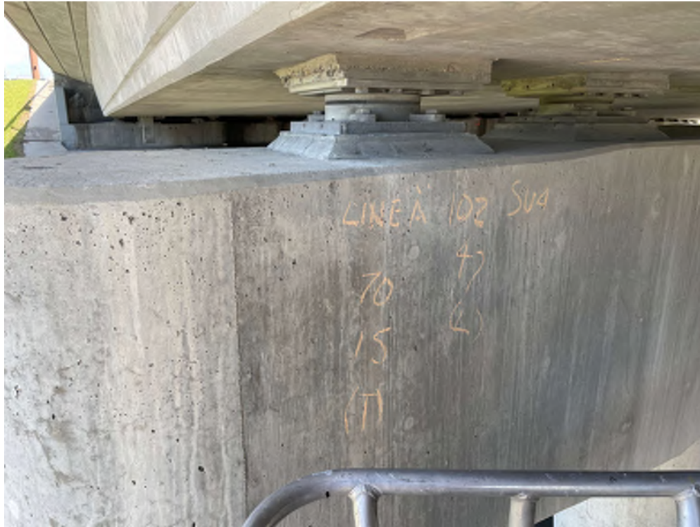
Photo 19 - SU4, Line "A" west exterior bearing
