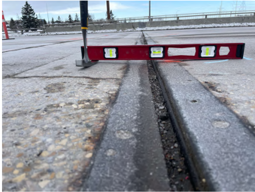
Photo 3 - Approach slab settlement, 10-20 mm noted at all approach slab locations, compared to deck blockout elevation
