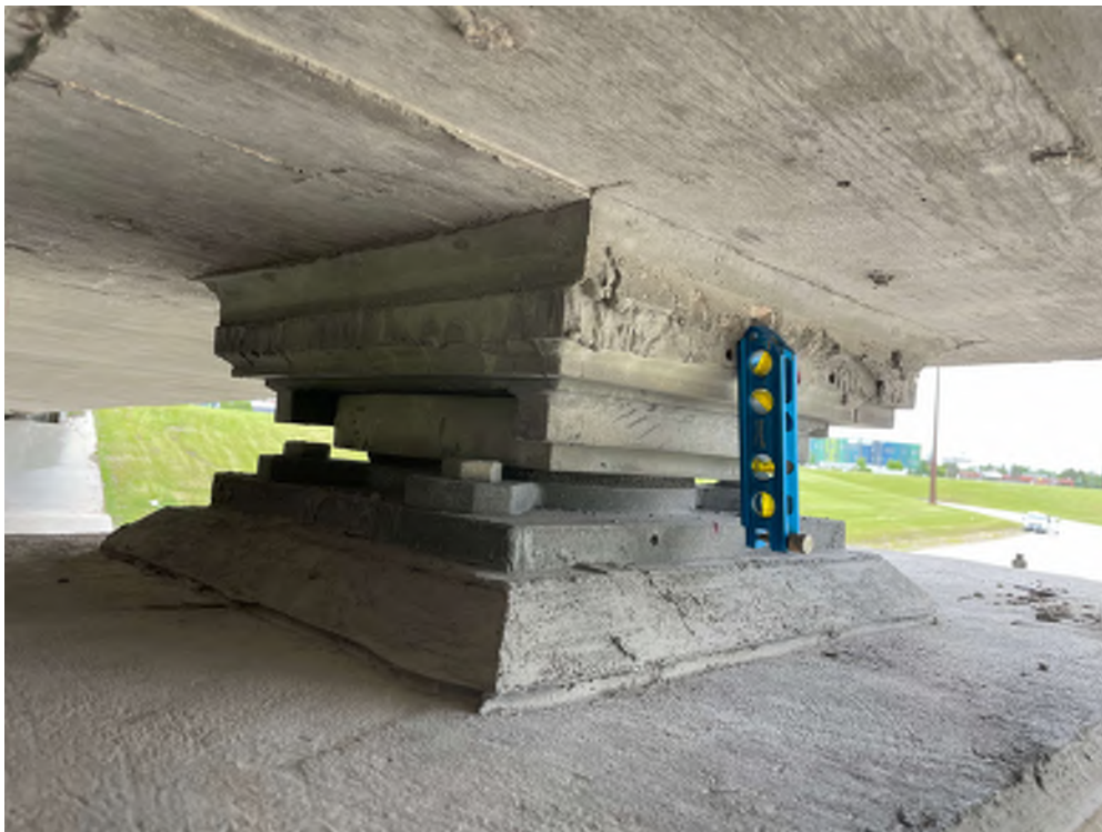
Photo 04 - SU3 Pier, Line "T" East exterior bearing
