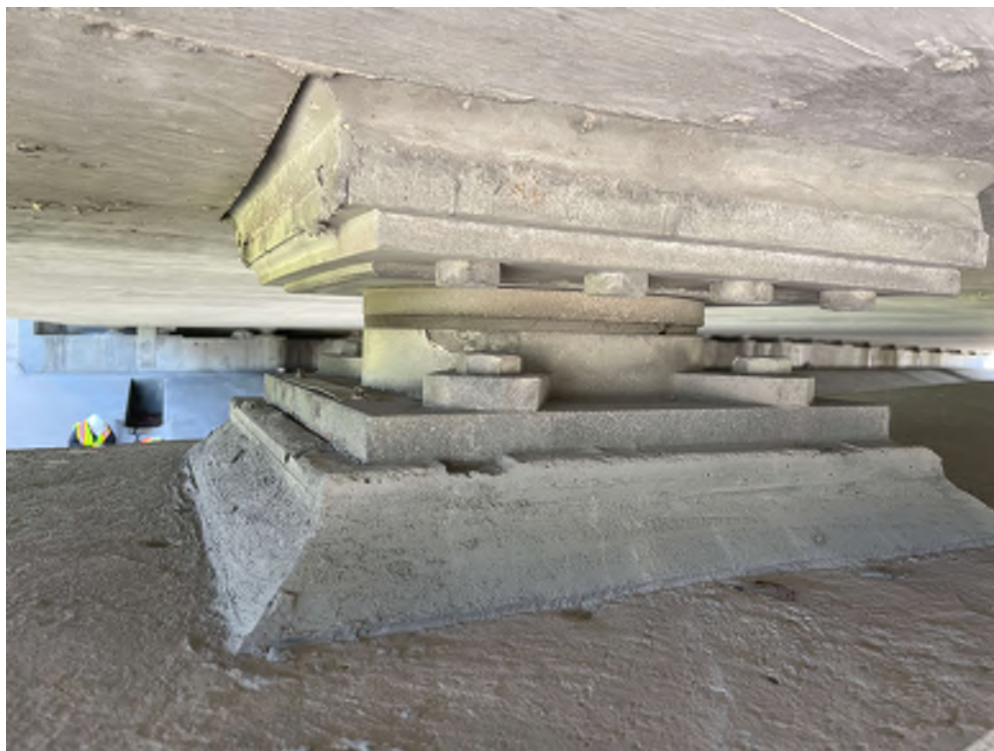
Photo 20 - SU4, Line "B" bearing, minor coating failure, Line "D" and "H" similar
