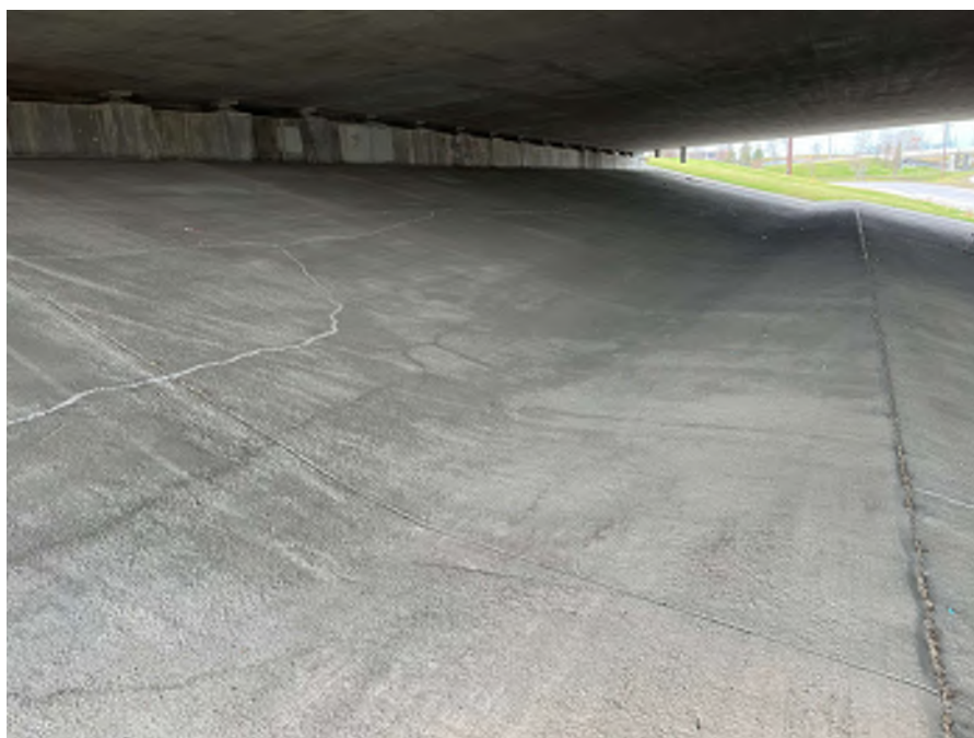
Photo 36 - South abutment slope paving - top portion
