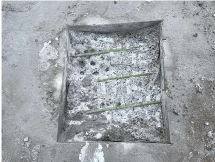
Photo 3 - Median Test Pit 1 - median slab rebar exposed, good condition
