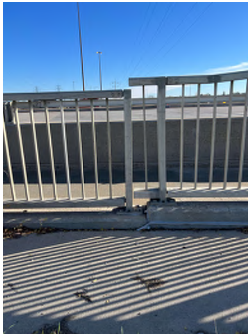
Photo 64 - Pedestrian handrail at NW corner showing differential settlement (~80mm)
