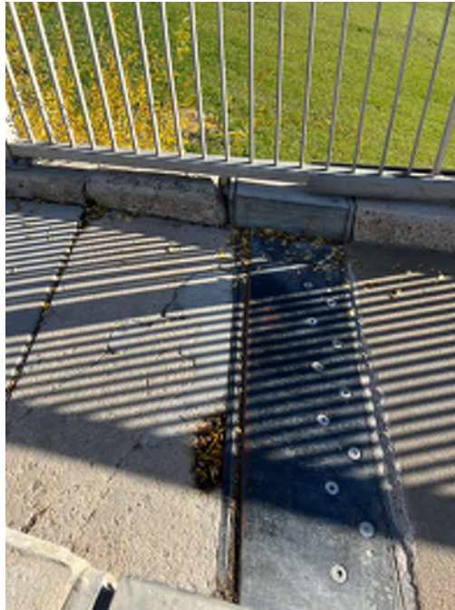
Photo 21 - SU5 expansion joint over sidewalk
