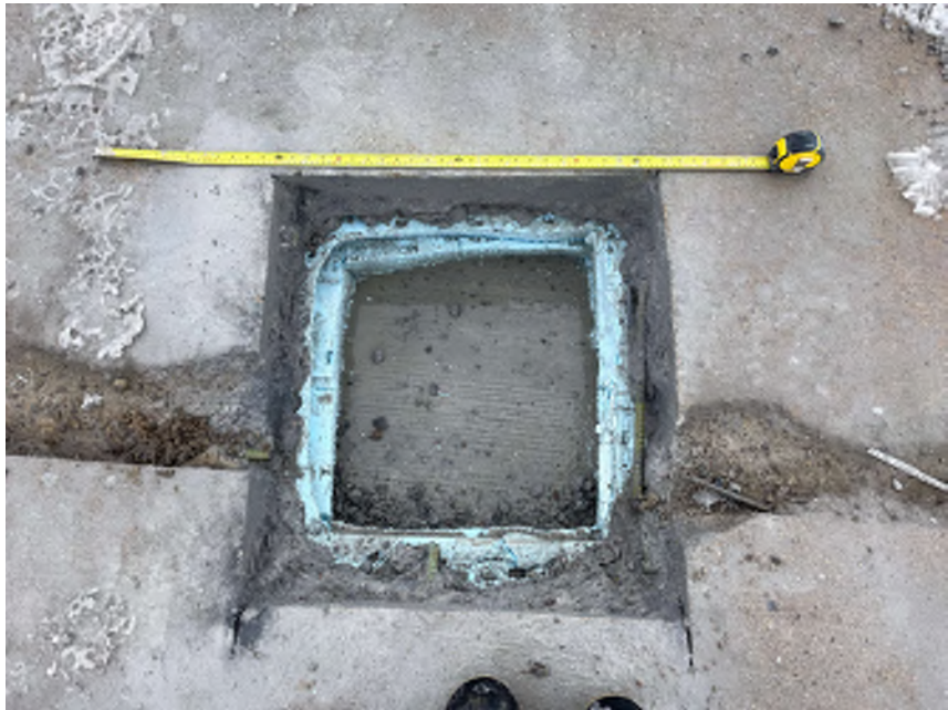
Photo 10 - Median Test Pit 2 - median slab concrete and styrofoam removed, concrete noted to be slightly wet and in good condition
