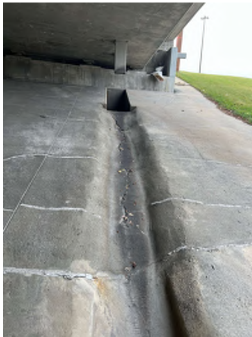
Photo 78 - SW drain gutter typical wide cracking on slope paving
