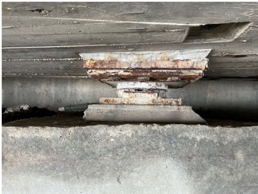
Photo 73 - SU5 abutment bearing 3 from East with corroded steel
