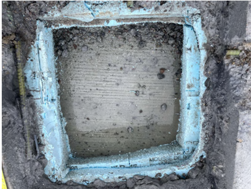
Photo 11 - Median Test Pit 2 - median slab concrete and styrofoam removed, concrete noted to be slightly wet and in good condition, closer view
