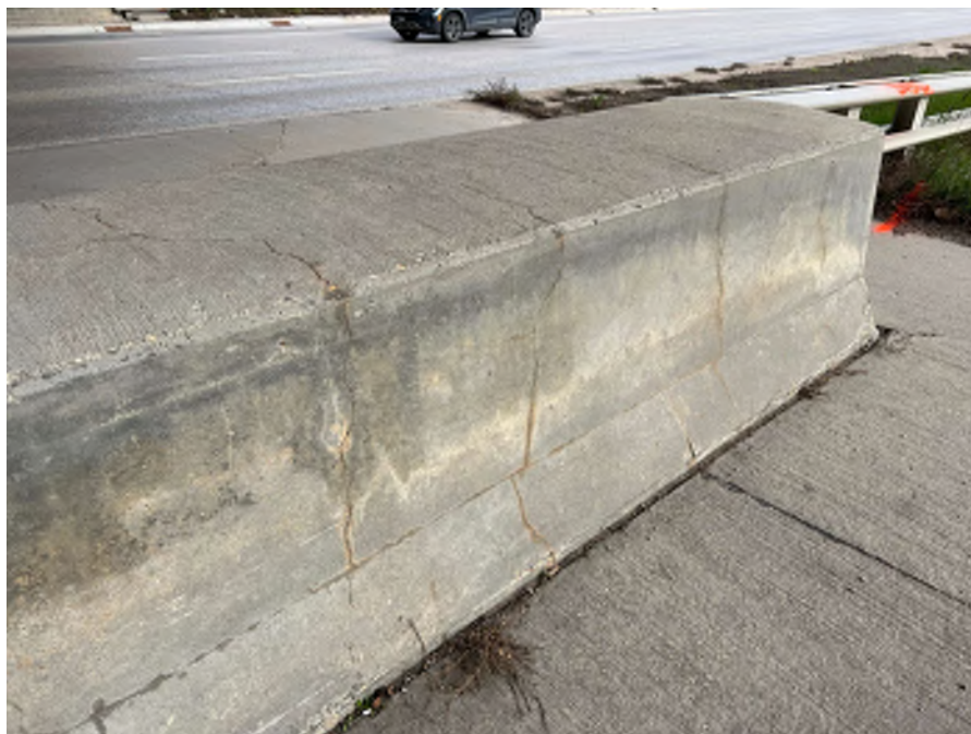
Photo 80 - Typical narrow vertical cracks on pier base pedestals
