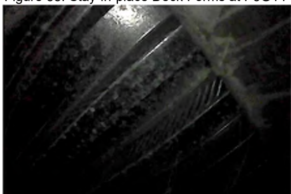
Figure 40: Stay-in-place Deck Forms at P3G16
