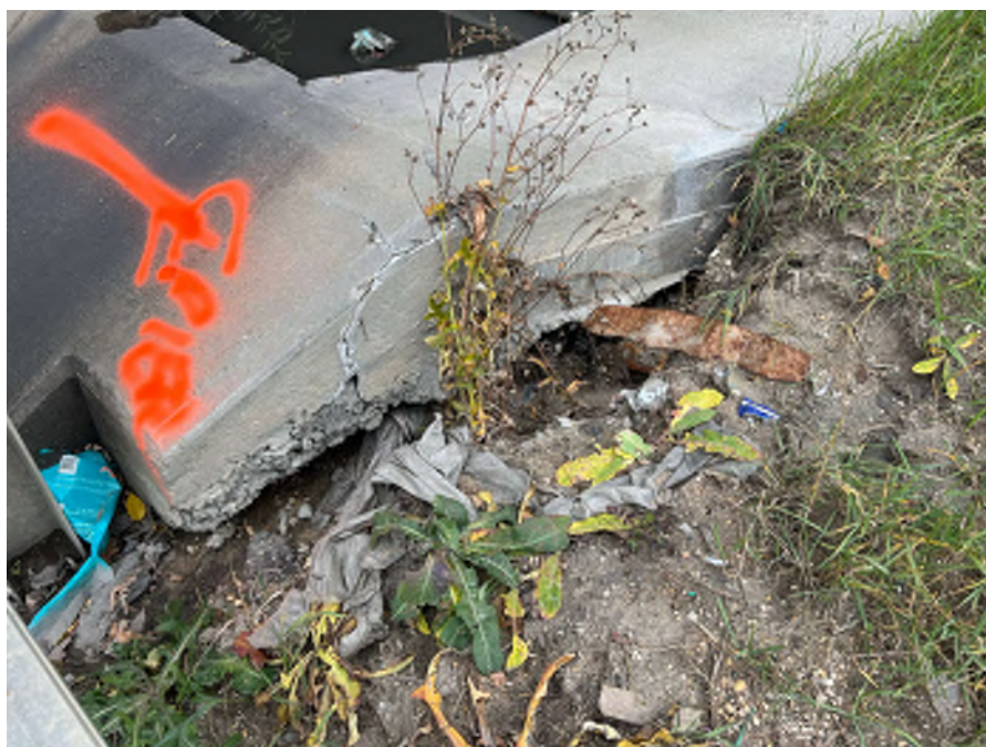
Photo 81 - SW embankment near SU2 pier run off erosion hole
