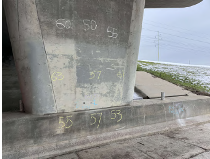
Photo 9 - Typical bottom of pier condition note cracking on barrier wall at base of pier
