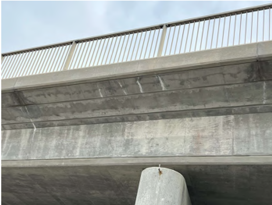
Photo 77 - Typical exterior soffit narrow cracks with efflorescence
