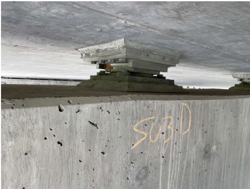
Photo 10 - SU3 Pier, Line 'D' bearing, coating failure on west side of bearing
