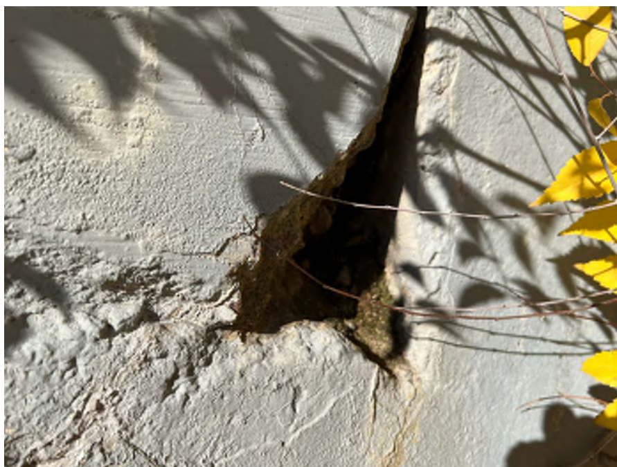
Photo 74 - Spall on corner of NE wingwall
