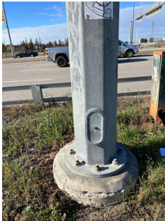
Photo 4 - Overhead sign structure, base plate and foundation
