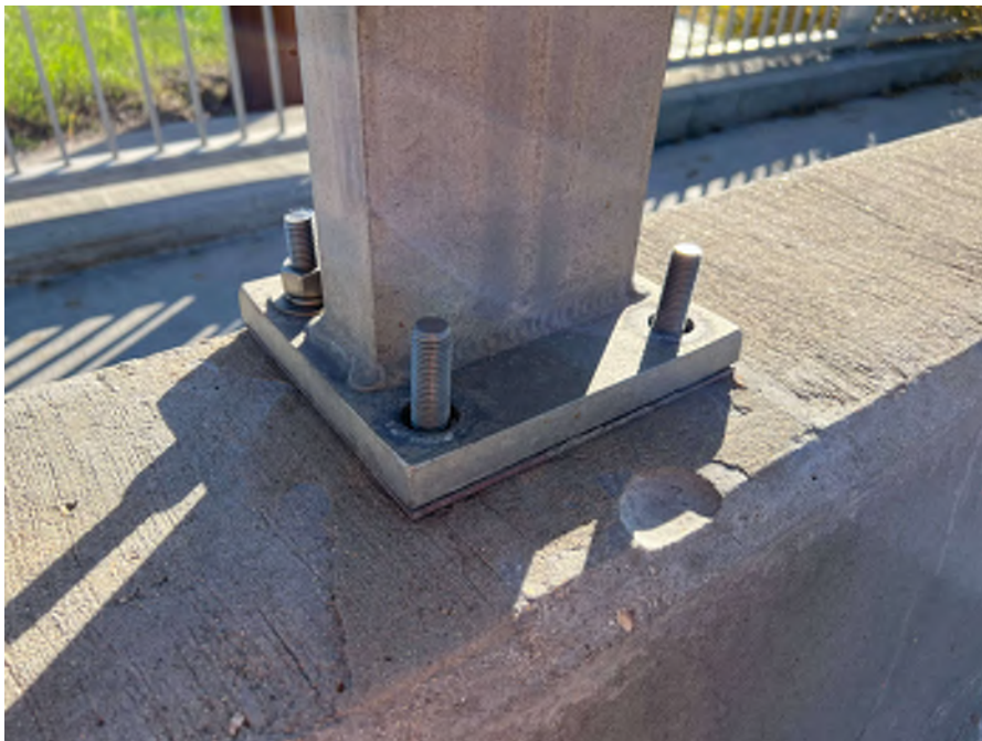
Photo 60 - East traffic barrier rail showing post missing 2 nuts and washers.
