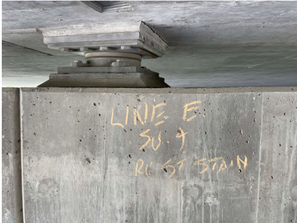
Photo 21 - SU4, Line "E" bearing, minor rust stain
