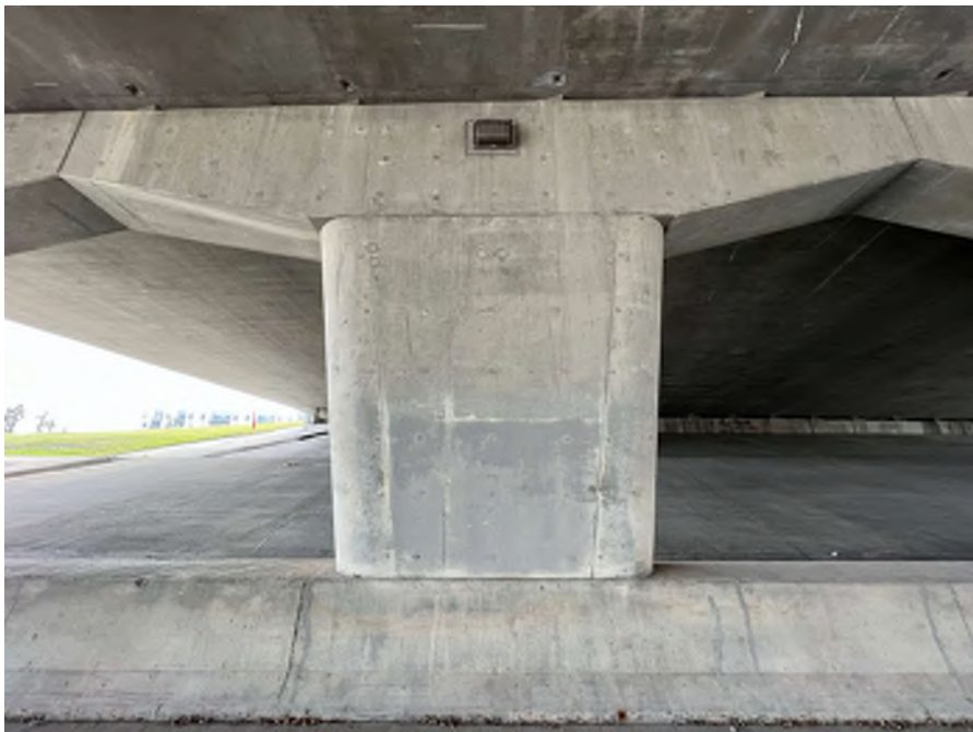
Photo 40 - Typical SU2 pier cap, shaft, and base pedestal
