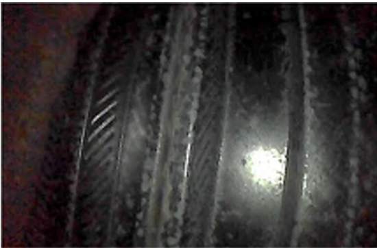
Figure 21: Stay-in-place Deck Forms at P1G1
