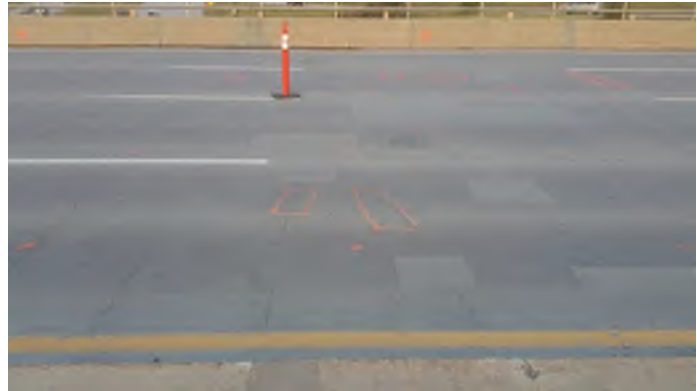
Photo 2.3 – Typical High Concentration of Cracks, Patches and Delamination over Pier Area with Cracks through 2014 Repairs
