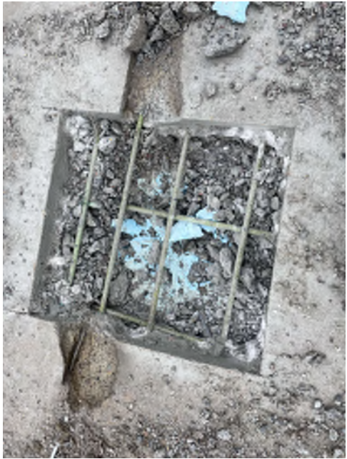
Photo 9 - Median Test Pit 2 - median slab concrete removed, styrofoam partially exposed, longitudinal bar under transverse joint corroded through additional view
