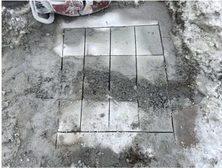
Photo 7 - Median Test Pit 2 - at start of removals, note deterioration at joint location, closer view
