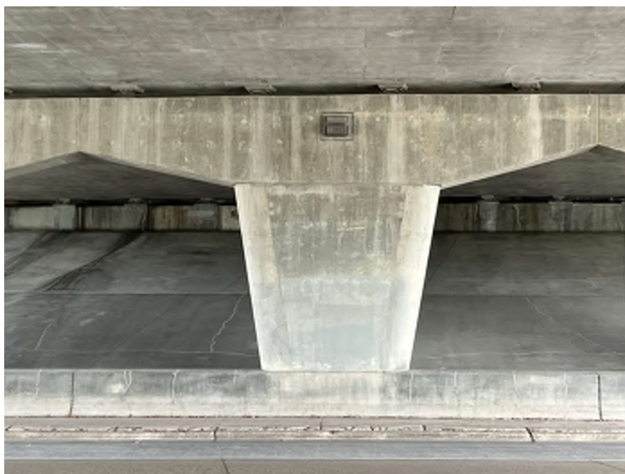
Photo 44 - Typical SU4 pier cap, shaft, and base pedestal
