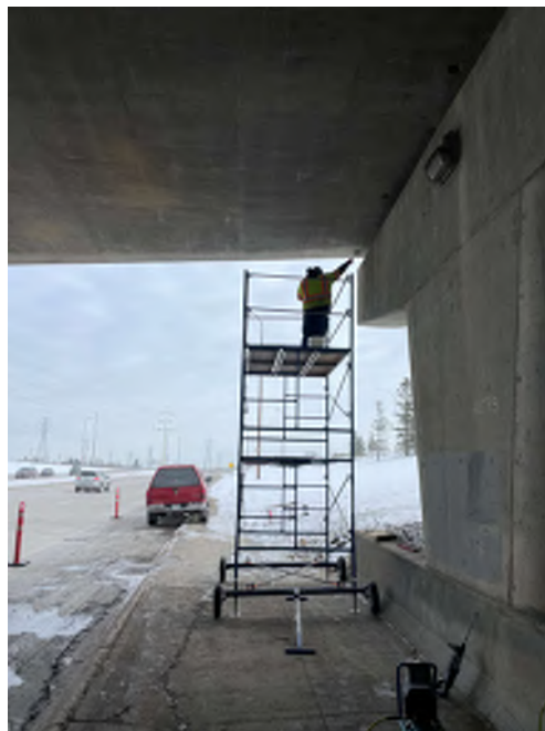
Photo10 - Borescope inspection completed by VCS Engineering Ltd with rolling scaffold for access
