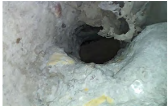
Figure 14: Blocked Drainage Hole at SAG14
