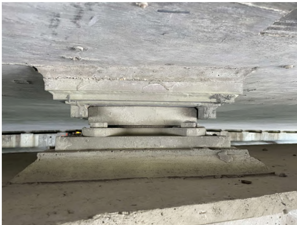
Photo 22 - SU4, Line "K" unidirectional bearing
