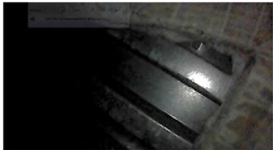
Figure 45: Stay-in-place Deck Forms at NAG1
