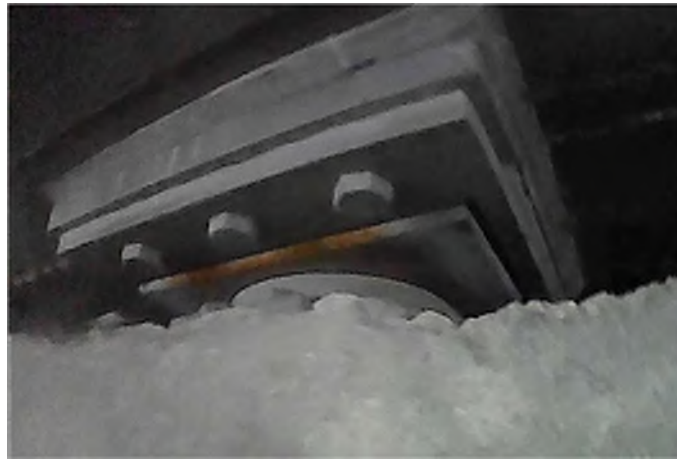
Figure 64: NAG15 Bearing Plate
