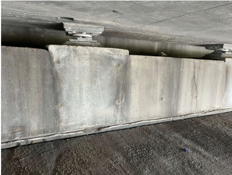
Photo 71 - Abutment wall typical narrow to medium vertical cracks
