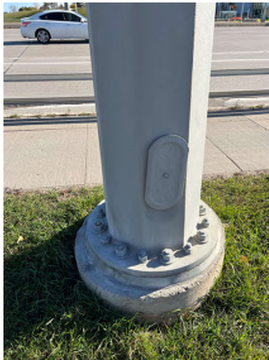
Photo 4 - Overhead sign structure, base plate and foundation
