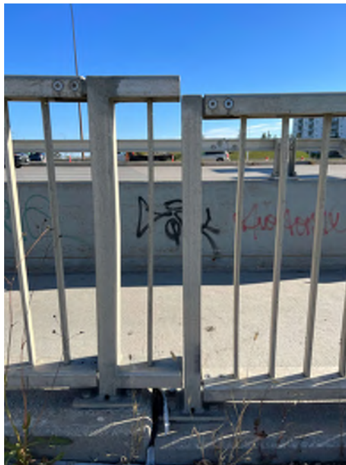
Photo 66 - Pedestrian handrail at SW corner showing differential settlement (~50mm)
