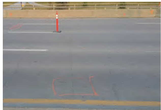
Photo 2.1 – Delamination with Wide Crack in Northbound Lanes
