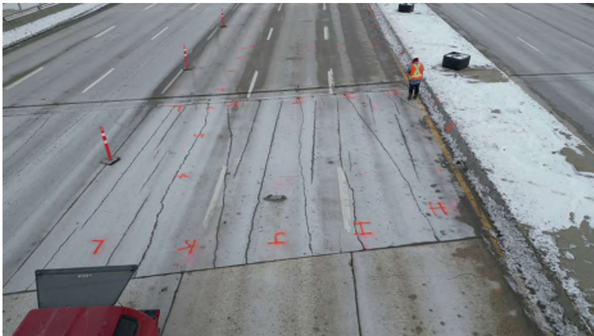
Photo 55 - Typical approach slab medium to wide cracking
