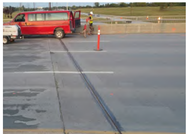
Photo 2.2 – Previous Patch with Map Cracking at North Abutment
