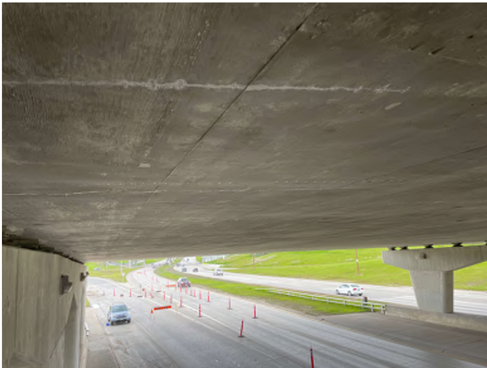
Photo 14 - Span 2, narrow crack with efflorescence near SU2 Pier
