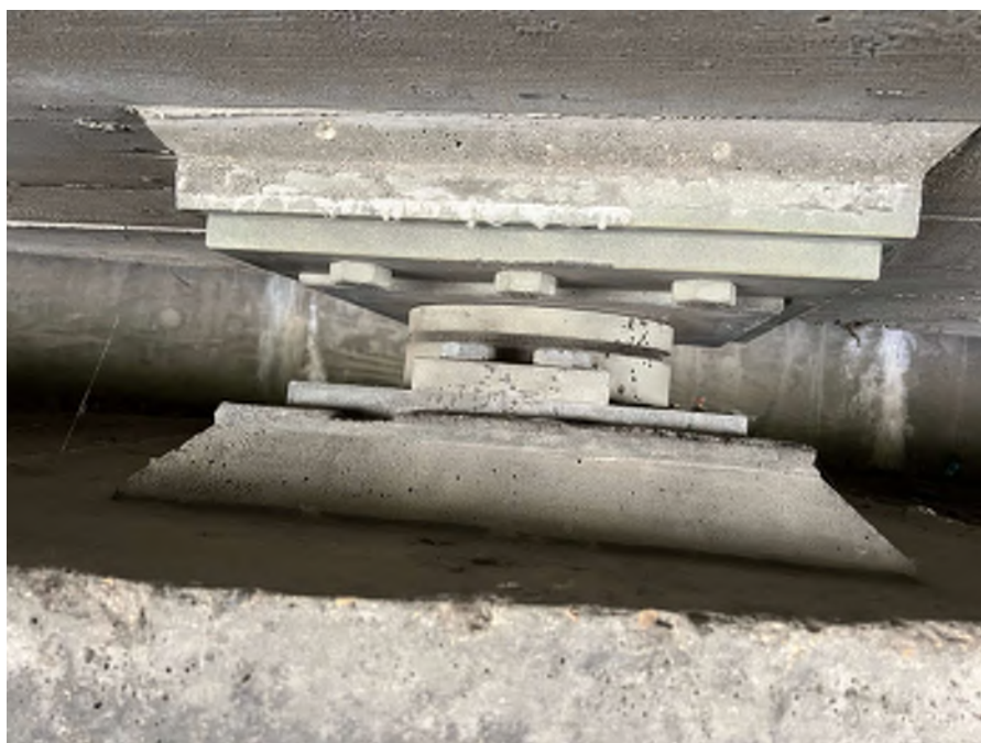
Photo 32 - Typical SU1 abutment bearing
