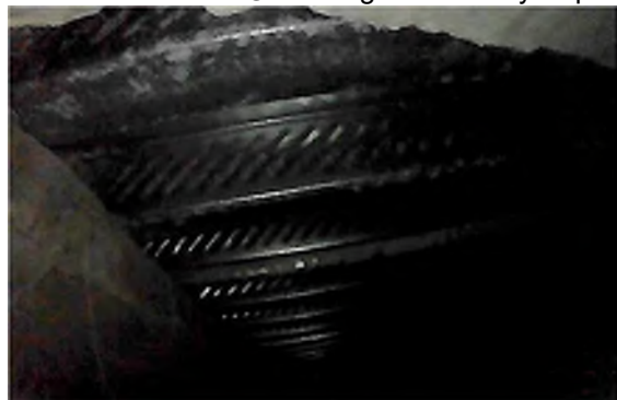
Figure 33: Stay-in-place Deck Forms at P1G13
