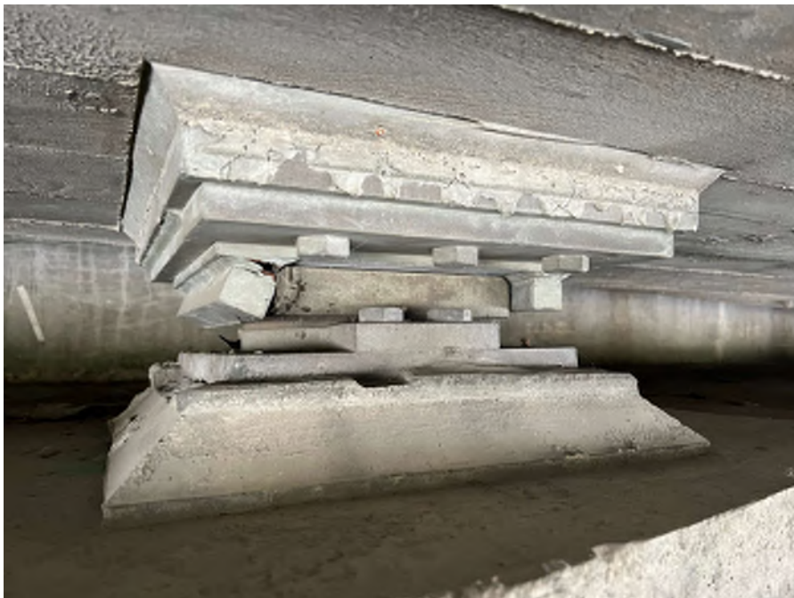
Photo 72 - SU1 abutment bearing 11 from West with cracked bearing plate
