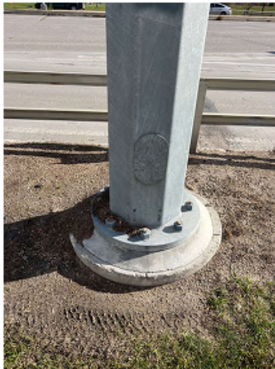
Photo 4 - Overhead sign structure, base plate and foundation
