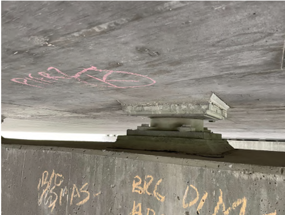
Photo 05 - SU3 Pier, Line "K" bearing near transverse centreline – note- confirmatory measurements taken on bearing
