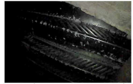
Figure 62: Stay-in-place Deck Forms at NAG19
