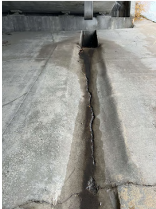
Photo 79 - NE drain gutter typical wide cracking on slope paving
