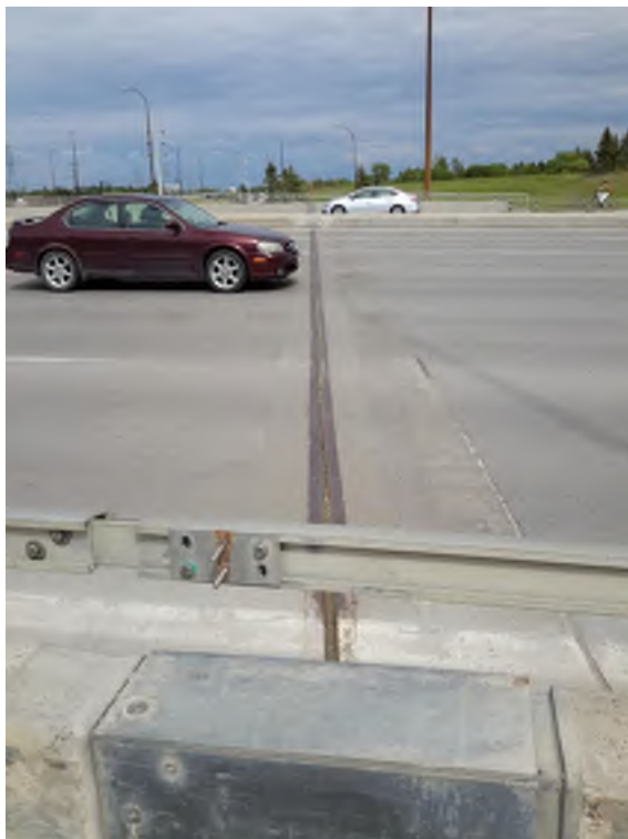
Photo 31 South expansion joint, southbound lanes, very narrow gap. 2017-08-23
