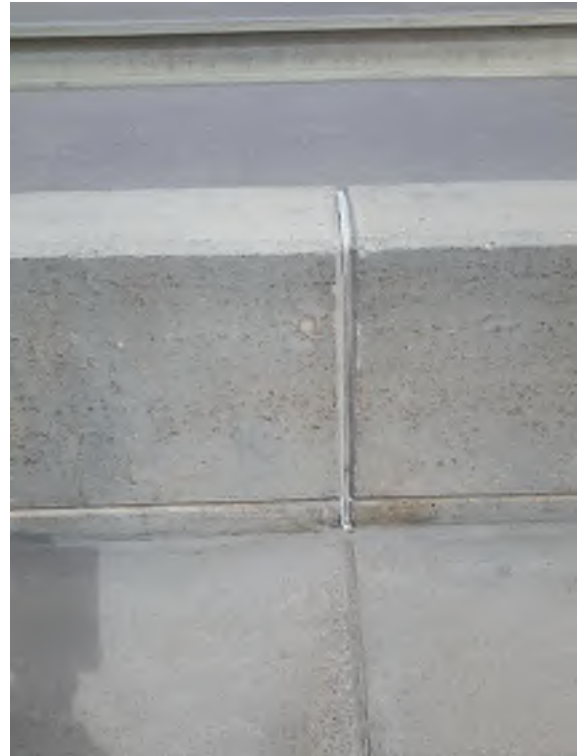
Photo 34 Typical traffic barrier joint.
