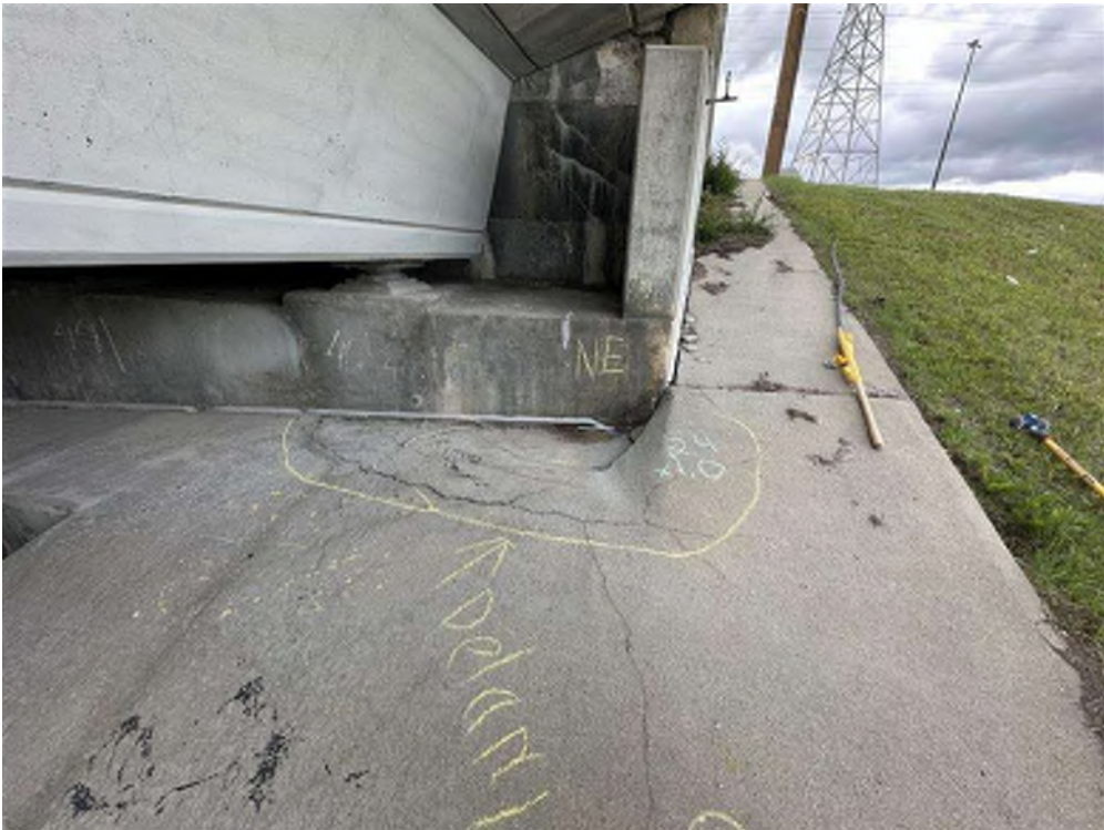
Photo 34 - NE slope paving, delamination 1.0 m x 2.4 m
