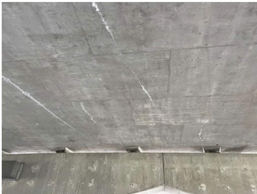
Photo 76 - Typical soffit hairline to narrow cracking with efflorescence near piers
