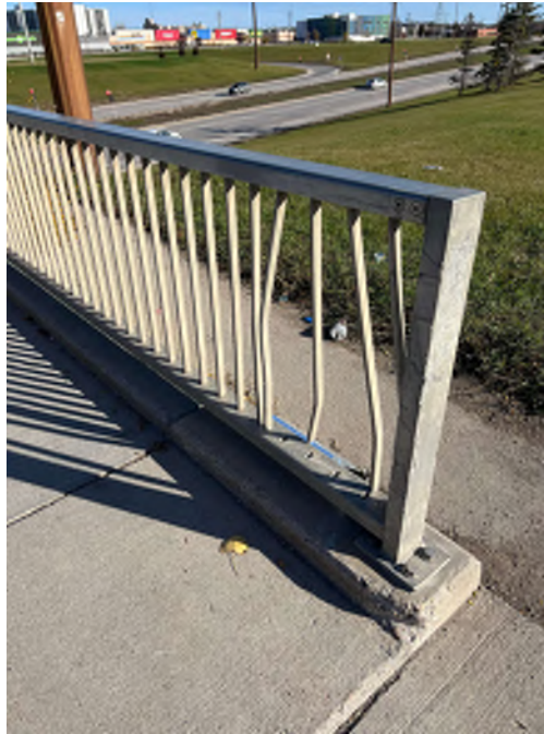
Photo 63 - Pedestrian handrail panel with 4 broken pickets at SE corner
