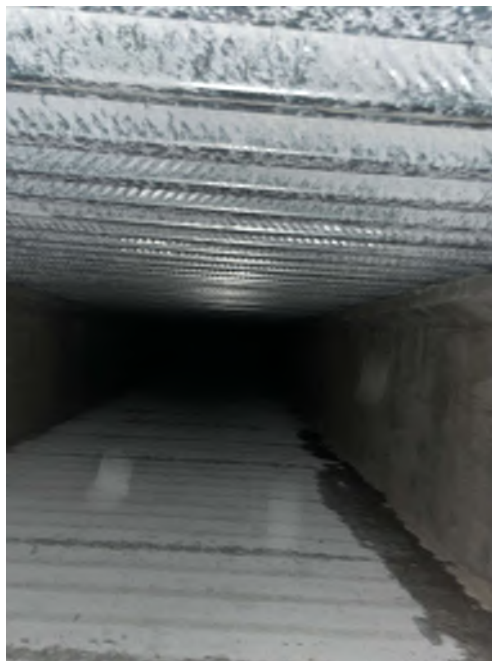
Photo 14 - Deck core hole D29, view inside box girders, note white corrosion oxidation product on SIP formwork
