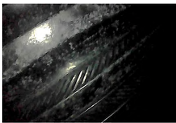
Figure 50: Stay-in-place Deck Forms at NAG6
