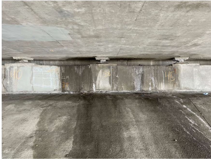
Photo 7 - Abutment wall, intermittment leakage across width of bridge and showing vertical cracking
