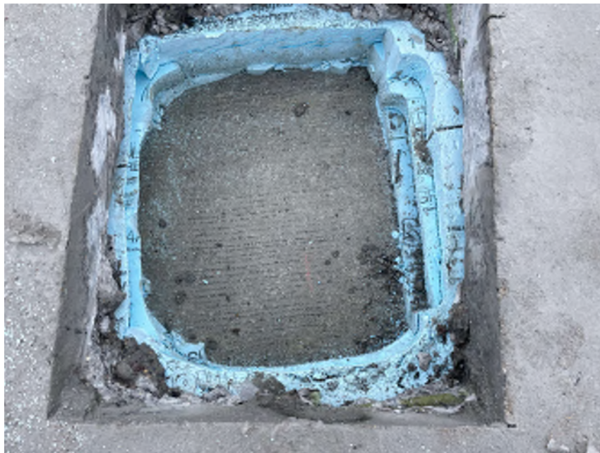
Photo 4 - Median Test Pit 1 - median slab concrete and styrofoam removed, concrete noted to be dry and in good condition
