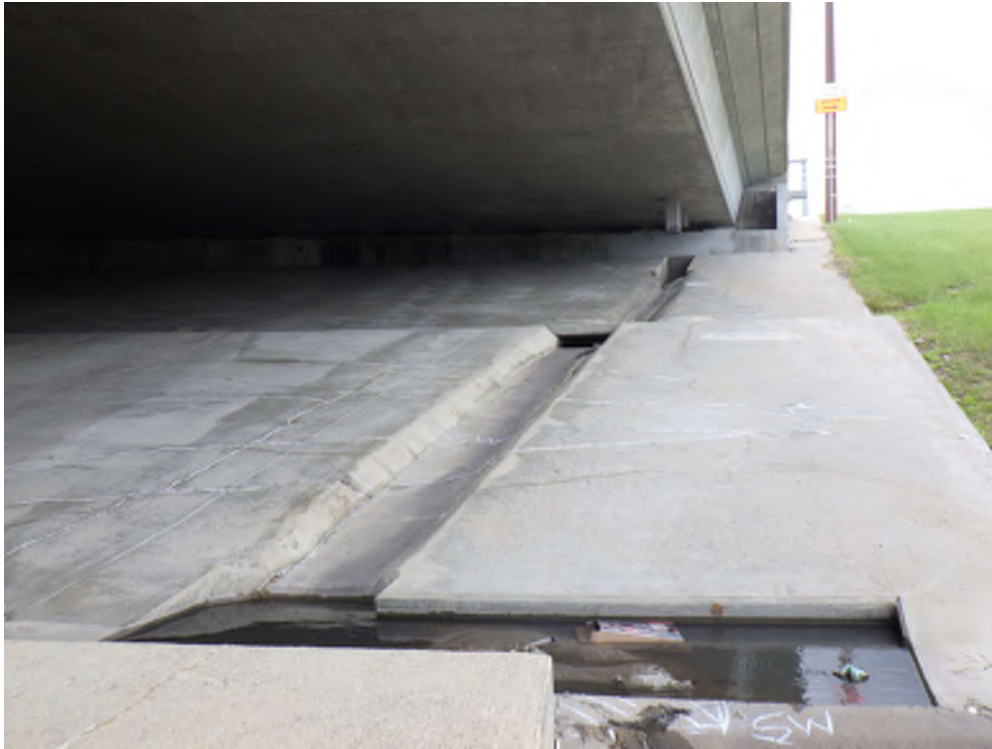
Photo 25 - SW slope paving drainage trough
