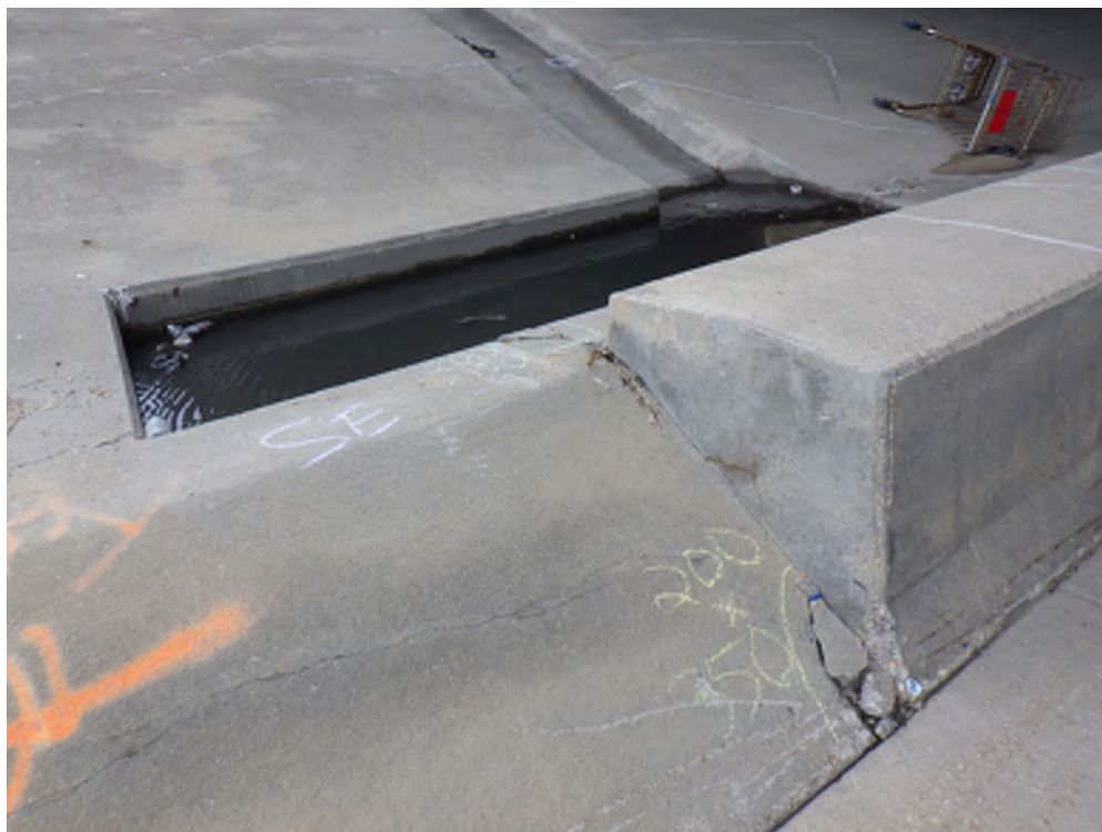
Photo 28 - SE slope paving lower catch basin, small areas of delamination and spalling
