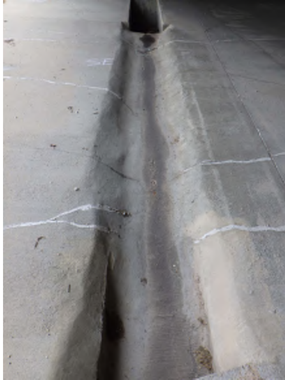
Photo 29 - SE slope paving drainage trough, closer view of wide cracking and localized small delaminations
