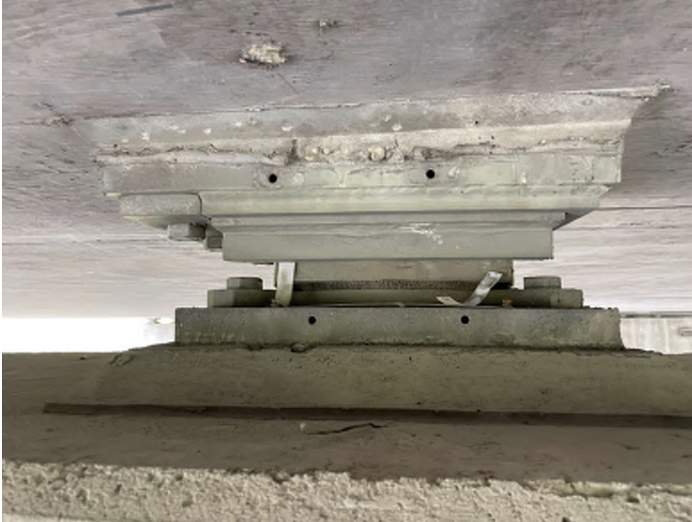
Photo 07 - SU3 Pier, Line "I" bearing, loose Teflon strips on south side, close up view
