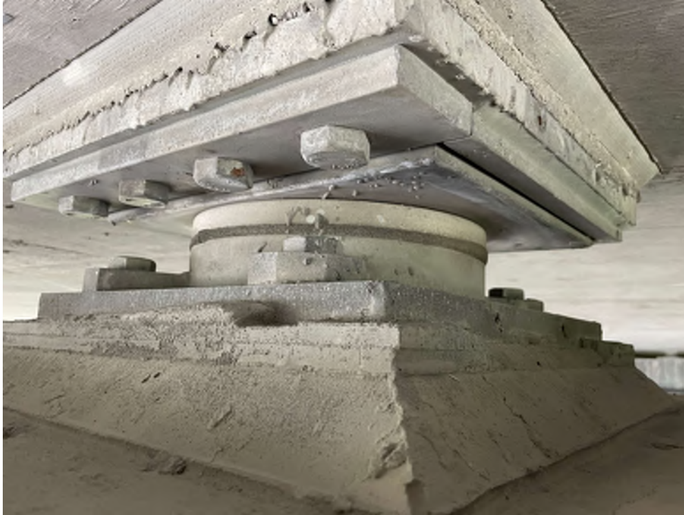
Photo 13 - SU2 Pier, Line "N", coating spatter on sliding plate, closer view
