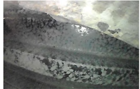
Figure 60: Stay-in-place Deck Forms at NAG17
