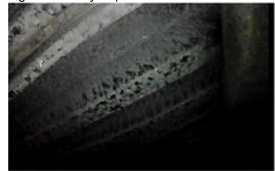
Figure 54: Stay-in-place Deck Forms at NAG11
