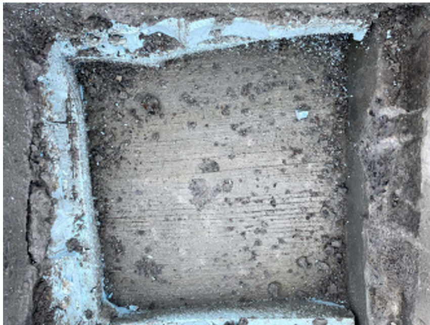
Photo 16 - Median Test Pit 3 - median slab concrete and styrofoam removed, concrete noted to be dry and in good condition, light flaking surface chipping occurred during s
