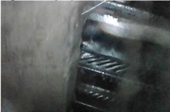
Figure 31: Stay-in-place Deck Forms at P1G11
