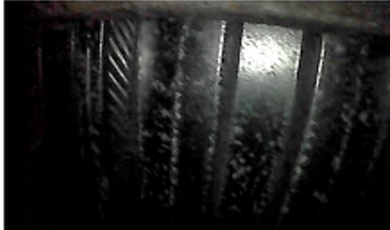
Figure 24: Stay-in-place Deck Forms at P1G4
