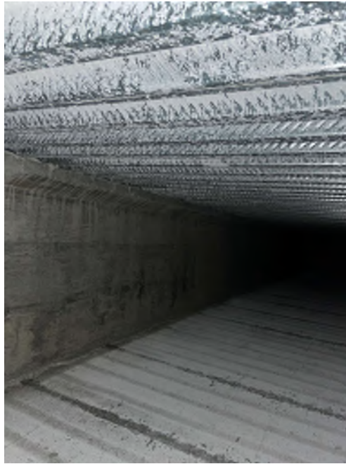
Photo 15 - Deck core hole D29, view inside box girders, girder web and top flange, note dampness and staining
