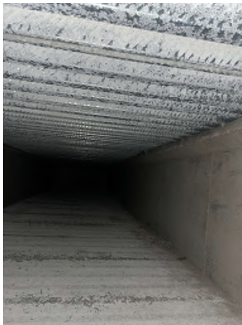
Photo 12 - Deck core hole D12, view inside box girders, note white corrosion oxidation product on SIP formwork, additional view
