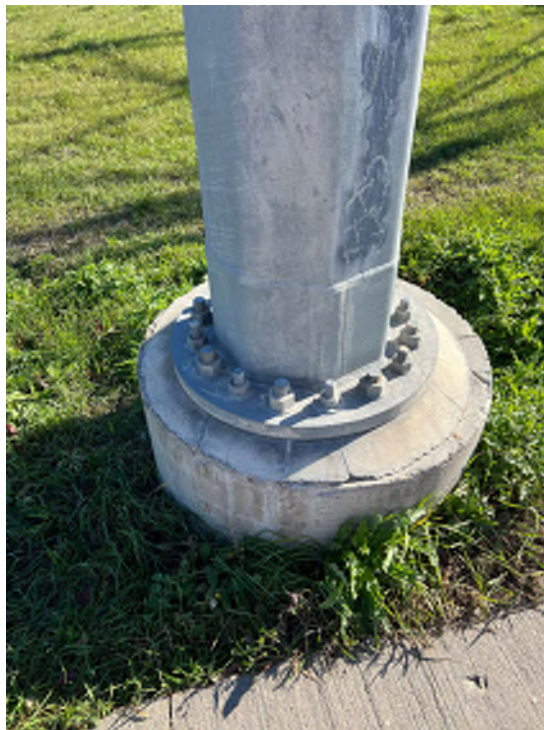
Photo 6 - Narrow cracking on foundation grout pad
