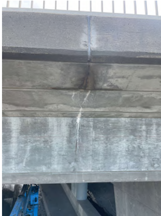
Photo 17 - Deck overhang at sidewalk curb joint near SU2, note wetness and efflorescence
