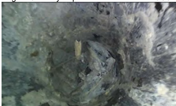
Figure 36: Blocked Drainage Hole at P3G12
