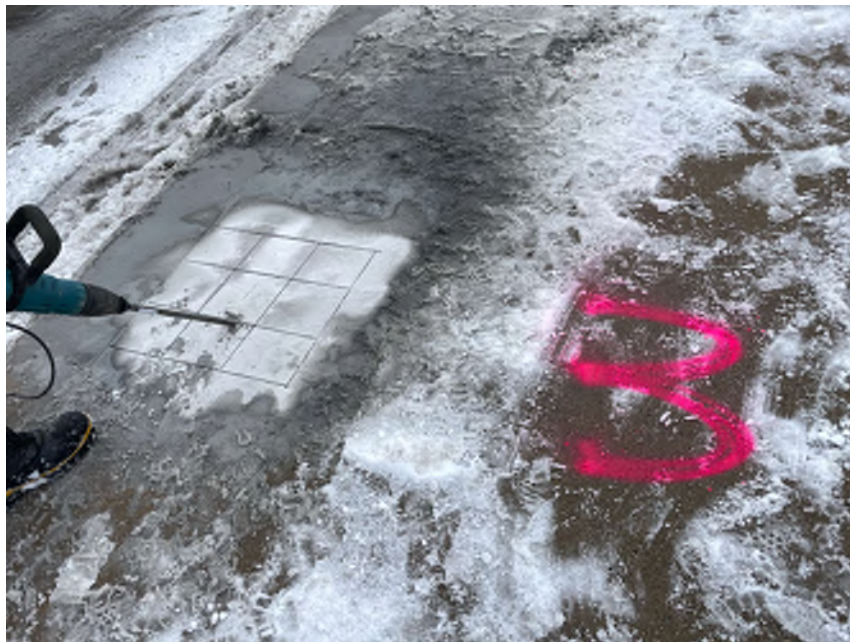
Photo 12 - Median Test Pit 3 - at start of removals
