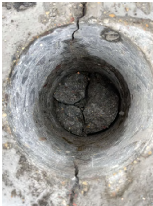
Photo 4 - Approach slab core APP7, taken through a wide longitudinal crack which extended the depth of the core
