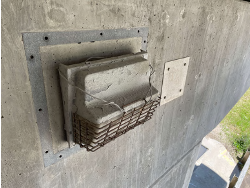
Photo 23 - SU4, light temporarily repaired near east end on south face
