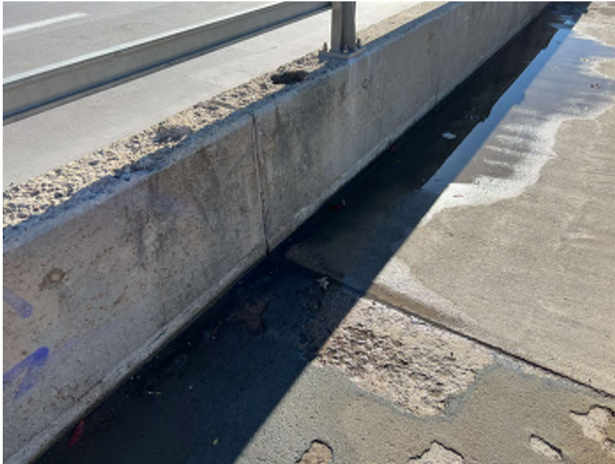
Photo 57 - West barrier and sidewalk area of severe scaling and spalling
