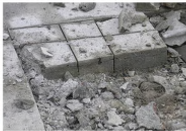
Photo 2.5 – Test Patch with Shallow Delamination
