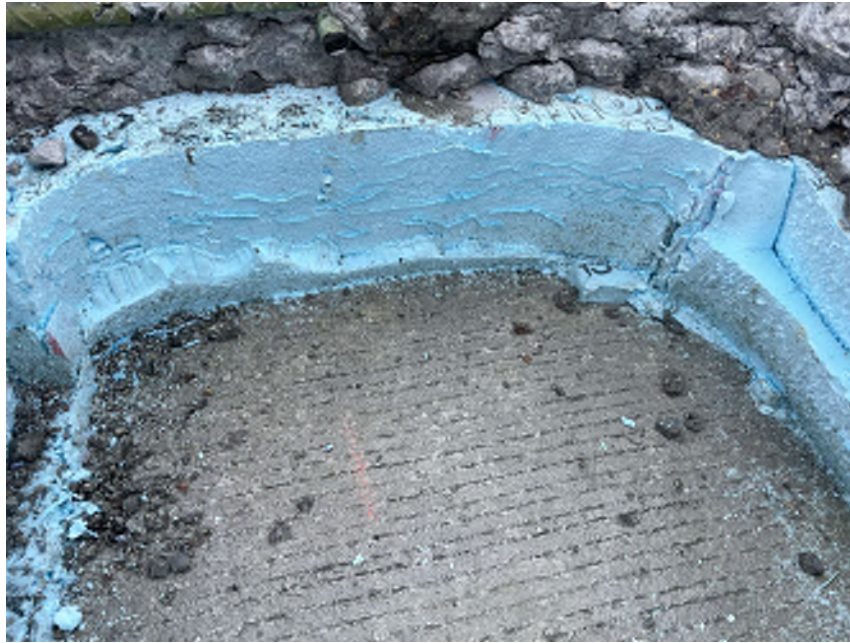
Photo 5 - Median Test Pit 1 - median slab concrete and styrofoam removed, concrete noted to be dry and in good condition, closer view
