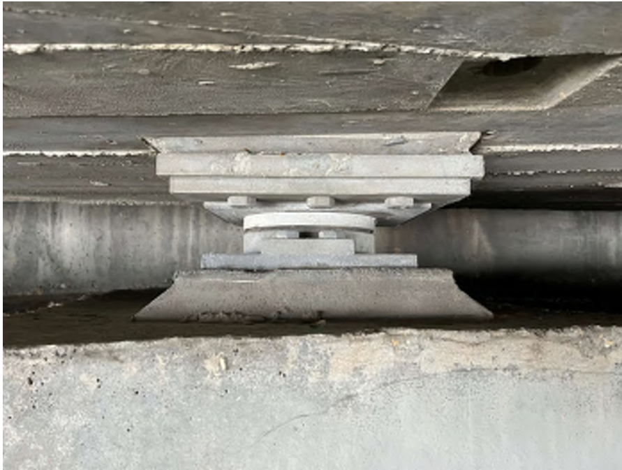
Photo 47 - Typical SU5 abutment bearing
