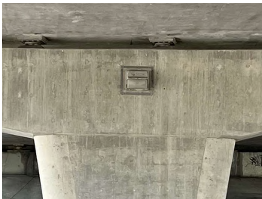
Photo 23 - Typical pier mounted light
