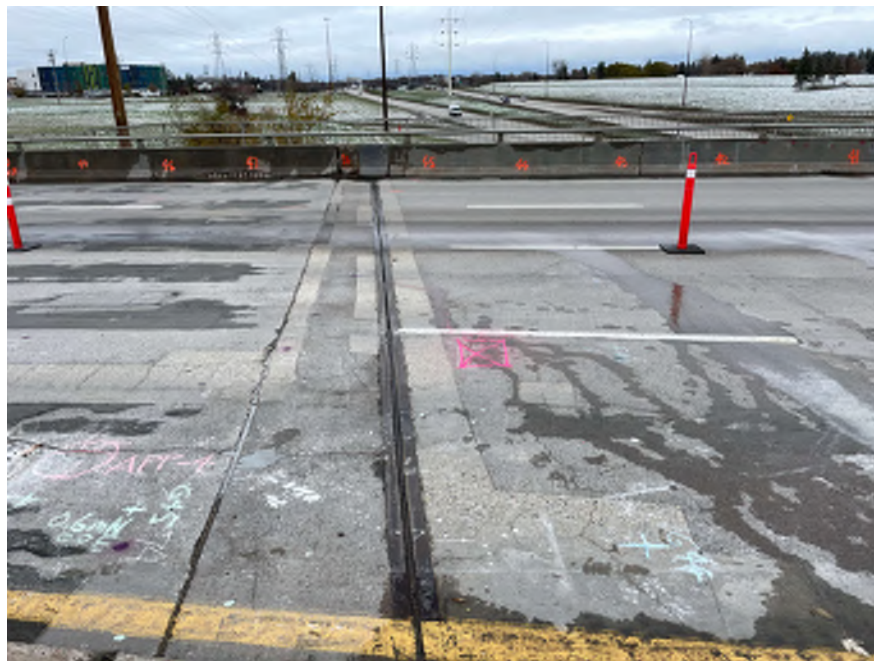
Photo 2 - Typical expansion joint, showing uneven expansion across bridge width
