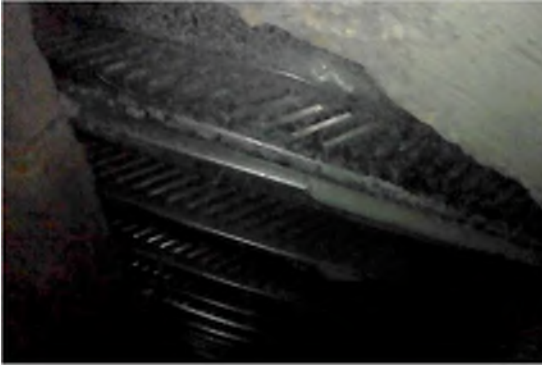
Figure 15: Stay-in-place Deck Forms at SAG15
