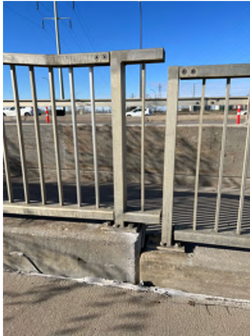
Photo 65 - Pedestrian handrail at NE corner showing differential settlement (~90mm)
