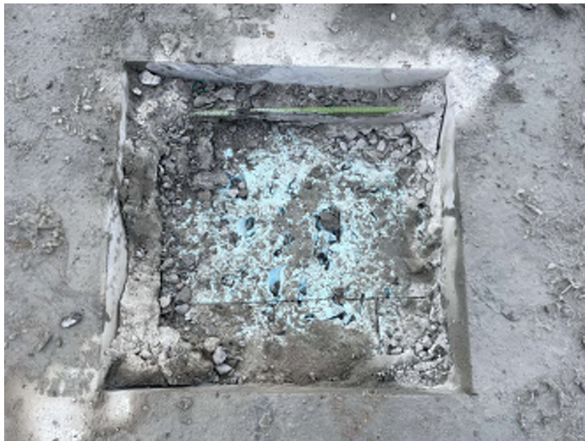
Photo 14 - Median Test Pit 3 - median slab concrete removed, styrofoam exposed
