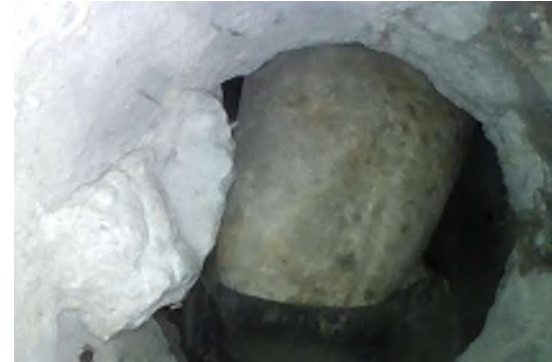
Figure 30: Blocked Drainage Hole at P1G10
