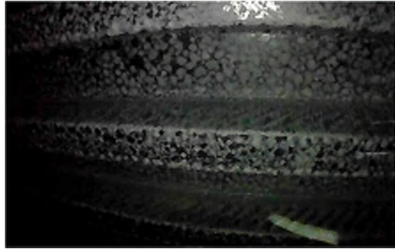
Figure 43: Stay-in-place Deck Forms at P3G19
