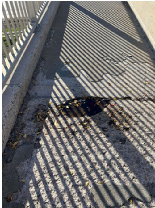
Photo 61 - East sidewalk worn epoxy coating and pothole
