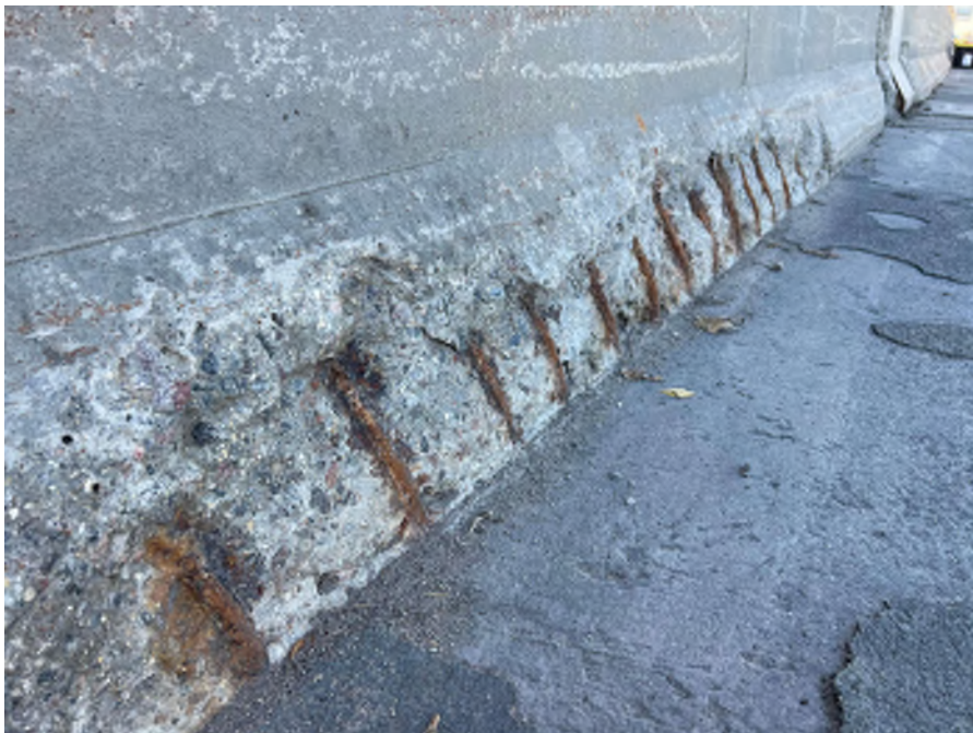
Photo 58 - NE approach barrier, spalls with exposed rebar
