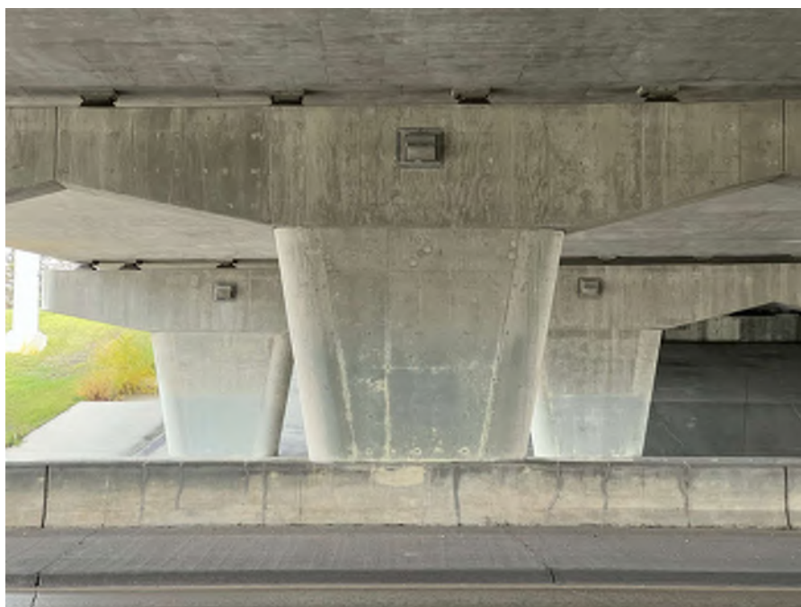
Photo 42 - Typical SU3 pier cap, shaft, and base pedestal
