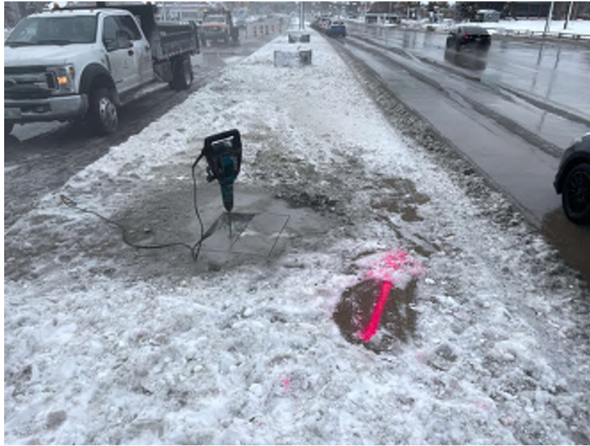
Photo 1 - Median Test Pit 1 - at start of removals
