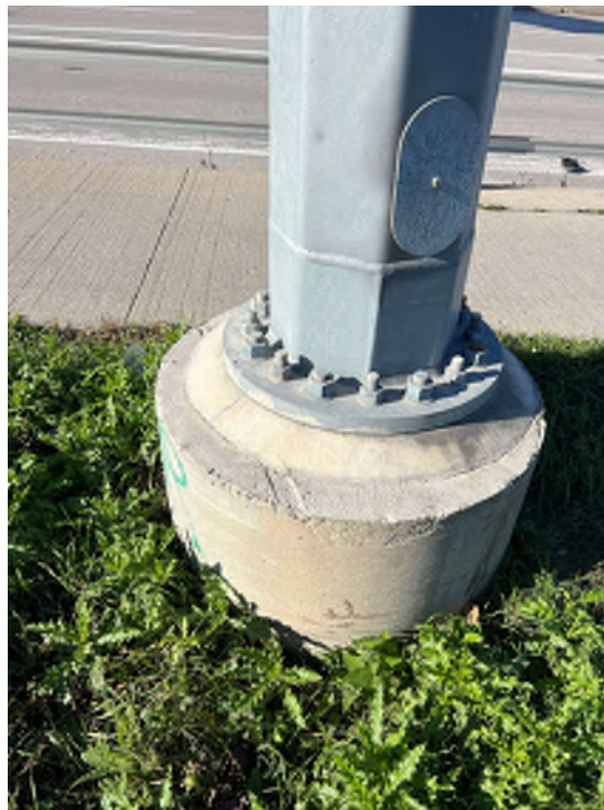
Photo 4 - Overhead sign structure, base plate and foundation
