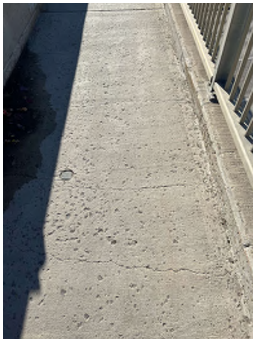
Photo 62 - West sidewalk hairline to medium transverse cracks
