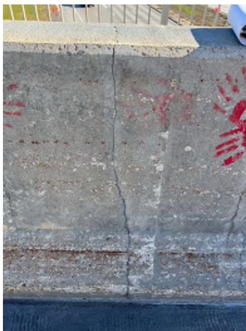
Photo 56 - Typical vertical narrow to medium cracking on traffic barrier inside face
