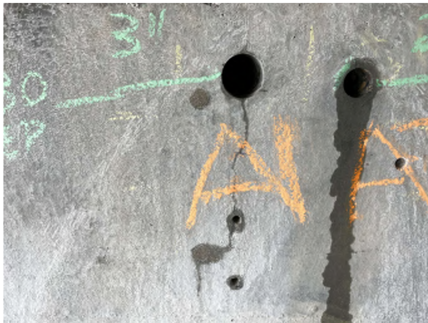
Photo 8 - Abutment core A1, core taken through narrow to medium crack
