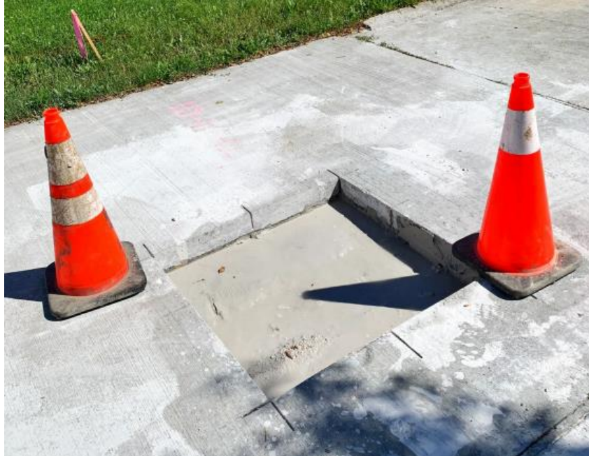
TH24-01 – Sawcut Concrete at Testhole Location
