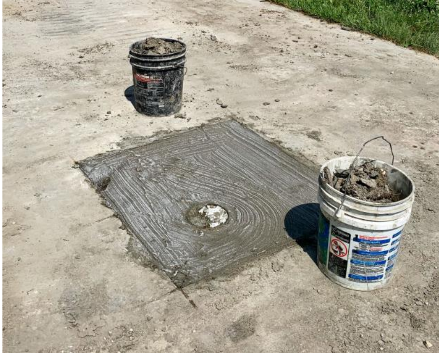
TH24-01 – Grouted with Flush Mount Standpipe Piezometer Installed
