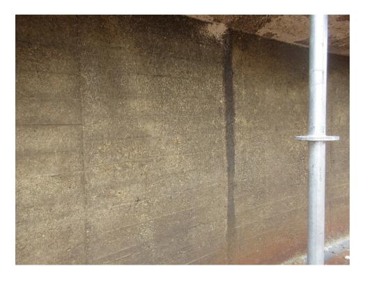
Photo 5: Repaired crack in wall of clarifier
