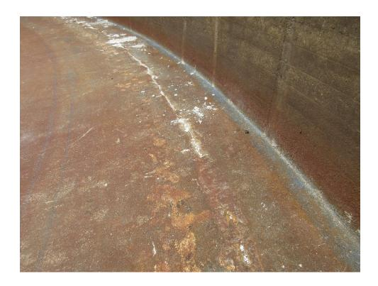
Photo 8: Crack in base slab of clarifier parallel to perimeter of tank
