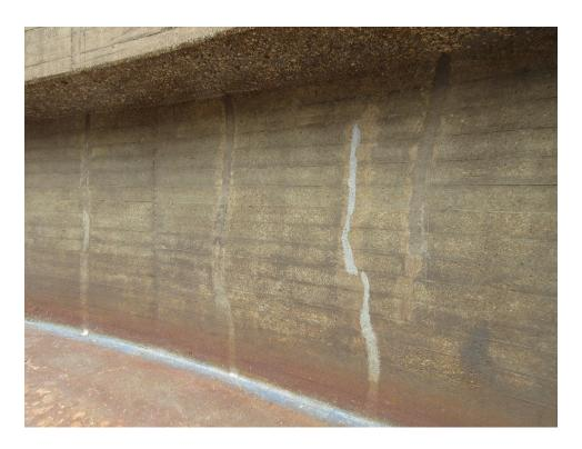
Photo 7: Signs of repaired cracks in wall of clarifier
