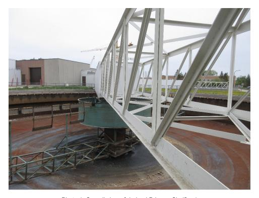
Photo 1: Overall view of drained Primary Clarifier 1
