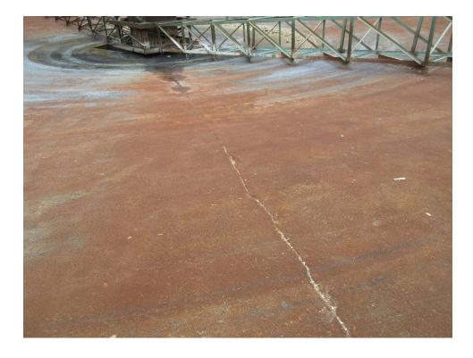
Photo 9: Crack in base slab of clarifier extending from center to exterior wall
