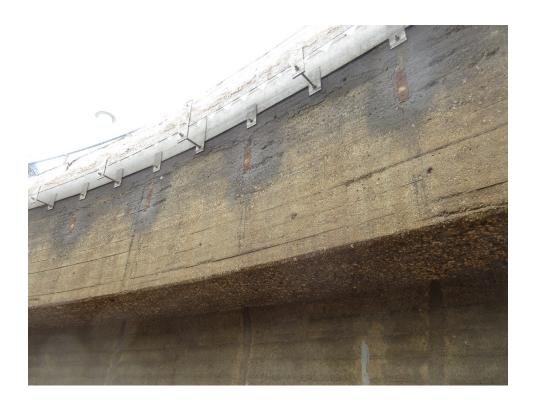
Photo 6: Corroded connection brackets in the side of launder
