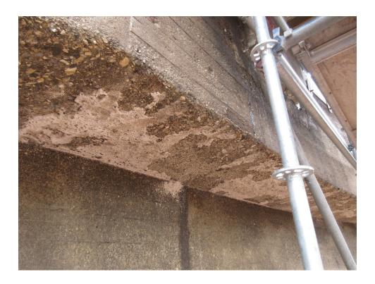
Photo 4: Eroded concrete at underside of launder
