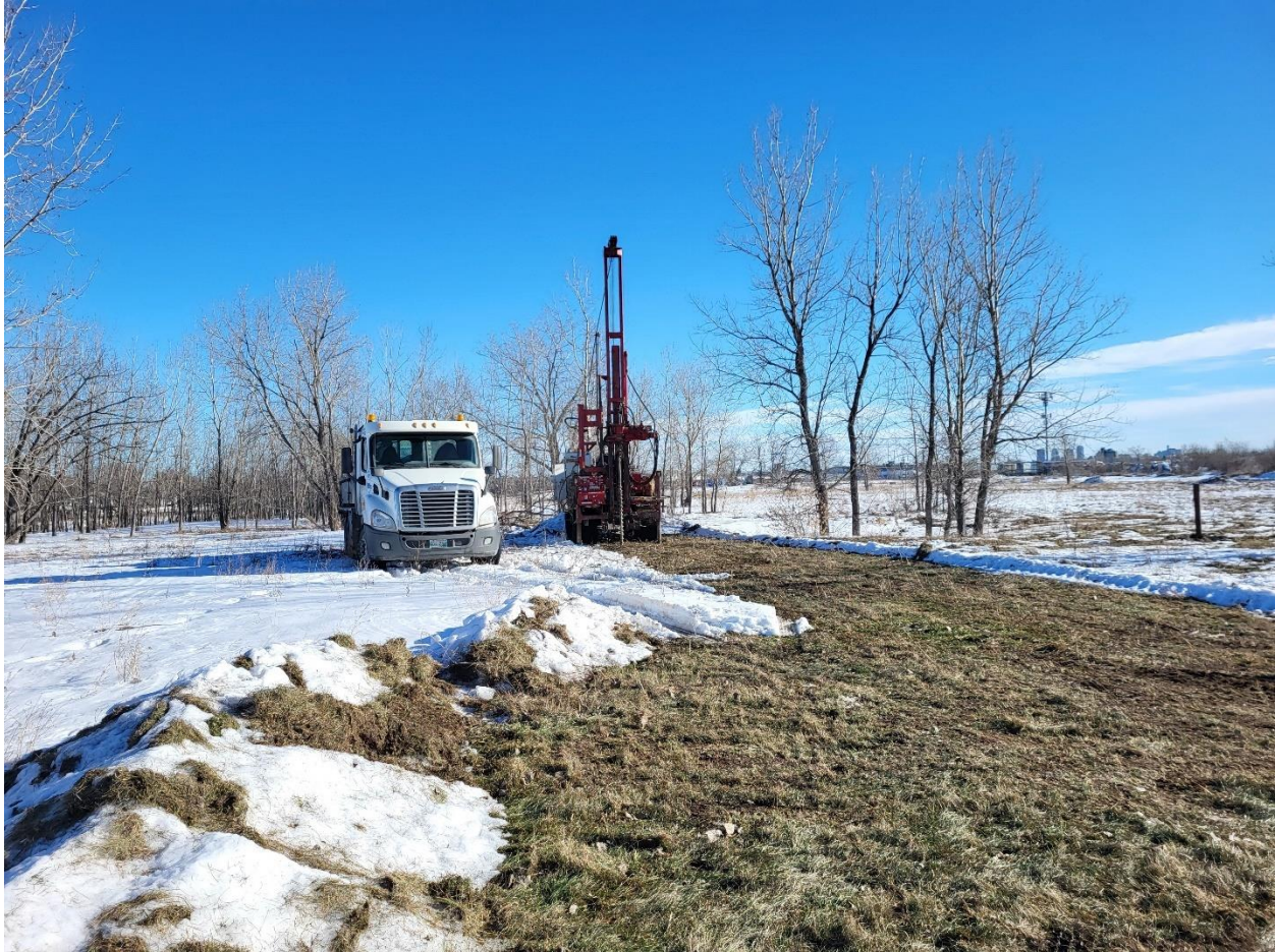
Figure 5 - Solid Stem Auger for TH24-12
