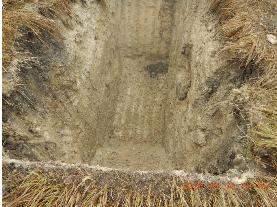
TP24-05 Photo 1: Top of bedrock encountered at 3.5 m
