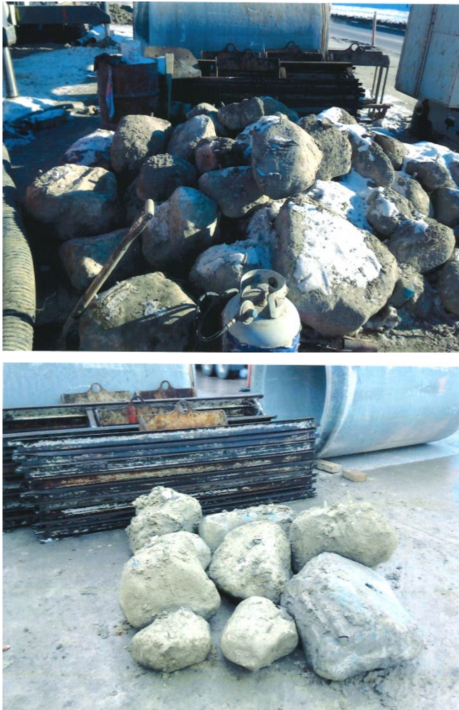
FIGURE 5-1: BOULDERS REMOVED DURING TUNNELLING FOR THE NW INTERCEPTOR SEWER PROJECT (2015)
