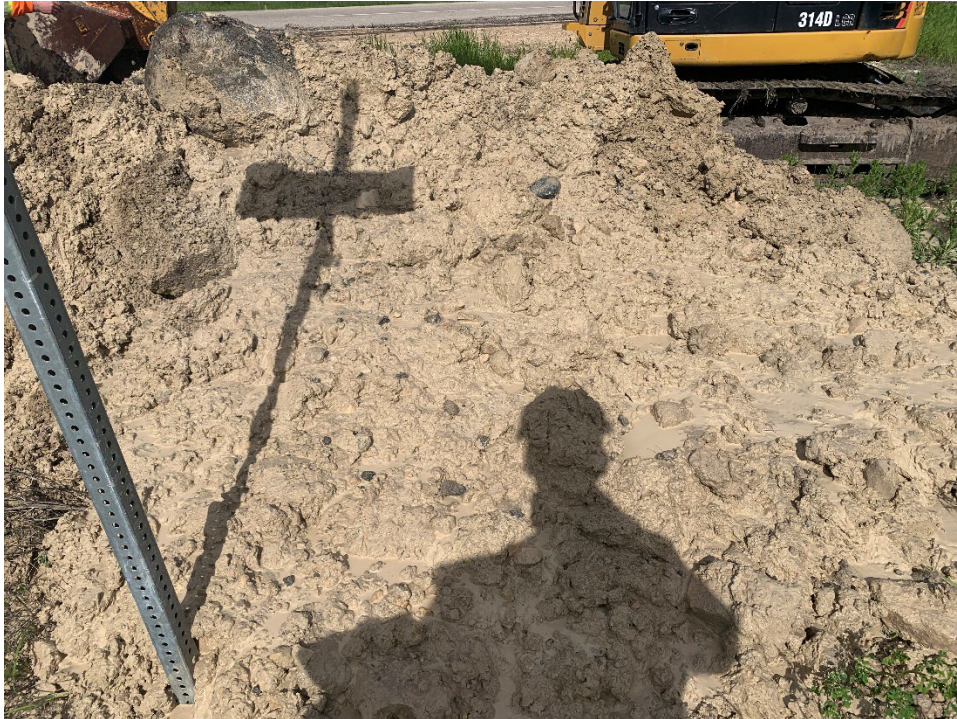
TP24-06 (North) Photo 3: Overview of saturate silt till excavated (after pit base blowout)
