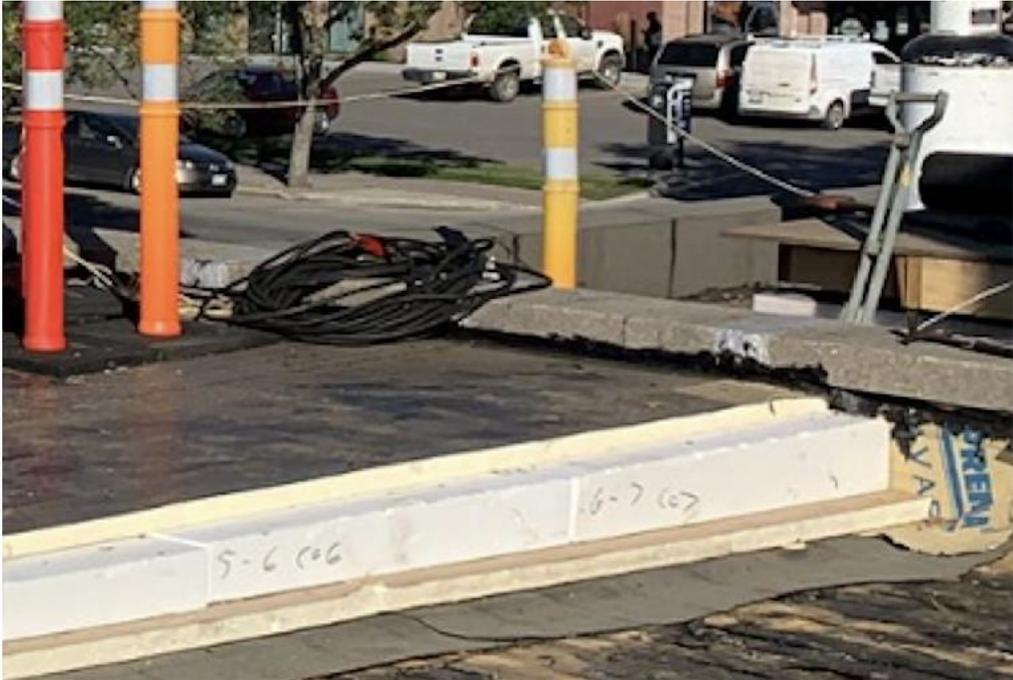
Example of past Firehall with above intended R-value. Two layers of 2" ISO with Type 2 tapered EPS.
