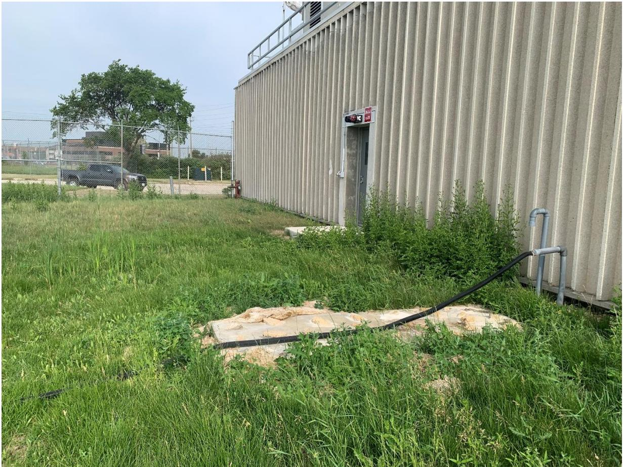
*Figure 2: Existing sump discharge swale to be removed – looking west.*
