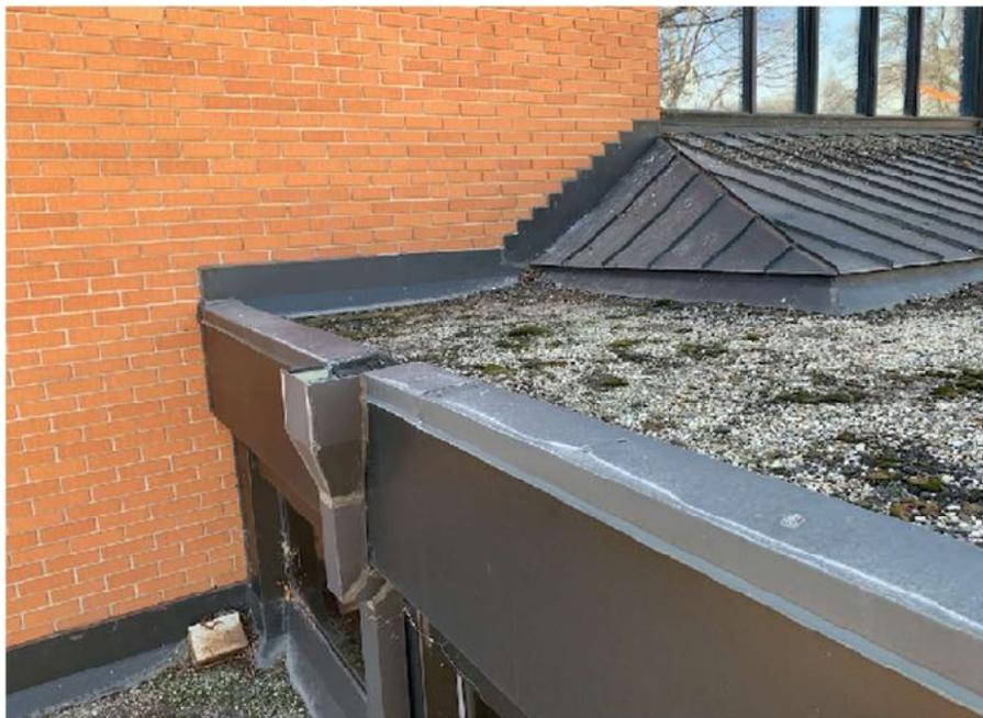
Fig. 12: Roof-C: Modify & seal new reglet flashing(s) as required. Roof thickness not to exceed freeboard of metal roof curb clearance. Re-slope parapet tops min. 2% back to roof.
