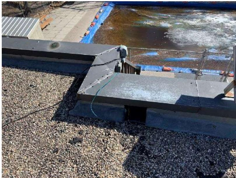
Fig. 8: Roof-A: Exterior electrical by City of Winnipeg. Parapet tops to be re-sloped back to roof a min. of 2%.
