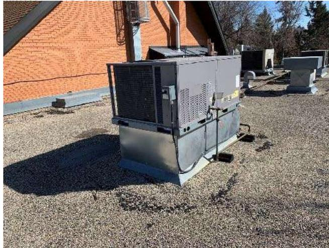
Fig. 5: Roof-A: Remove capped curbs & infill decking as required. Raise & reset mechanical as required.
