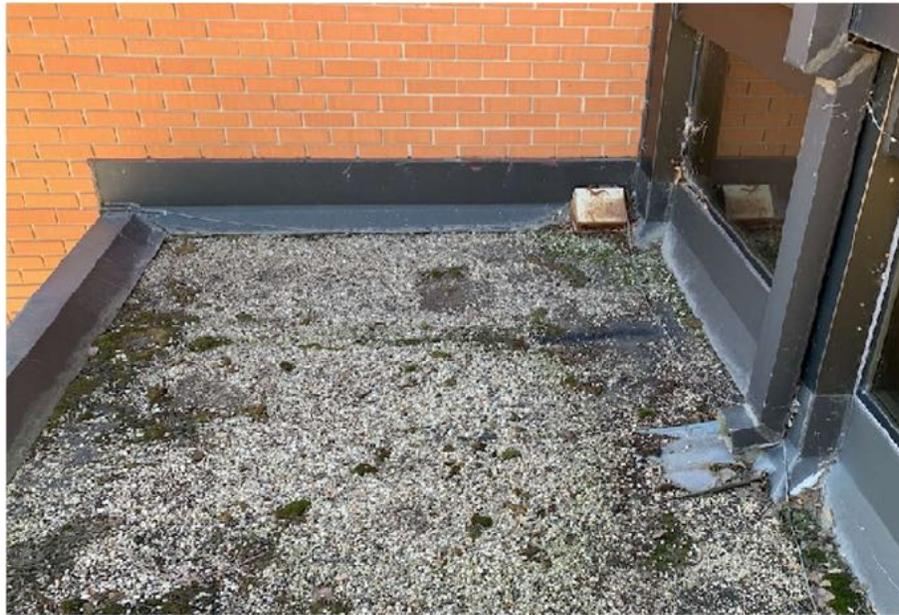
Fig. 11: Roof-B: Save splash pans for re-use. Modify & seal new reglet flashing(s) as required.
