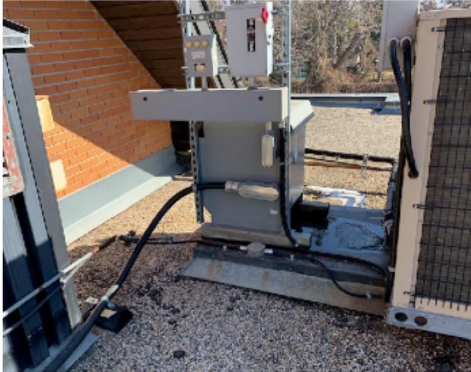
Fig. 7: Roof-A: Modify & raise platform curb including electrical & mechanical to facilitate min. 8 above new roof height.
