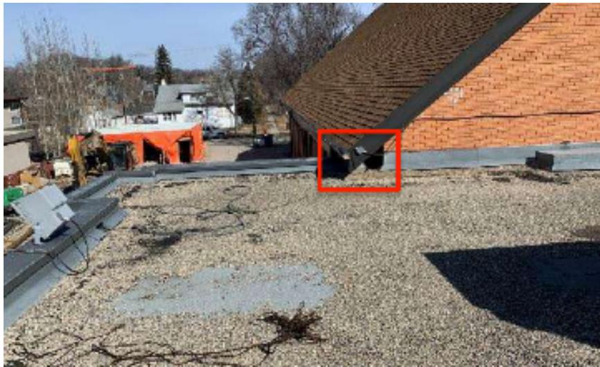
Fig. 4: Roof-A east end disengage flashing & trough and save for re-use; alterations required to facilitate new SBS roof assembly. Provide all required new waterproofing & counter-flashings to seal transition from steep-slope to low-slope. Box-out, insulate & sheath 1/2" plywood at minimum as required to provide support for SBS up-stands. Supply & install new apron flashing at coping to fascia.
