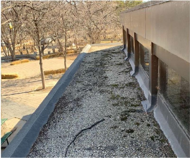
Fig. 10: B: New roof thickness not to exceed glazing threshold clearances. Re-slope parapet tops min. 2% back to roof.
