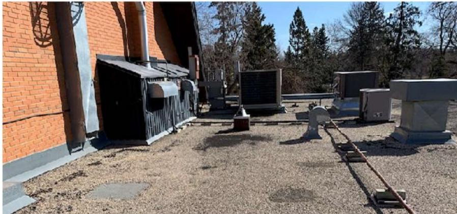
Fig. 6:Roof-A:Renovate ladder length & mechanical doghouse siding as required to facilitate new roof height(s). Paint gas line & provide new gas line blocking to code.
