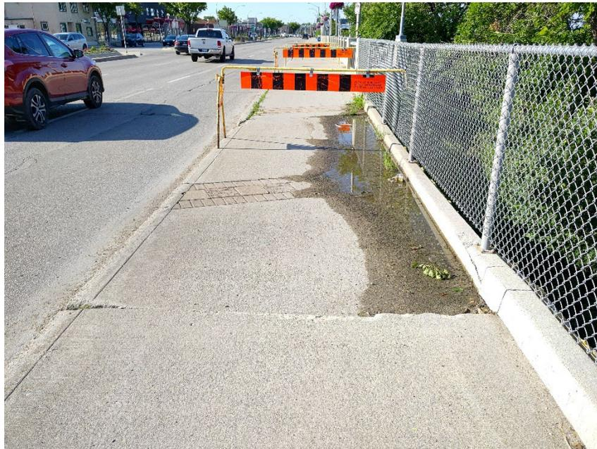
Photo 14: Water collecting at a settled slab (looking south)
