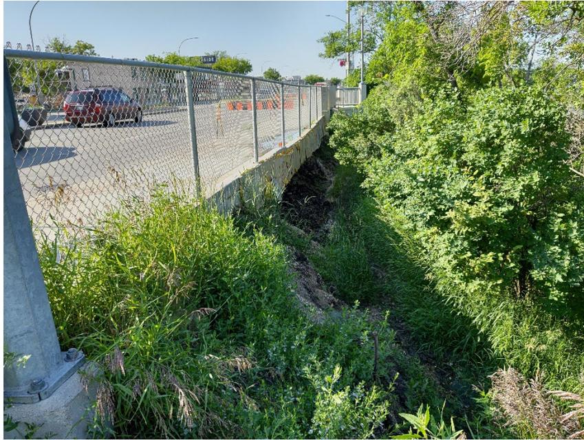
Photo 3: Section of undermined sidewalk foundation (looking southeast)
