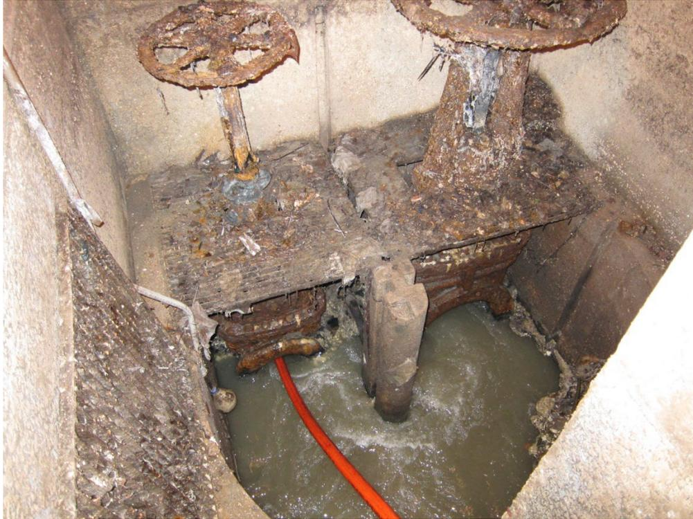
**Figure 11 -Upstream siphon inlets, 300 mm siphon on left (to be lined), 450 mm siphon on right.**
