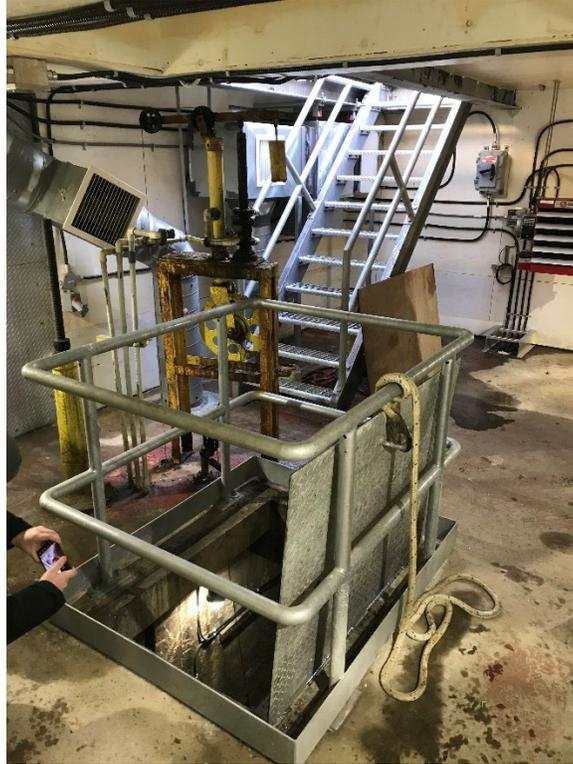
**Figure 3 – Downstream siphon chamber at intermediate floor level. Stair access and access hole in intermediate floor.**
