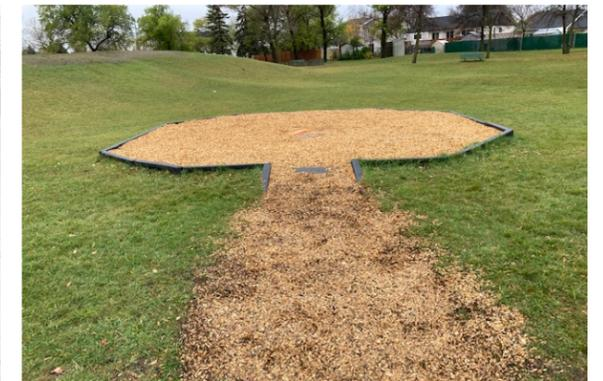
PHOTO B: Safety Surface, Footing and Plastic Edging to be Removed
