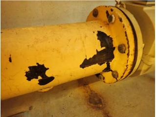
Photo 1. Paint Sample S-01 location (beige piping system; RAS 1; composite sample).
