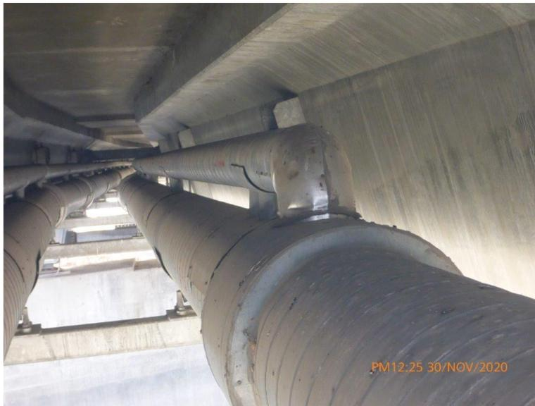
**Site 2 – Air release connection at mid span of bridge, looking west.**
