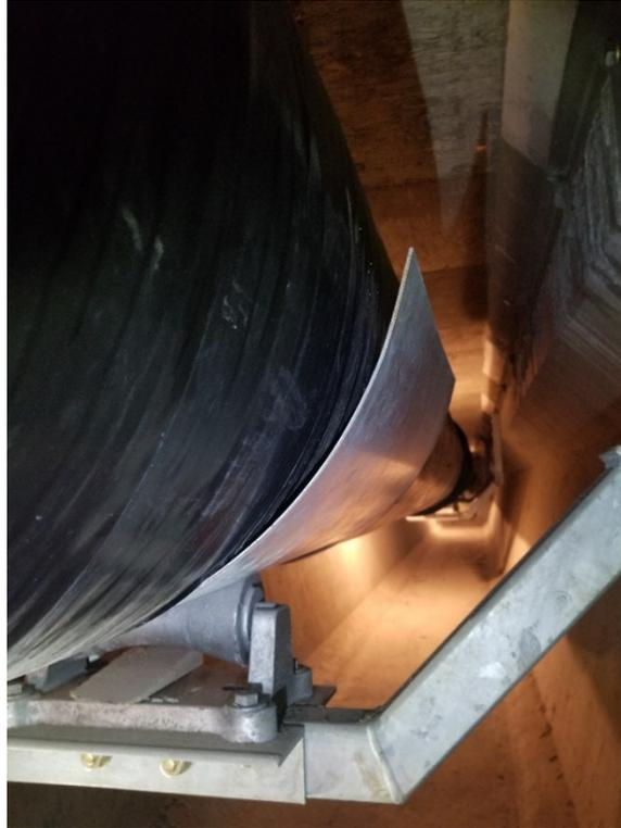
**Site 1 – Typical roller support and weight distribution plate.**
