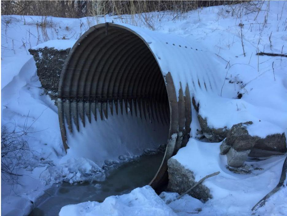
Photo 3: Close-up of outfall showing invert above the winter ice level.
