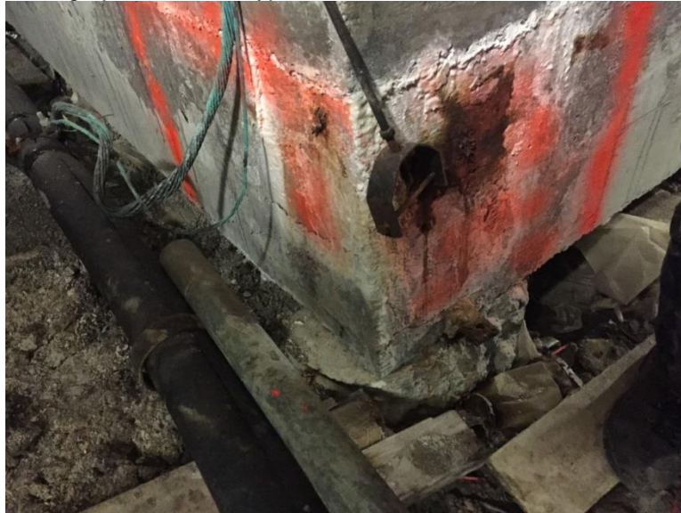
Photograph 3.2.2.1-3: Typical concrete deterioration.
