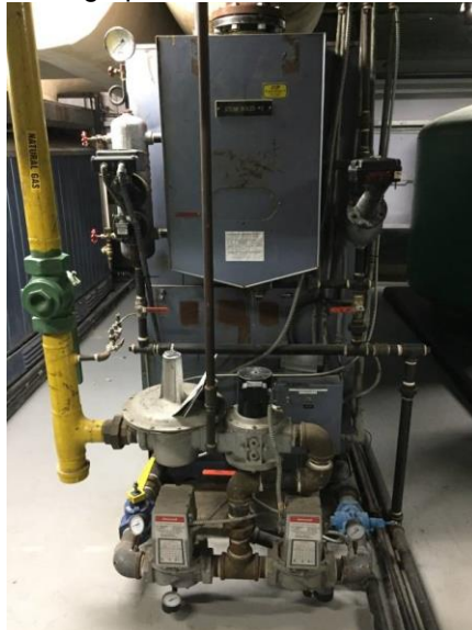
Photograph 2.5.1-1: One of two low pressure steam boilers
