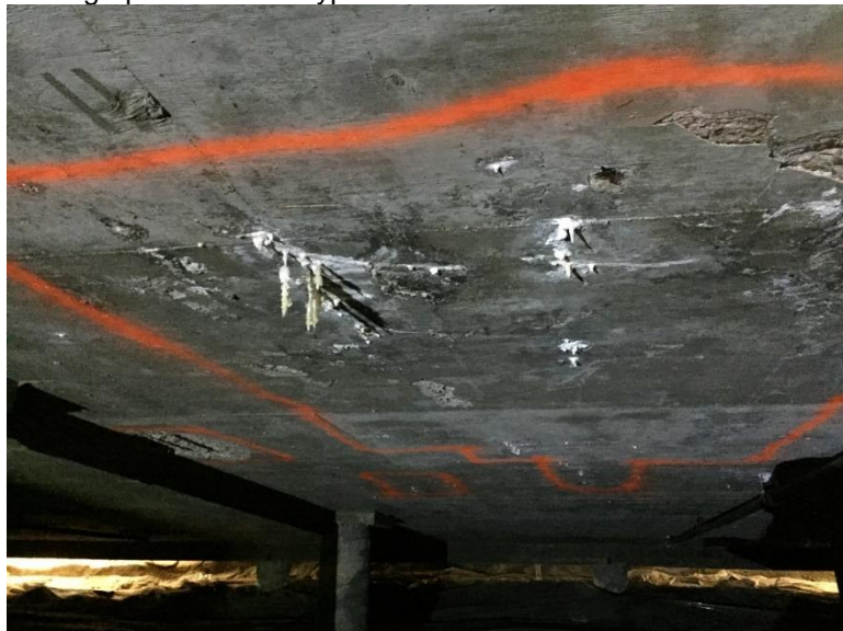
Photograph 3.2.2.1-2: Typical concrete deterioration.
