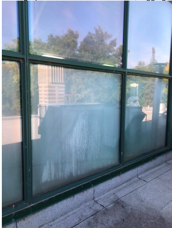
Photograph 3.4.1.2-2: Condensation, fogging of pool north side windows
