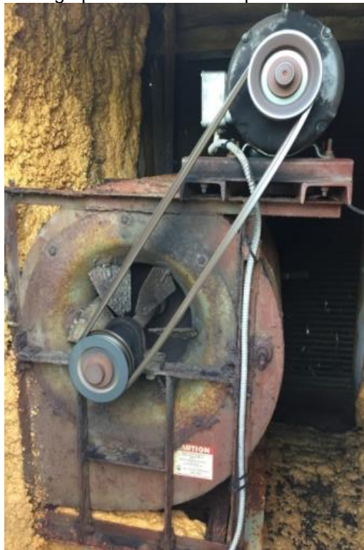
Photograph 3.4.1.1-1 Rooftop HRV Fan deterioration
