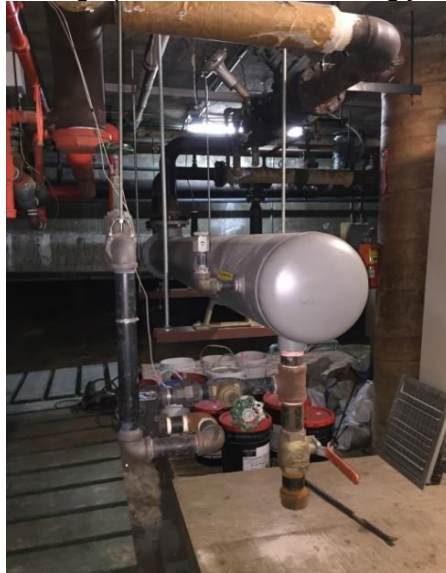
Photograph 2.5.3.1-2: Steam to glycol heat exchanger serving AHU-1
