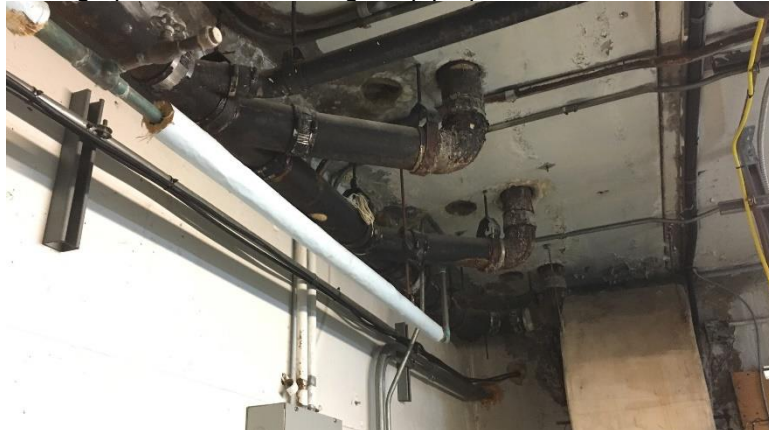
Photograph 3.2.3.1-3: Leakage at pipe penetrations.
