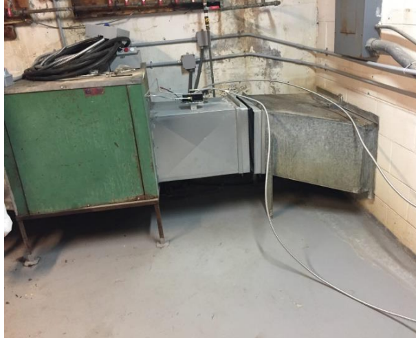
Photograph 2.5.3.3-1: AHU-3 unit supplying combustion air to boilers
