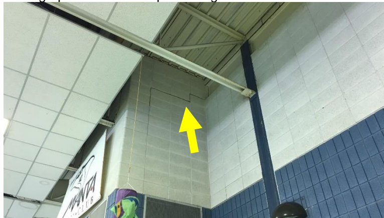
Photograph 3.2.4.2-1: Step cracking in south wall.
