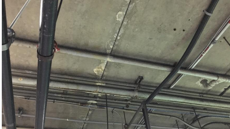
Photograph 3.2.3.1-1: Leakage along main floor hollowcore joints.
