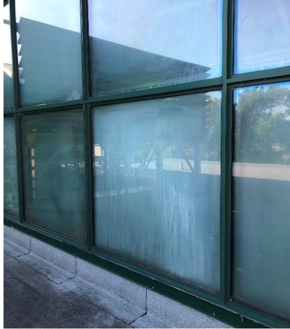
Photograph 3.3.2.1-4: Typical example of a failed sealed glazing unit, exhibiting condensation between the lites.
