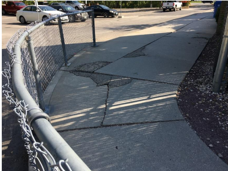
Photograph 3.1.1.1-1: Partial view of sidewalk cracking and movement.
