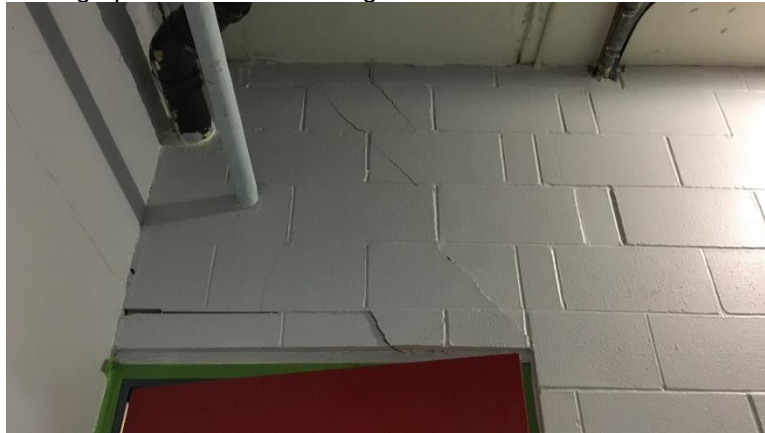
Photograph 3.2.1.2-1: Cracking in CMU wall.
