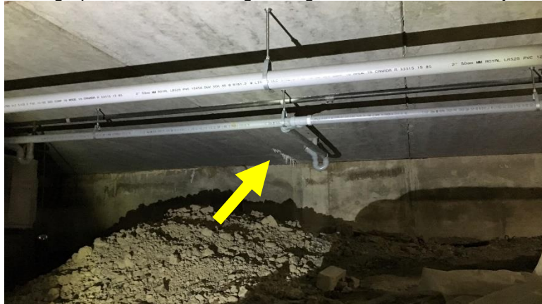
Photograph 3.2.3.1-2: Leakage along main floor hollowcore joints.
