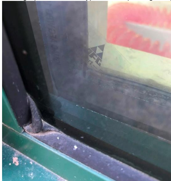
Photograph 3.3.2.1-5: Typical example of glazing sealant displacement.
