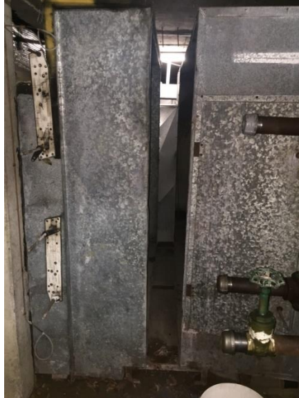
Photograph 2.5.3.1-1: AHU-1 serving pool deck; glycol loop down for repairs
