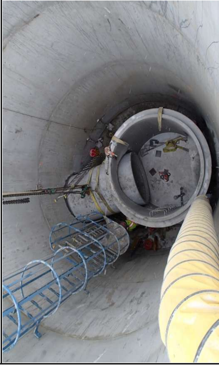
Photo 3 (Looking E): Lowering MH32 chamber and 1350 mm pipe
