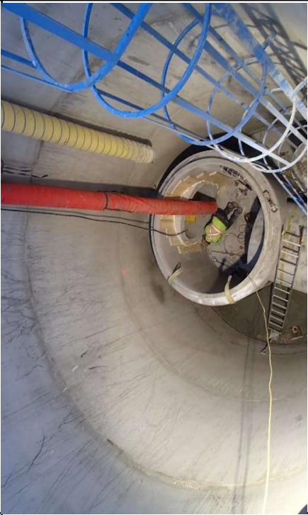
Photo 4 (Looking W): Preparing MH32 chamber connection for a concrete pour tomorrow.
