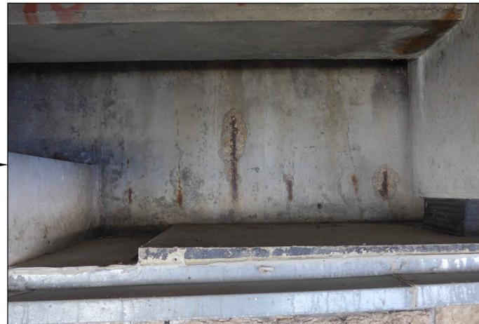
TYPICAL EXPOSED REINFORCEMENT
