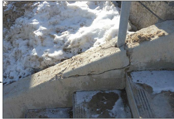
TYPICAL DELAMINATED AND SPALLED CONCRETE AROUND HANDRAIL POST AT NORTH PLAZA
