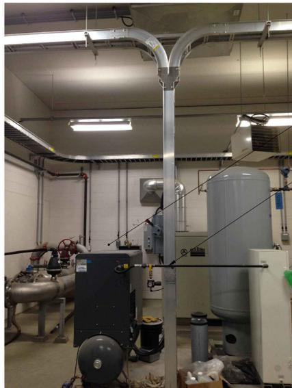
NEW 50Ø INSTRUMENT AIR LINE TO EXIT BUILDING ALONG THE NORTH WALL. SEE DETAIL 3.
