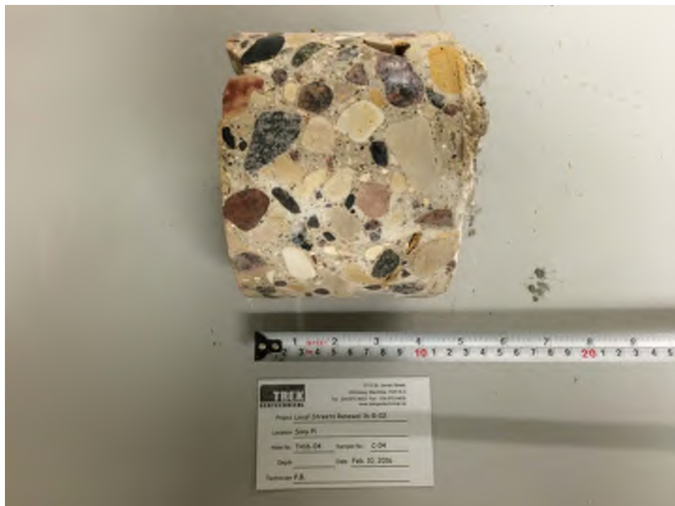
Photo 4: Pavement Core Sample at Test Hole TH16-04
