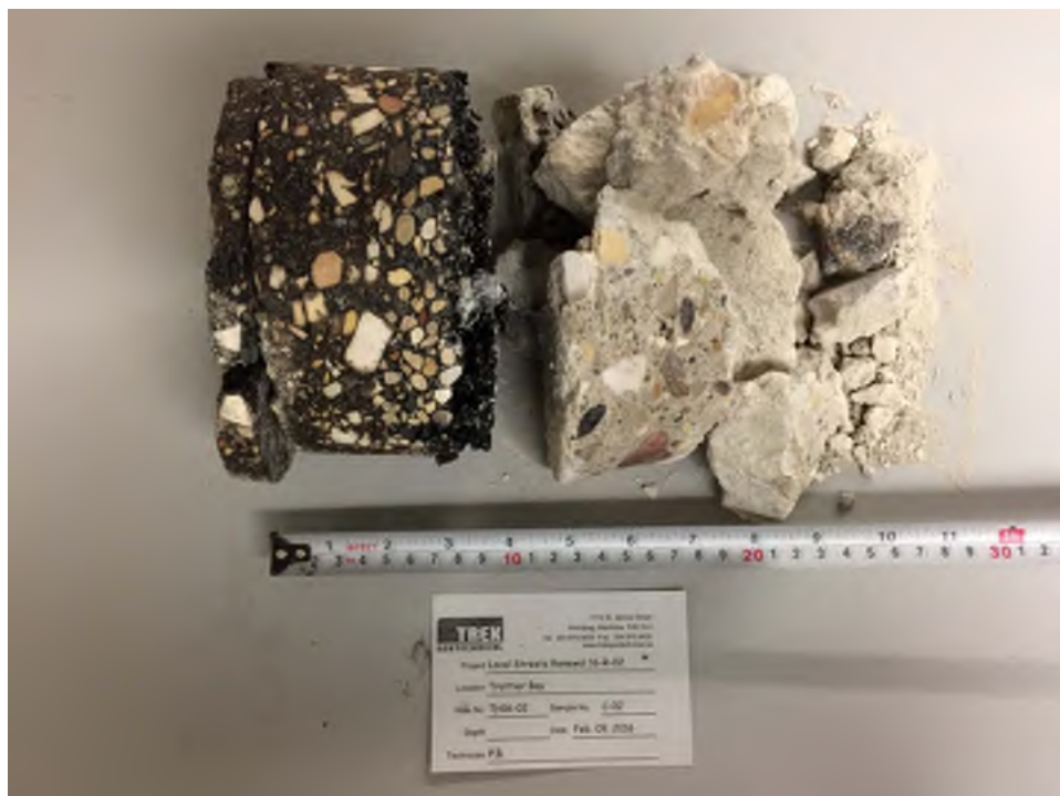
Photo 2: Pavement Core Sample at Test Hole TH16-02
