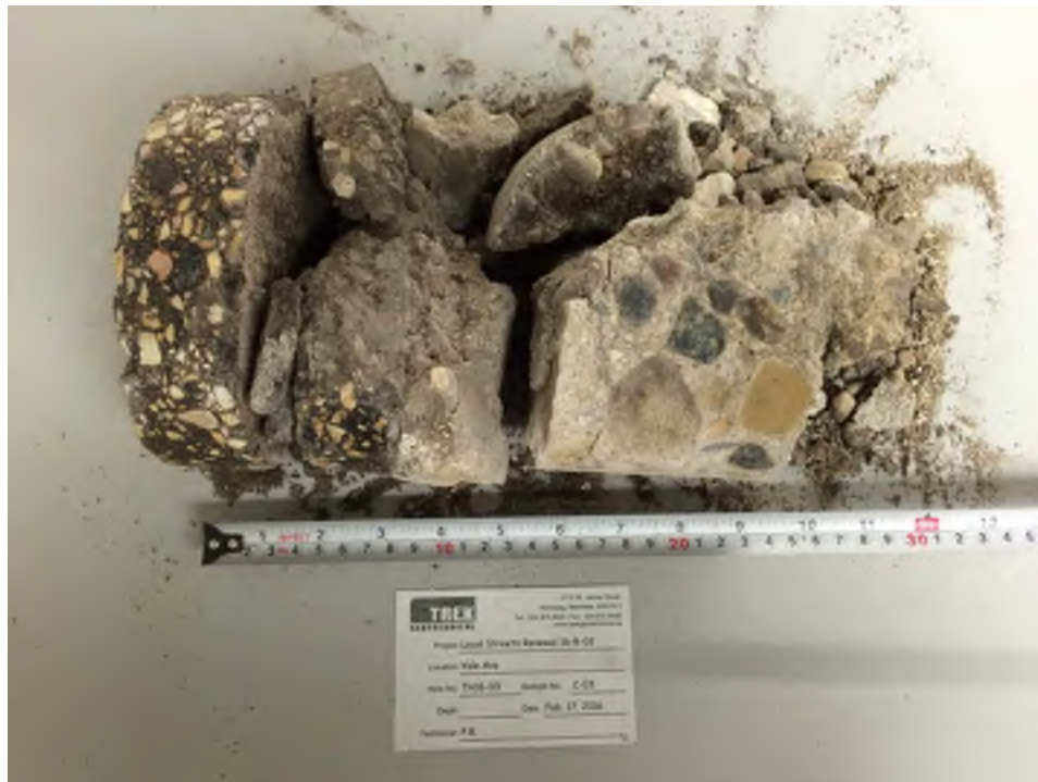
Photo 3: Pavement Core Sample at Test Hole TH16-03
