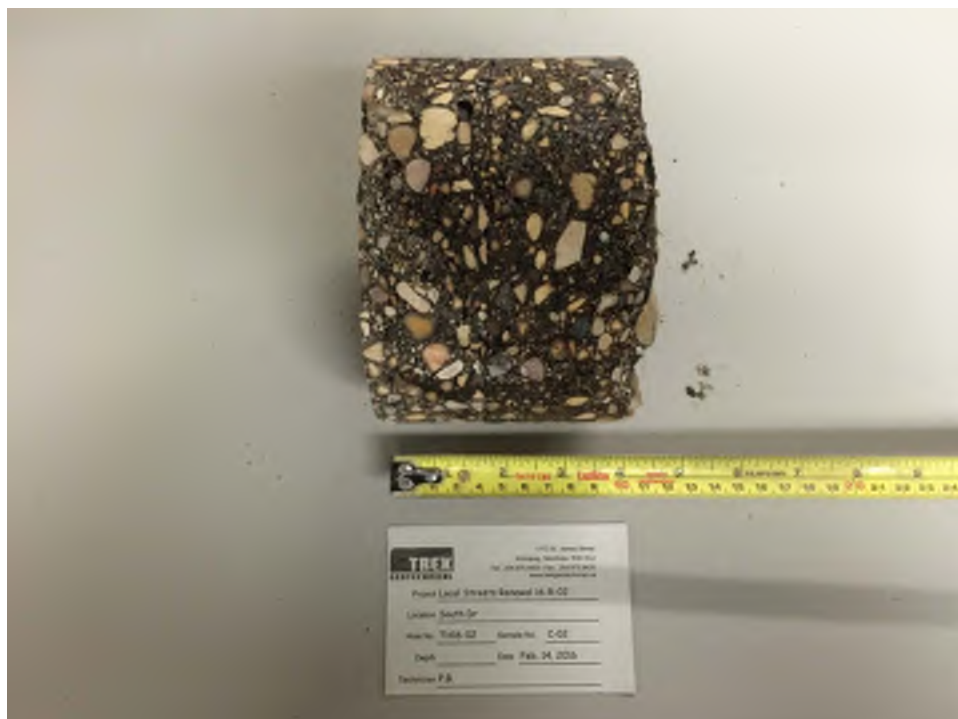
Photo 2: Pavement Core Sample at Test Hole TH16-02
