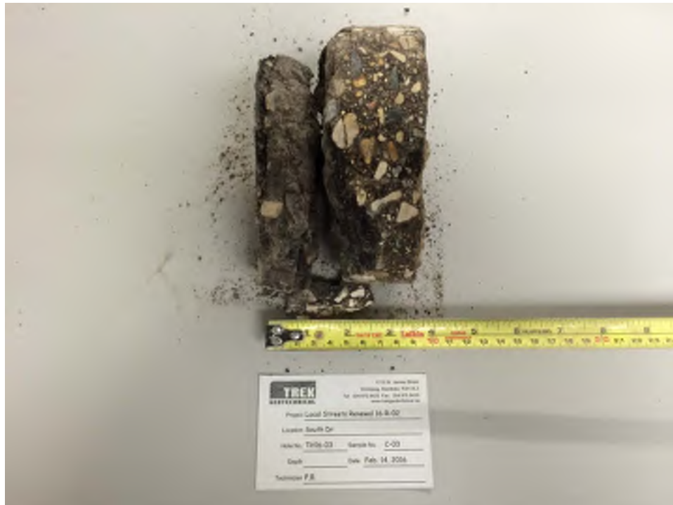
Photo 3: Pavement Core Sample at Test Hole TH16-03
