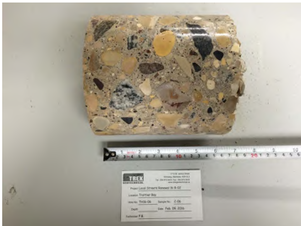
Photo 6: Pavement Core Sample at Test Hole TH16-06
