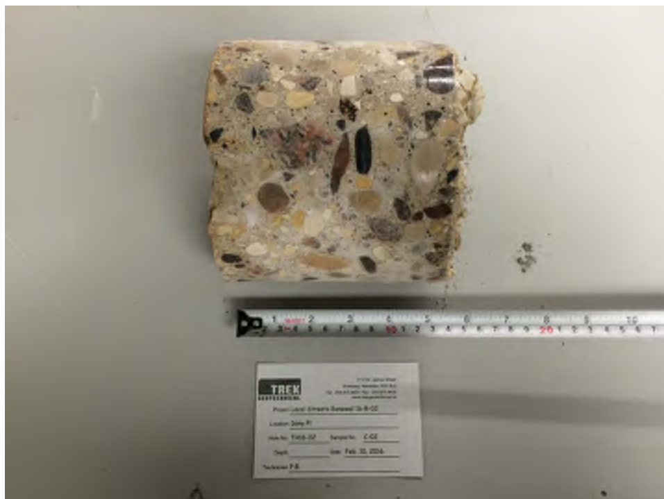
Photo 2: Pavement Core Sample at Test Hole TH16-02
