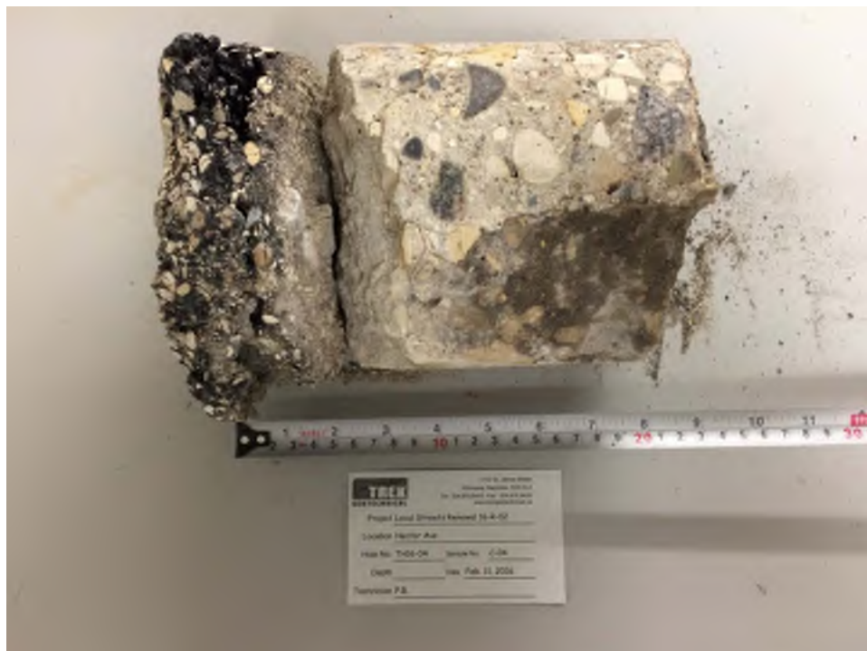
Photo 4: Pavement Core Sample at Test Hole TH16-04
