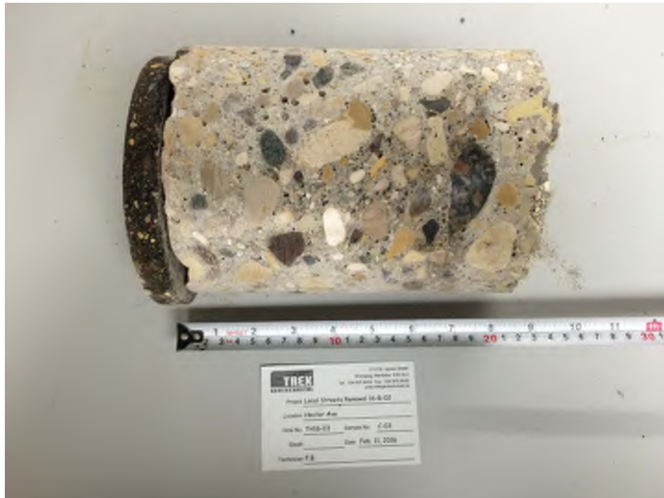
Photo 3: Pavement Core Sample at Test Hole TH16-03
