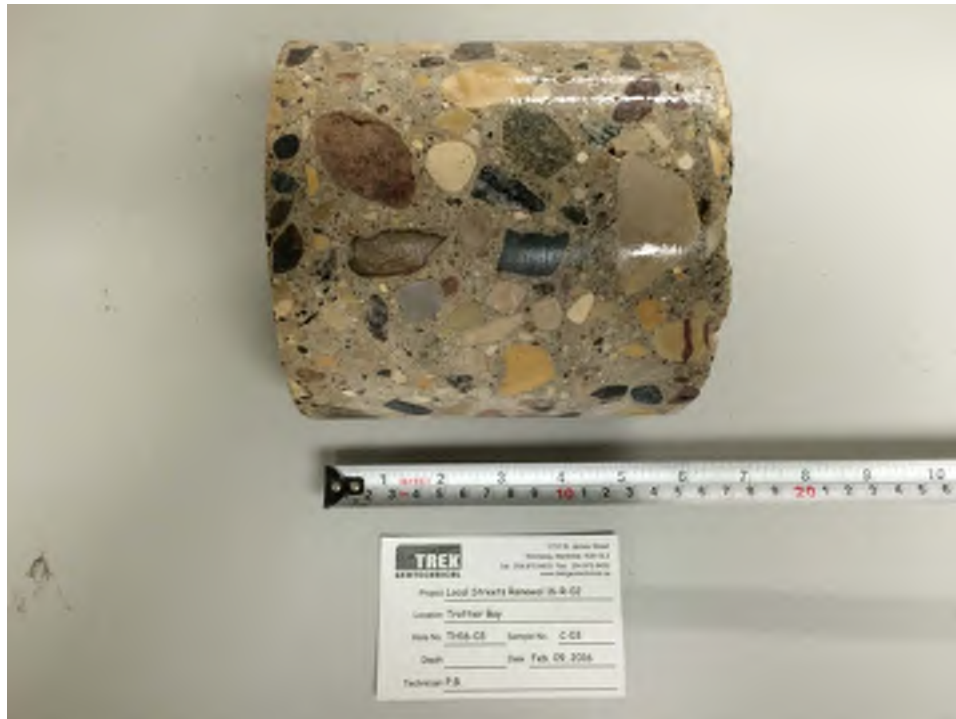
Photo 3: Pavement Core Sample at Test Hole TH16-03
