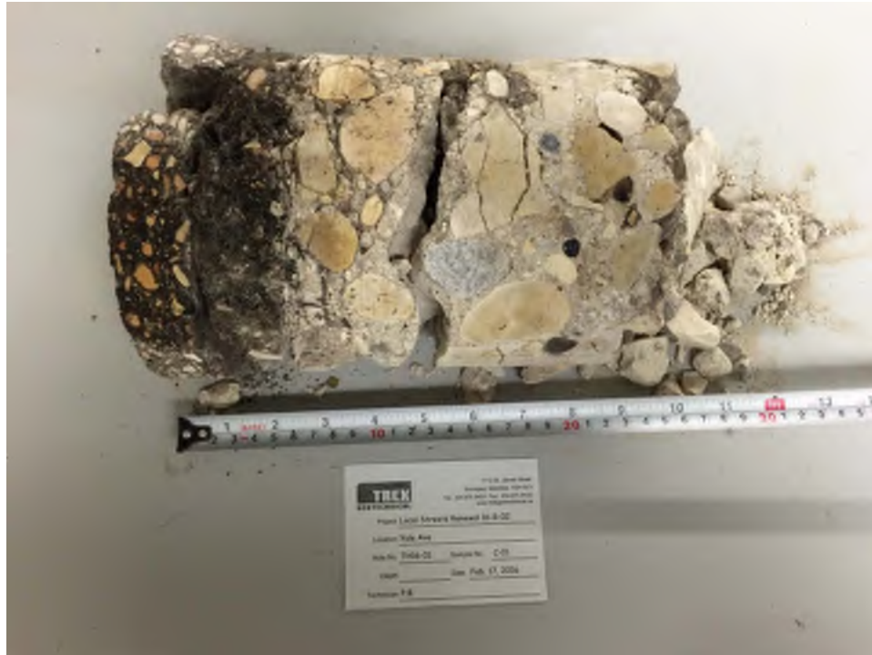
Photo 1: Pavement Core Sample at Test Hole TH16-01
