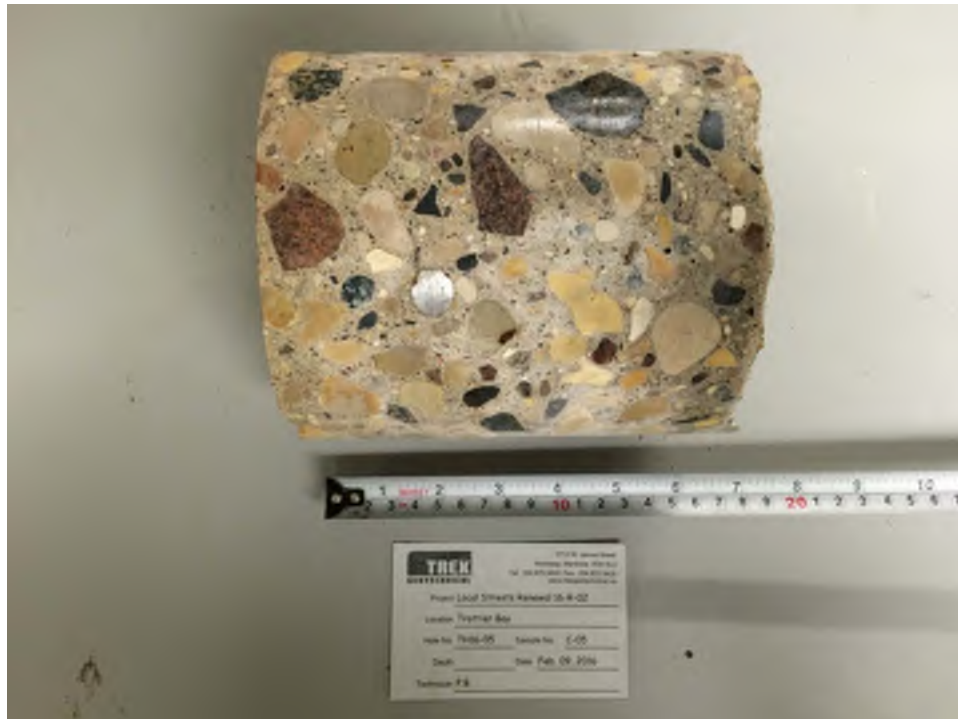
Photo 5: Pavement Core Sample at Test Hole TH16-05
