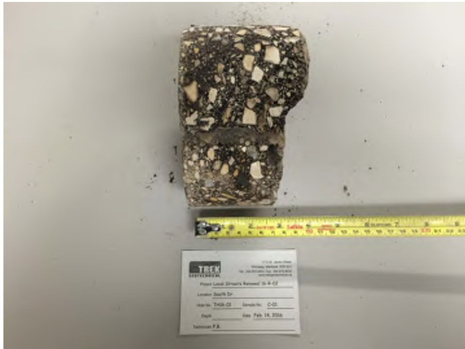
Photo 1: Pavement Core Sample at Test Hole TH16-01
