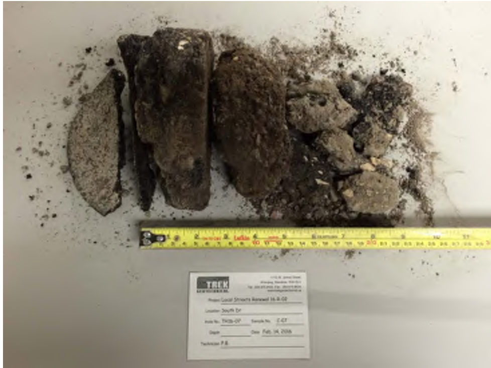
Photo 7: Pavement Core Sample at Test Hole TH16-07
