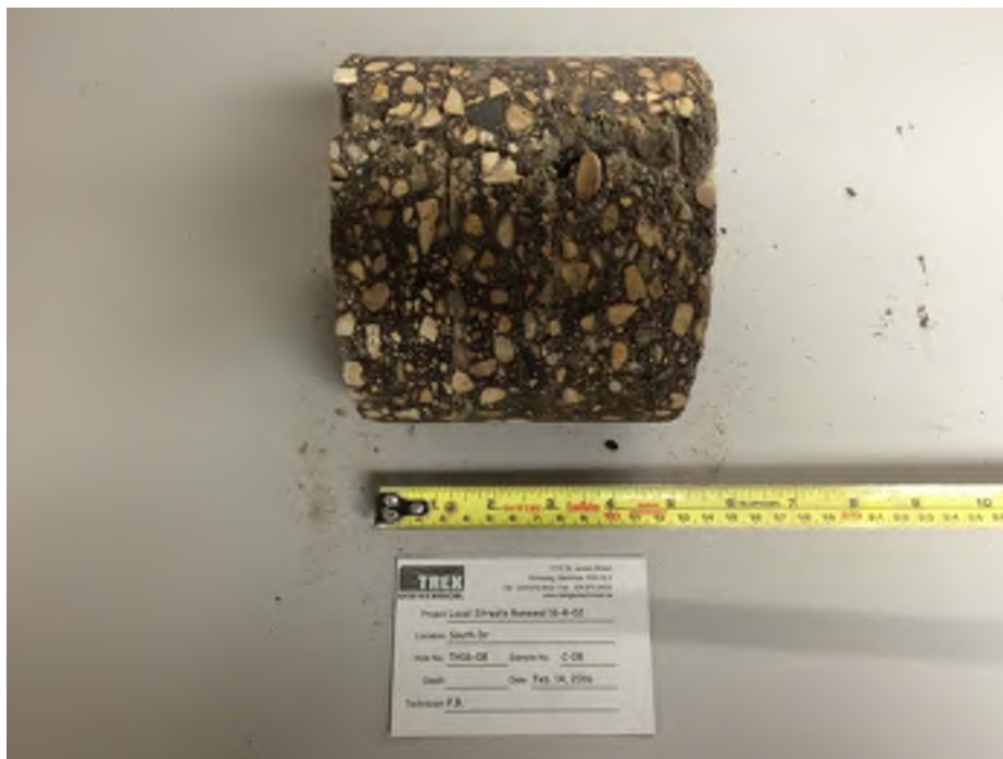
Photo 8: Pavement Core Sample at Test Hole TH16-08
