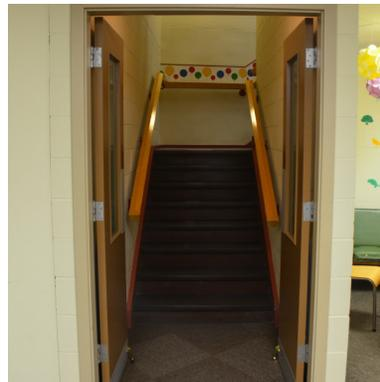
Non-fire rated doors into stairwell at basement level
