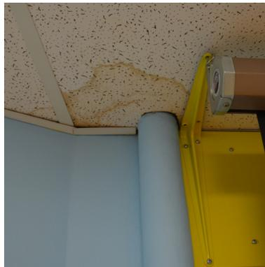
Water staining on acoustic ceiling
