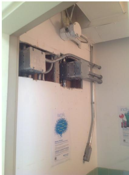
Figure 1: Junction Boxes & Extensions on Rear of Panelboards A & B
