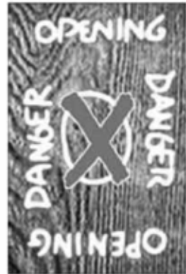
Examples of markings on a plywood cover.
