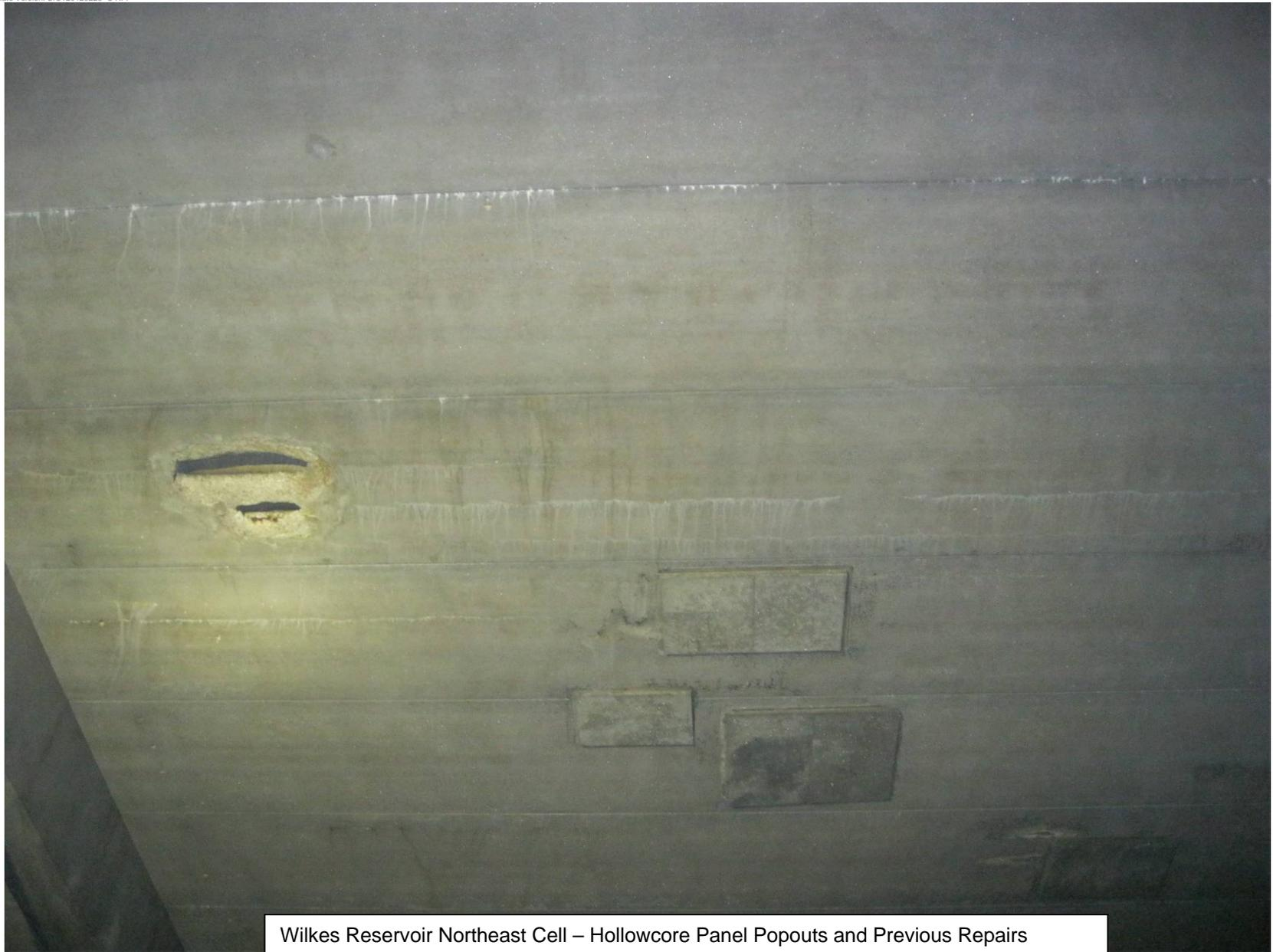
Wilkes Reservoir Northeast Cell – Hollowcore Panel Popouts and Previous Repairs
