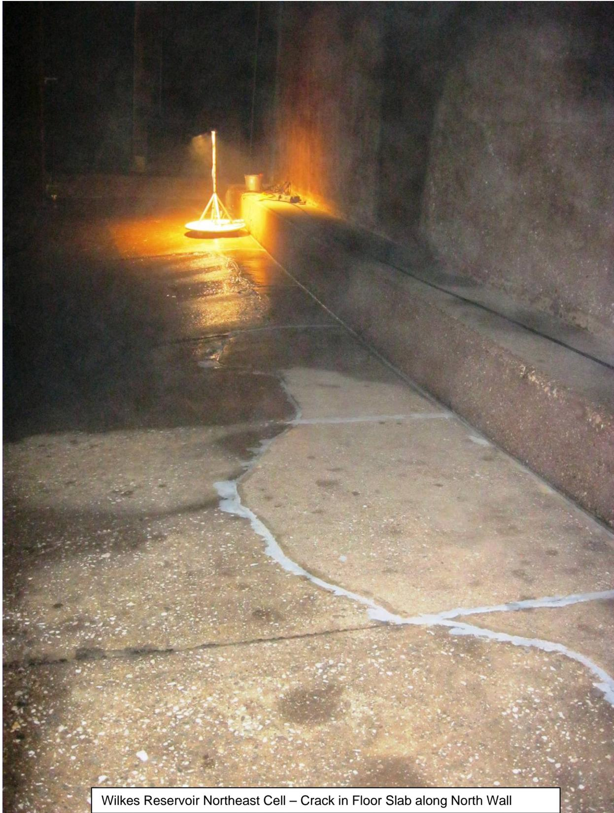
Wilkes Reservoir Northeast Cell – Crack in Floor Slab along North Wall
