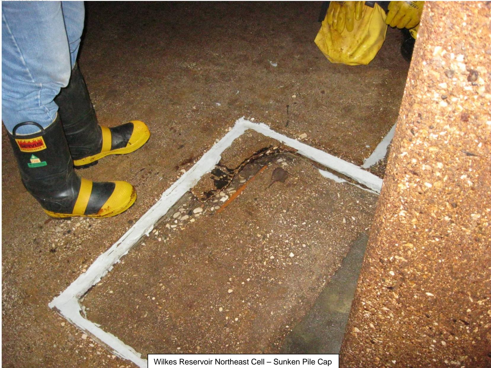
Wilkes Reservoir Northeast Cell – Sunken Pile Cap
