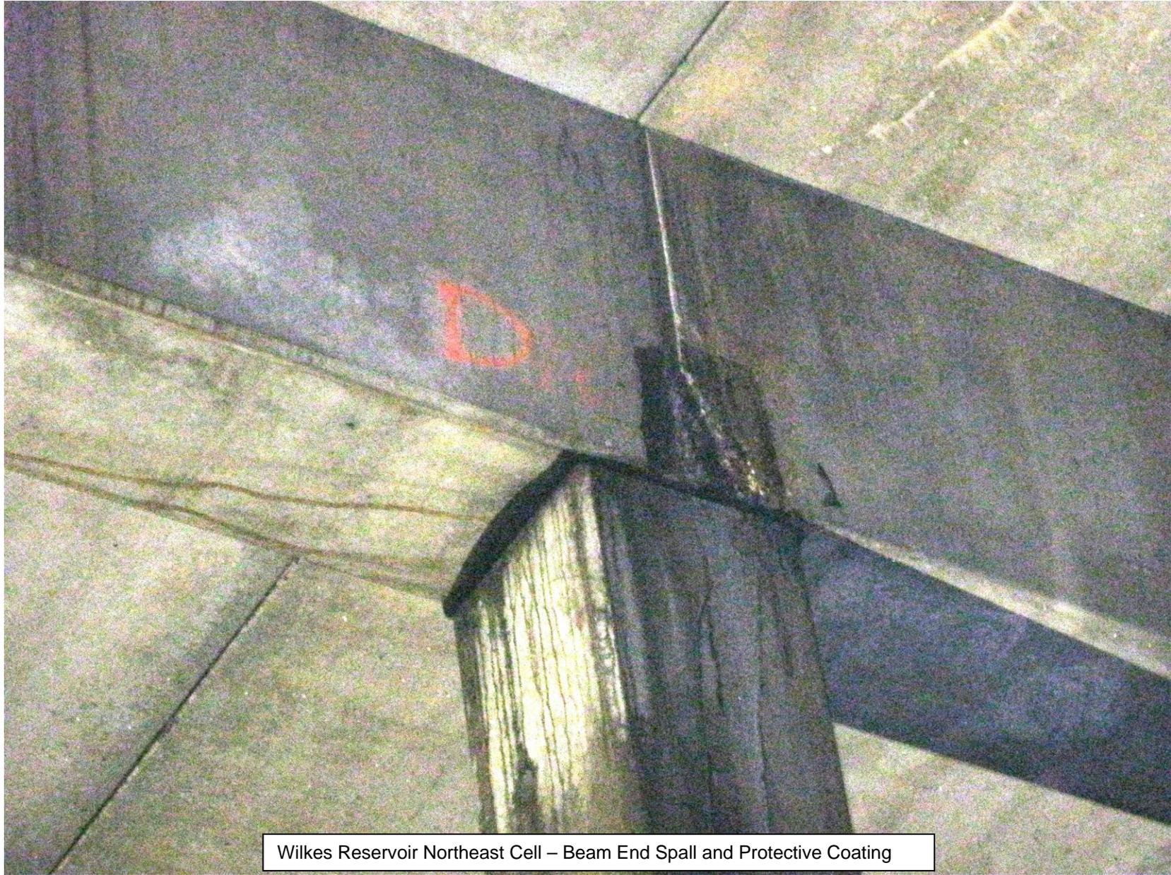
Wilkes Reservoir Northeast Cell – Beam End Spall and Protective Coating
