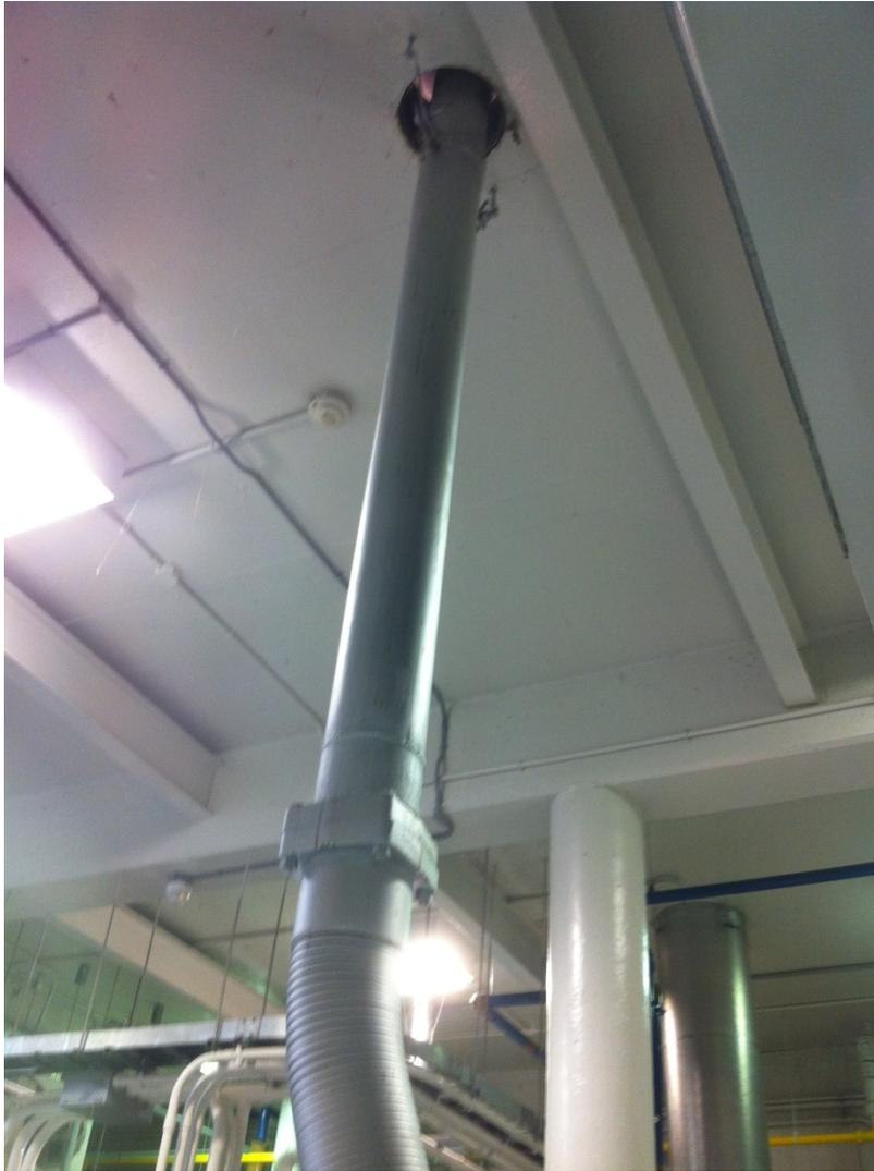
Photo A-3: Low Lift Pump Exhaust Vertical Section
