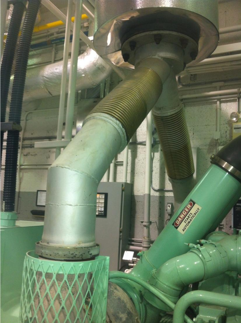
Photo A-2: Emergency Gen Set Exhaust Flexible Y Section
