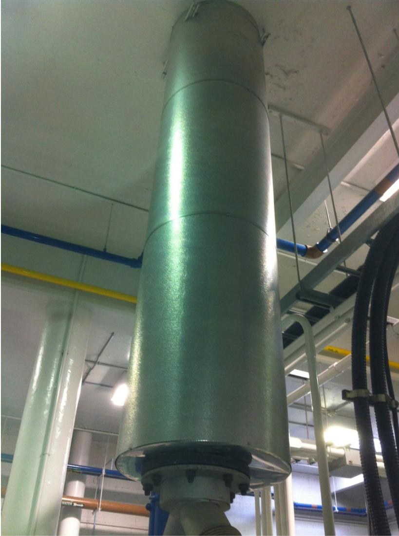
Photo A-1: Emergency Generator Exhaust Vertical Section
