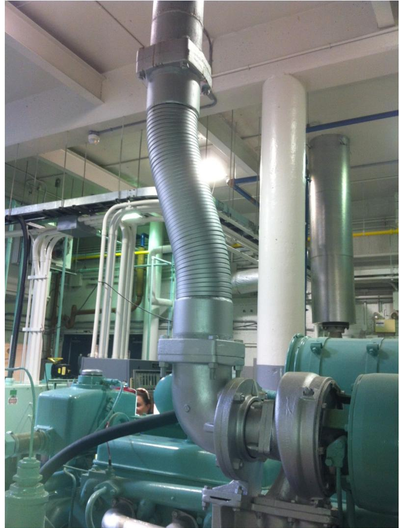
Photo A-4: Low Lift Pump Exhaust Flexible Section
