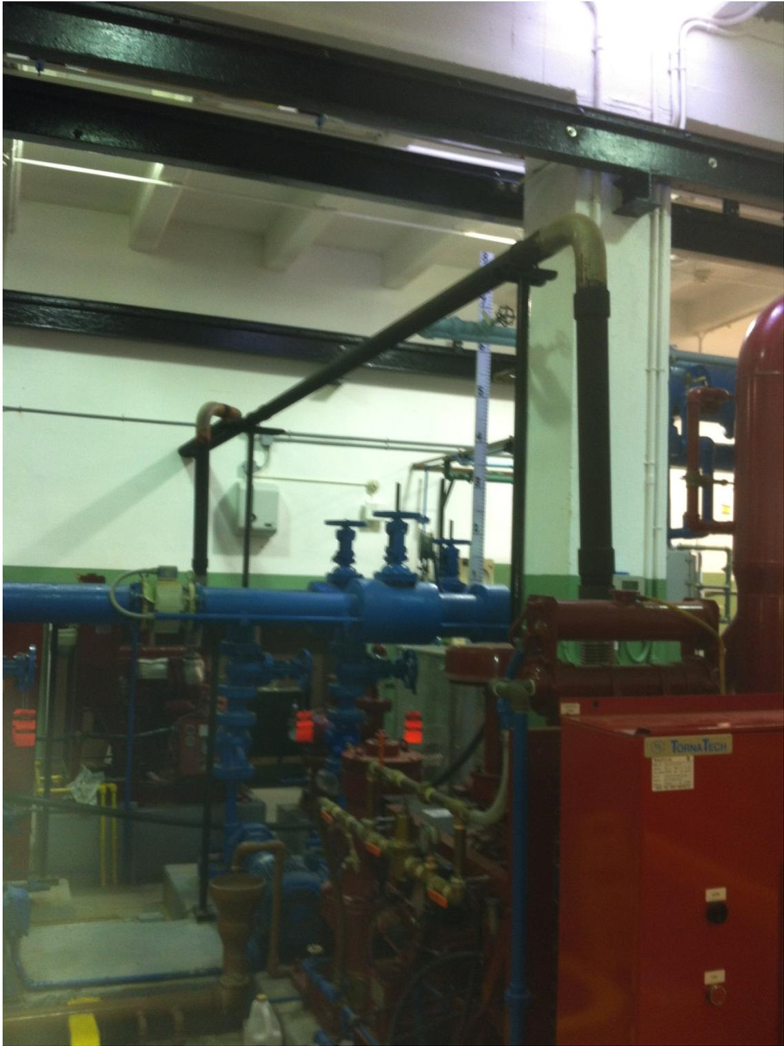
Photo A-8: Fire Pump #1 Exhaust Pipe Run
