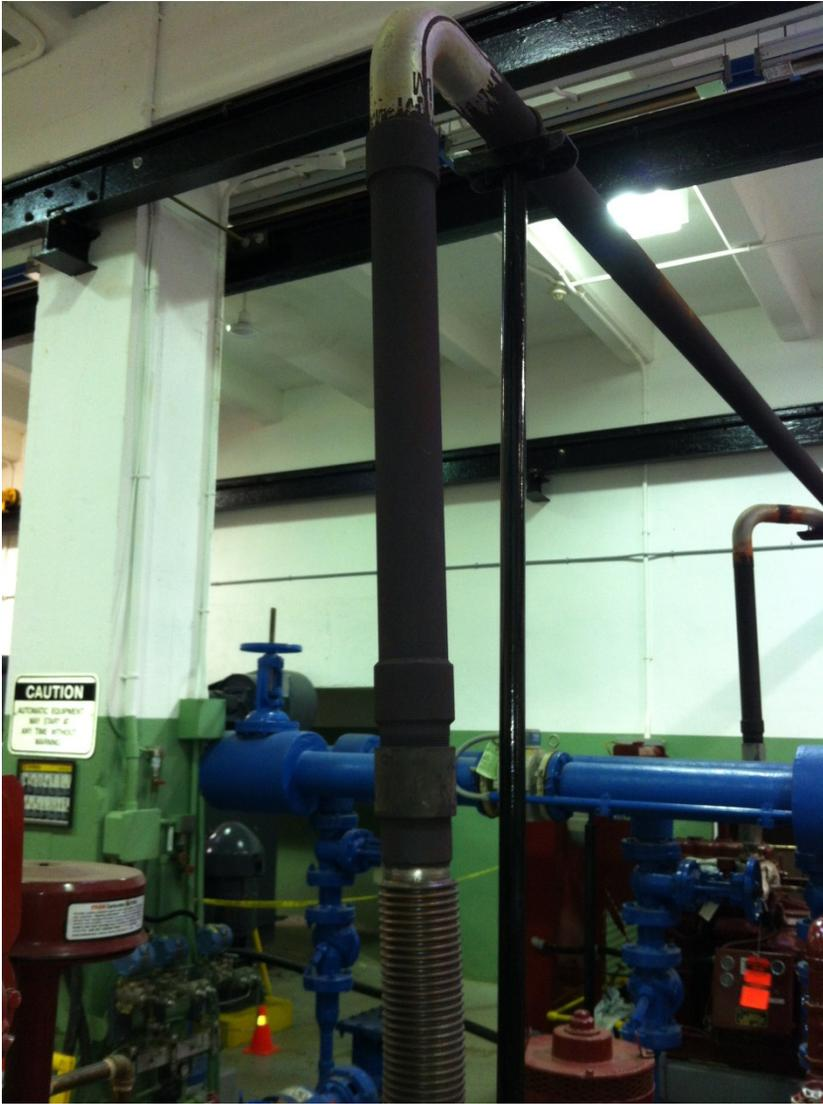
Photo A-6: Fire Pump #1 Vertical Exhaust and Bend
