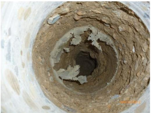
Figure 4 – Poly vapour barrier present 100 mm below underside of concrete
