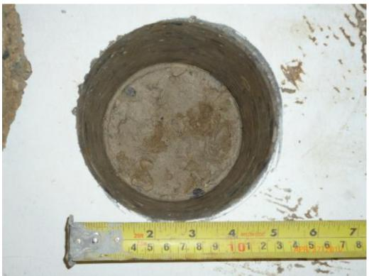
Figure 2 - Granular base course at underside of concrete slab
