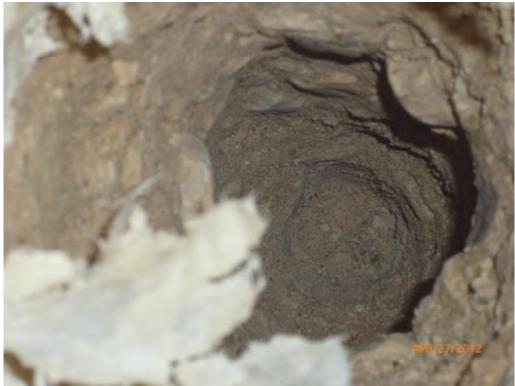
Figure 5 – Granular base at a depth of 0.75 m below top of concrete slab
