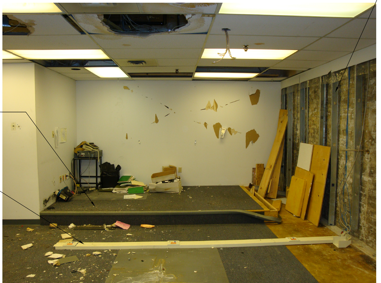
3 EXISTING ROOM A03 NTS
