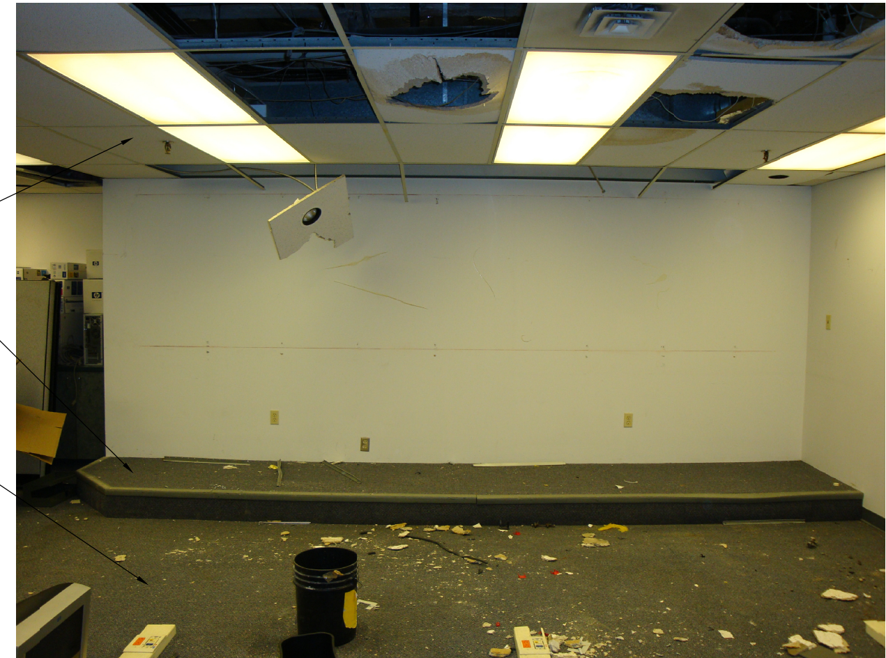
2 EXISTING ROOM A03 NTS
