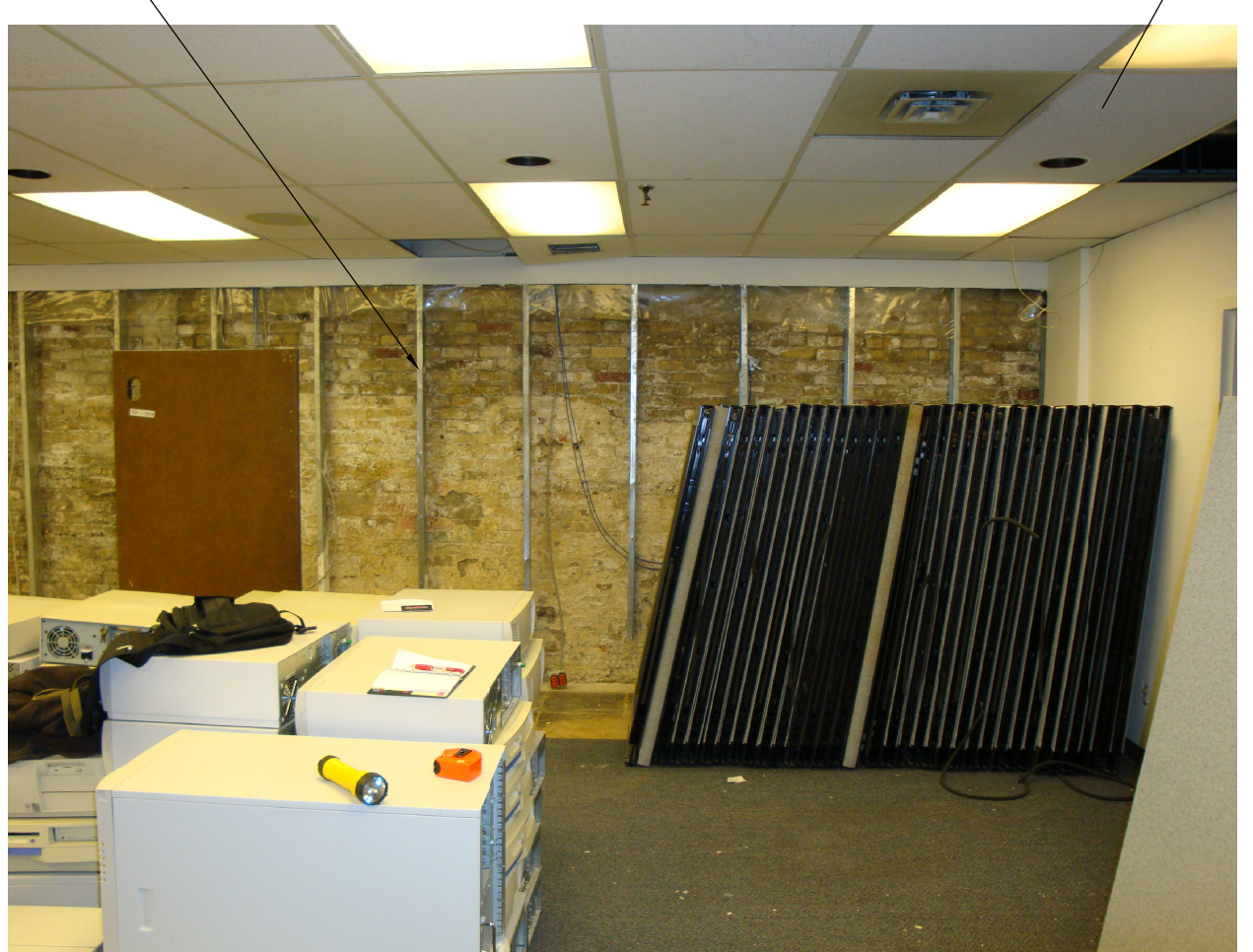
5 EXISTING ROOM A03 NTS
