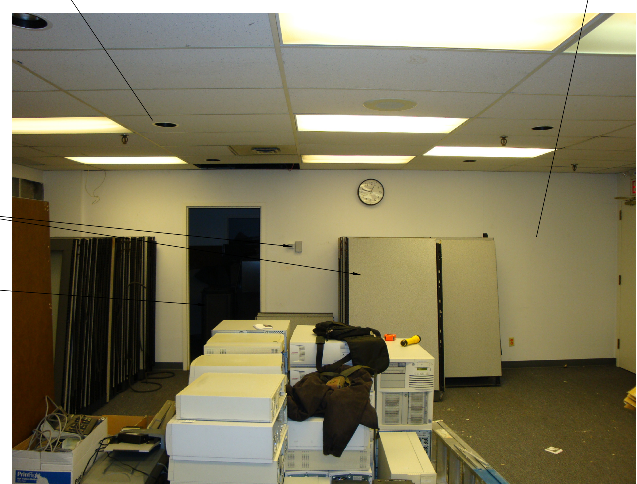
6 EXISTING ROOM A03 NTS
