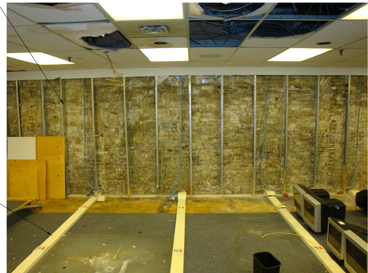
4 EXISTING ROOM A03 NTS
