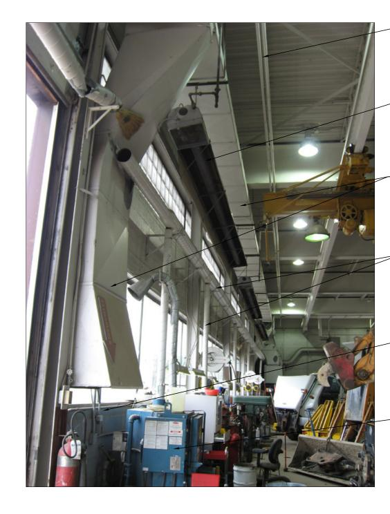
REMOVE NATURAL GAS PIPING (+/- 150'-0", APPROX. 20'-0" AFF) FROM NORTH WALL OF SHOP AND STORE FOR REINSTALLATION AFTER O/H DOOR AND SLAB REPLACEMENT, DISCONNECT CONNECTIONS AND ENSURE SUPPLY IS CORRECTLY CUT-OFF, RE-CONNECT @ TIME OF REINSTALLATION.
