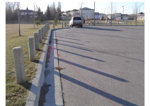
PARKING LOT EDGE. REMOVE BOLLARDS TO GAIN ACCESS TO THE SITE. REPAIR ALL DAMAGE.
